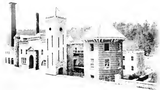
ONE OF THE FACADES AT THE GREAT OLD TAYLOR PLANT
