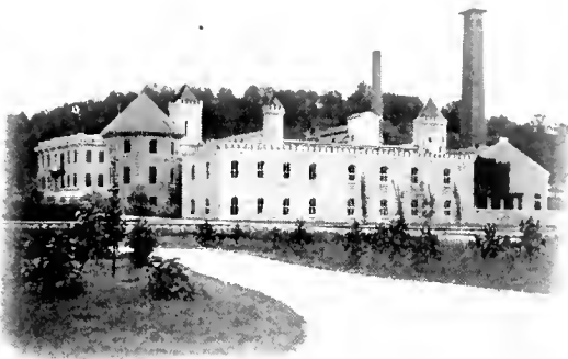
VIEW OF THE FERMENTORY ROOM OF THE OLD TAYLOR DISTILLERY
