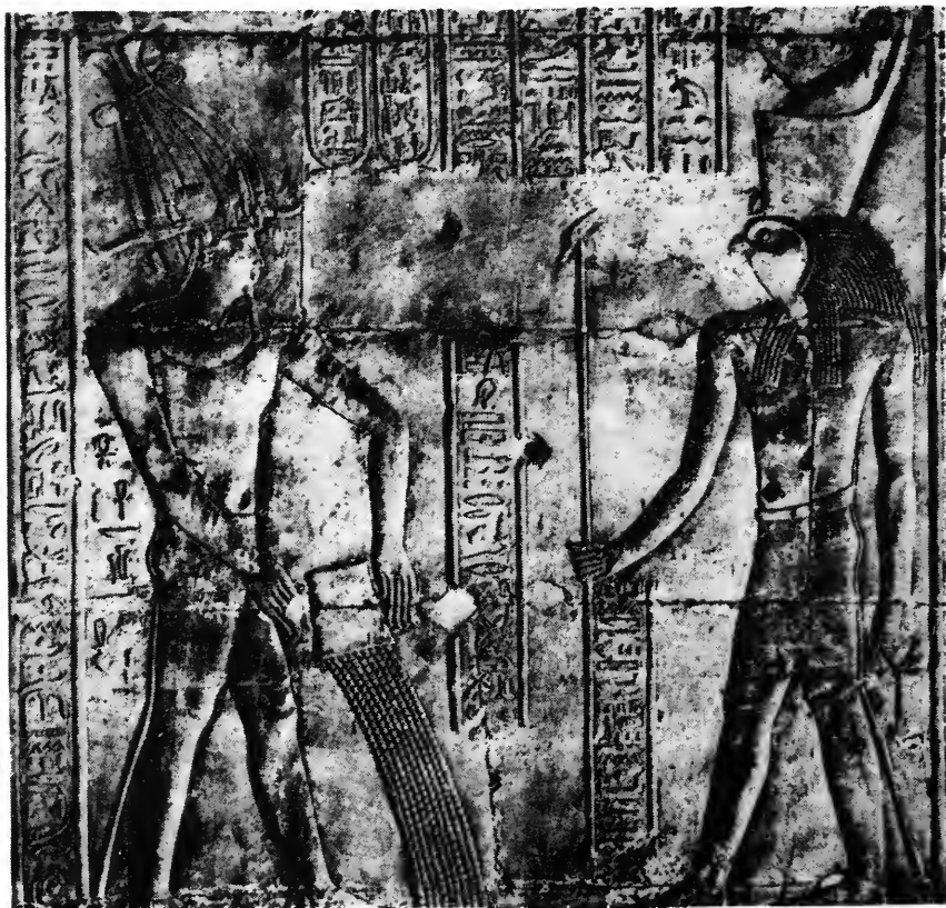
Pouring sand in the foundation trench (Temple of Edfu)
