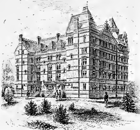
THE NEW DORMITORY, WITHERSPOON HALL.
