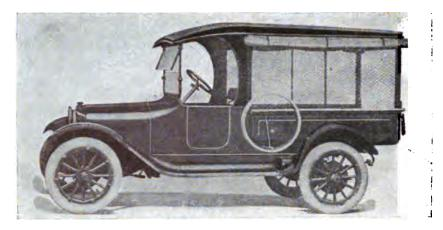
FIG. 561. In this car a passenger chassis is used; and front end, consisting of cowl, windshield and front door are worked into the commercial body construction
