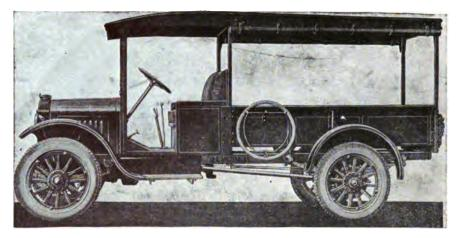
F1G. 566. A speed wagon type, with removable top and posts, easily convertible into an open body
