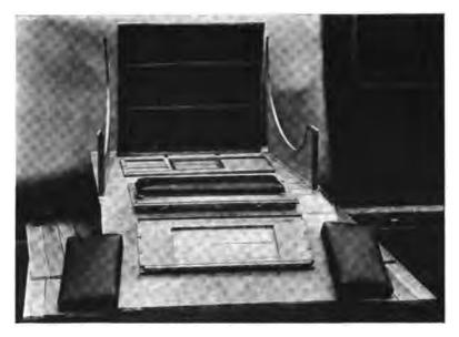
Fic. 614 Cab with all the main parts dismantied ready for crating. The knock-down feature is a very important one, as it reduces freight rates and is more convenient all around.
