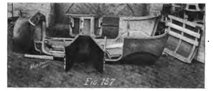
Side view of body partially disassembled for shipping purposes
