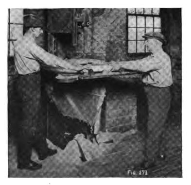
One of the processes of door-making. Sawing the door out of the frame
