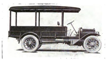
FIG. 556. Same type of express body as shown in Fig. 555, but with canopy top
