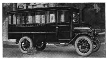
Fic. 595 Typical bus construction for short trips. (Vehisote panels used).
