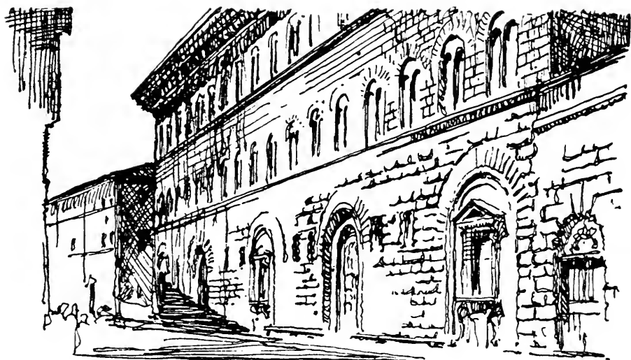
FIG. 44.—Riccardi Palace, Florence. Note the contrast in the surface treatment of the masonry in ground and upper stories.
