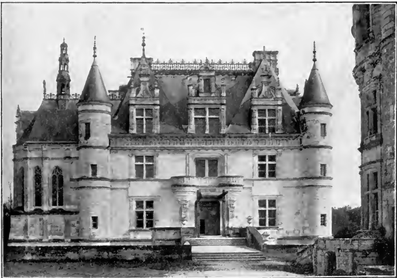
52. Chenonceaux. A fine example of both double and triple subordinate masses, the two turrets and the three dormers.
