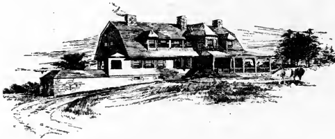
265. House at Little Harbor, N. H. The dormers are arranged as an unsymmetrical triple group.
