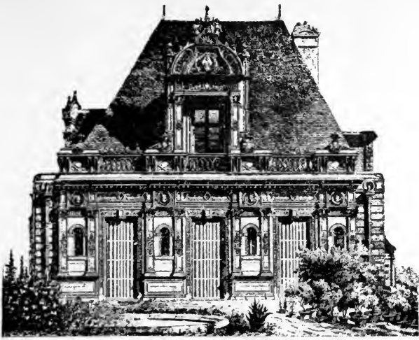
12. A Single Mass. Although sub-divided into horizontal parts by the line of the cornice, it is single in vertical division; that is, it has no other mass standing beside it. The oneness is accentuated, too, by the one big dormer on the roof.
