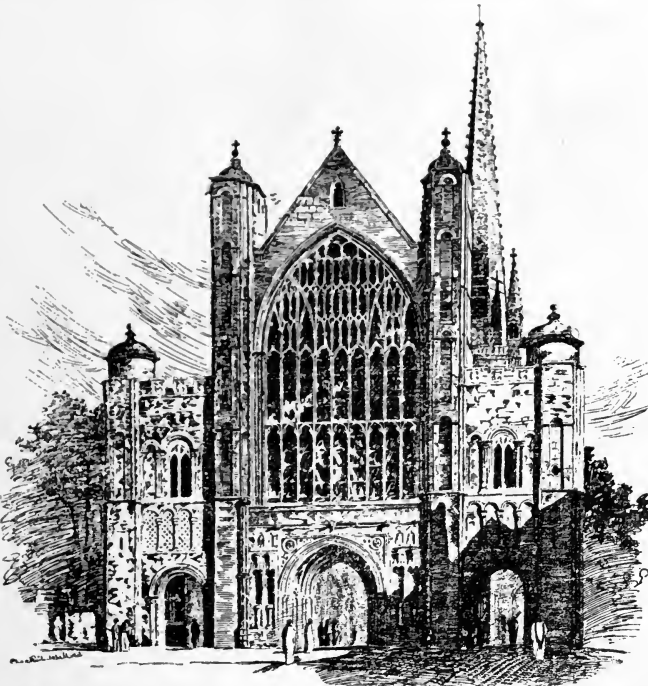
97. Norwich Cathedral, East Front. The central gable is the mass; the square-topped aisles are the appendages.
