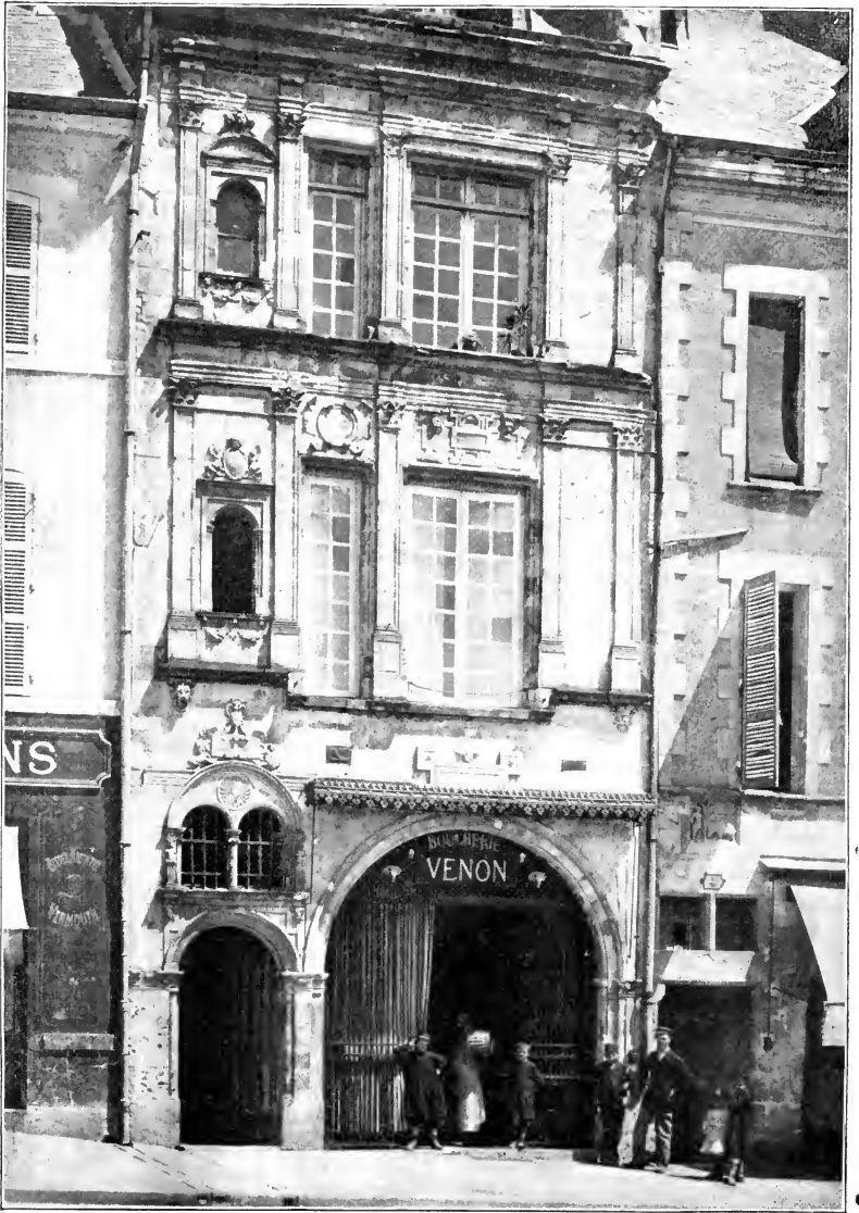
124. House, Place des Halles, Orleans, France. Not only the arches of the first story but the windows above are double unequal groups. It would improve the composition to omit the anomalous niches in the upper stories.
