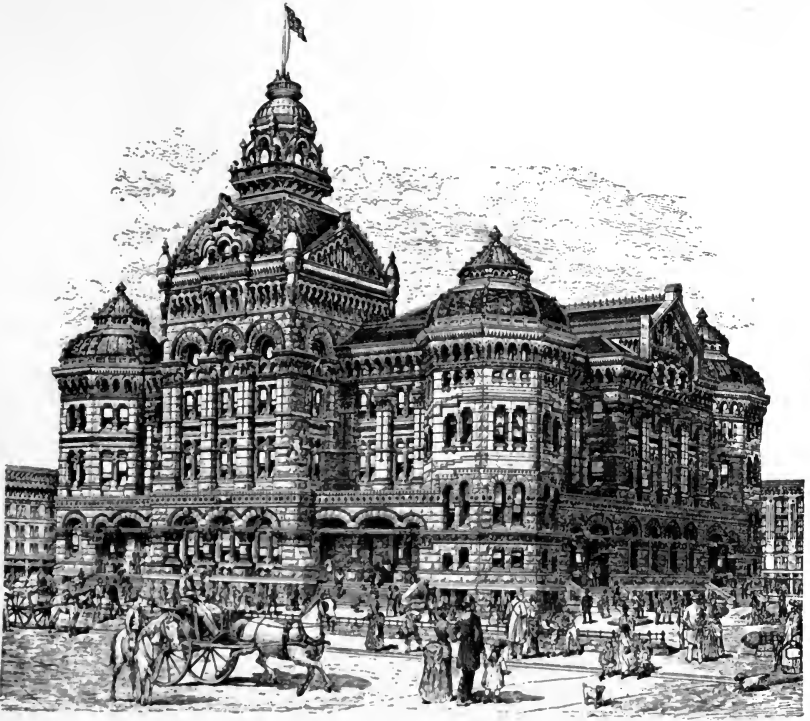
293. Another example for critical analysis. Masses not properly subordinated.
