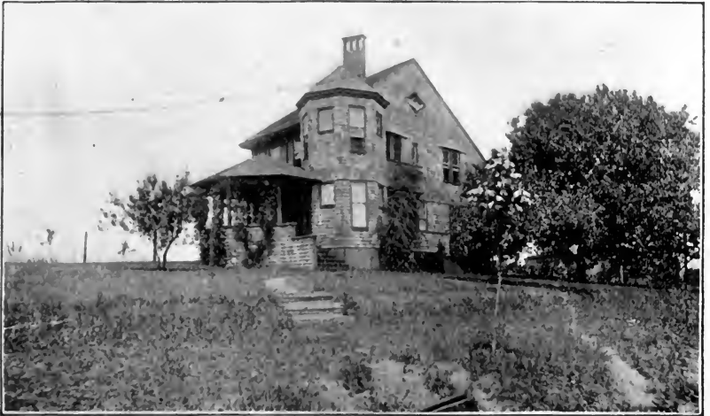
228. Small country house, a single mass, with one subordinate mass and one appendage.
