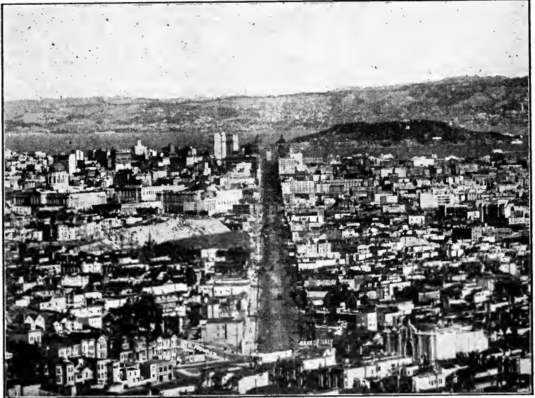
FIG. 43.—Market Street, San Francisco. This street is 120 feet wide between property lines, and 80 feet between curb lines. It is unique among larger city thoroughfares in that for its entire length through the central district it is equipped with four street-car tracks. At the end of Market Street is what is said to be the largest ferry terminal in the world. ( Gabriel Moulin, photographer, San Francisco. Courtesy of San Francisco Chamber of Commerce. )
