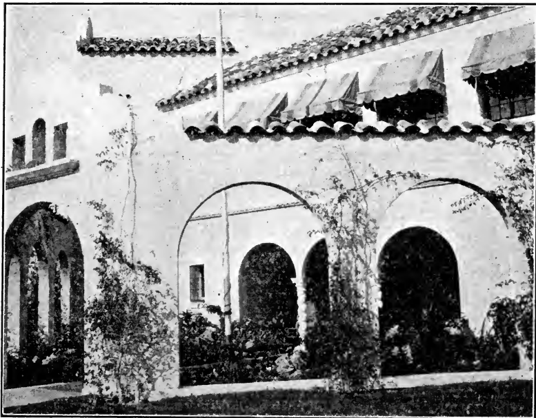
FIG. 128.—Fire-engine house, Miami, Fla. The opportunity to make public buildings a credit to the community is not always so nicely realized as in the case of this fire-engine house. ( Photograph by the Author. )
