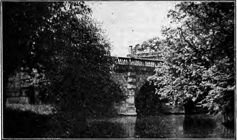
FIG. 139.—Magdalen Bridge at Oxford, England.
