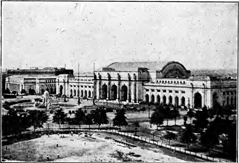
FIG. 138.—The plaza and Union Station, Washington, D. C.
