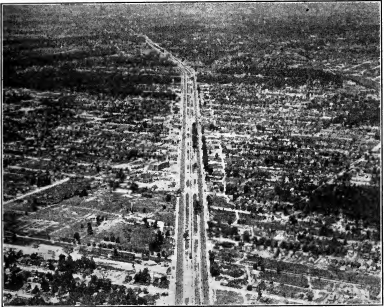
FIG. 41.—A "superhighway" of Detroit as seen from the air. The air-view comparison helps to visualize the immensity of the new superstreets of Detroit. These 204-foot ways when completed will have a central space of 84 feet for the exclusive use of rapid transit lines and planting, a 20-foot roadway for local traffic on each side, and a 15-foot sidewalk on each side. Wheel traffic may cross under at half-mile intersections, and pedestrians may pass over or under here and there as conditions warrant. ( Kalec and Forster, photographers. )
