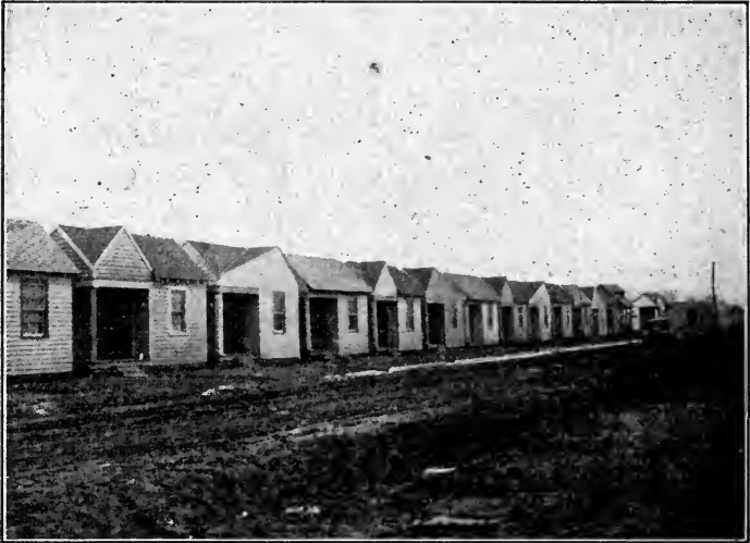
FIG. 103.—A row of shacks intended for homes. Freedom to build atrocities like these in a city is a reflection upon the good sense of the city.
