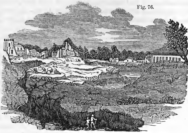
Deep fissure, near Pollstena, caused by the earthquake of 1783.
