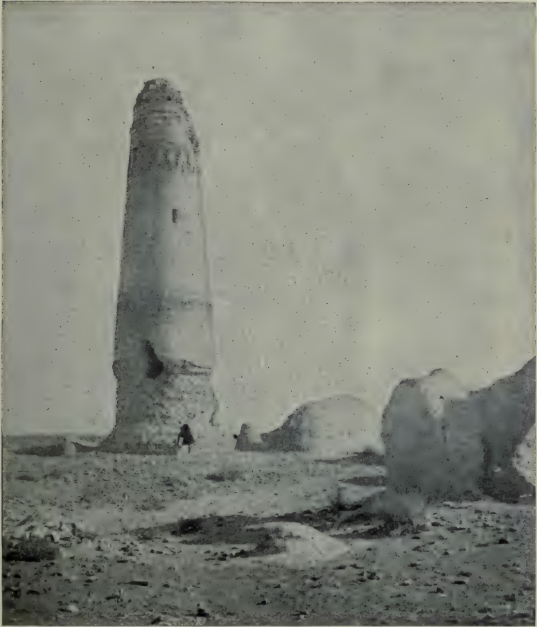
FIG. 118.—A Ruined Tower in Eastern Persia.
