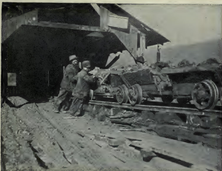
FIG. 62.—Shoving Cars in a Coal Mine.
