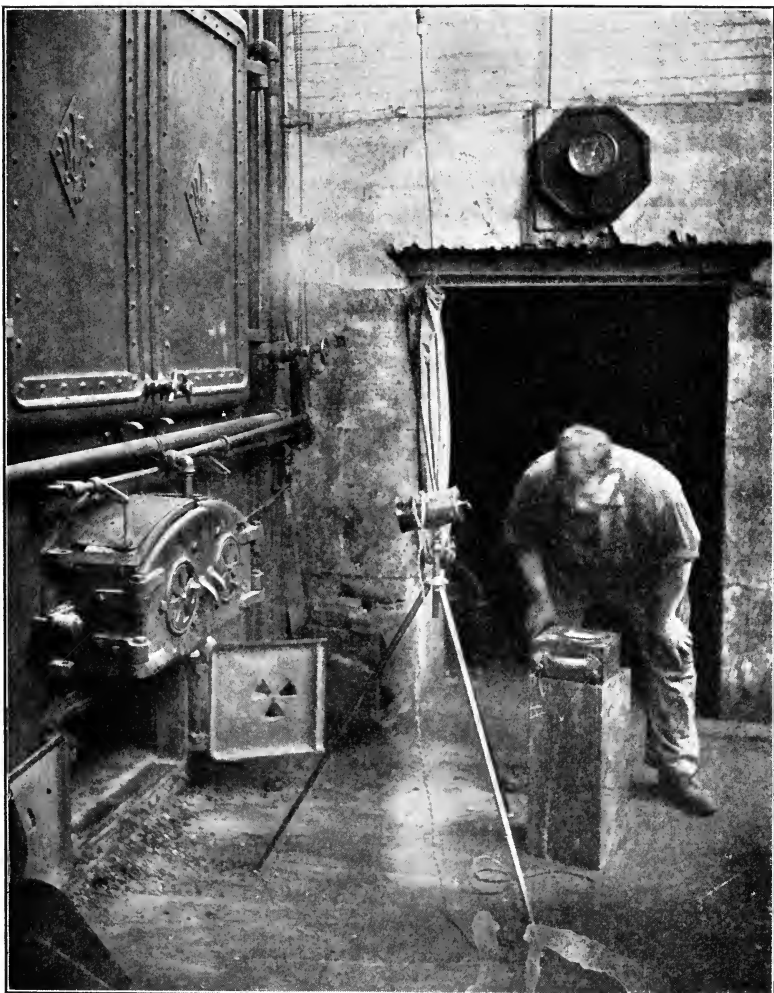
FIG. 61. — Fery pyrometer set up for an observation.
