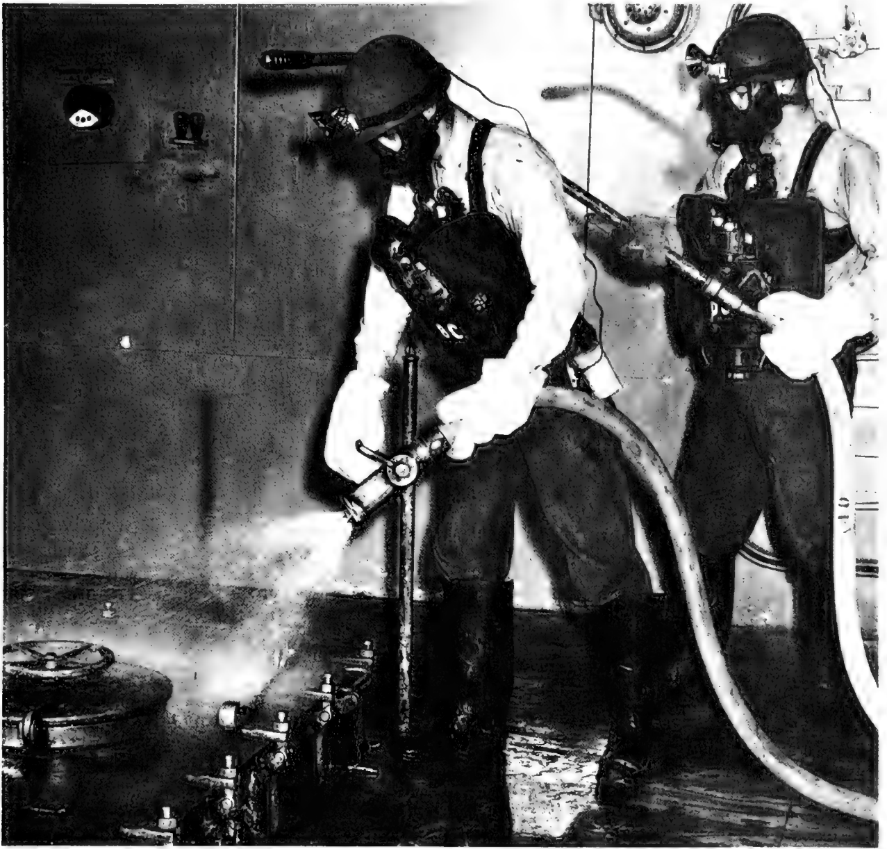
Figure 4-3.—Members of firefighting party cooling hatch.
