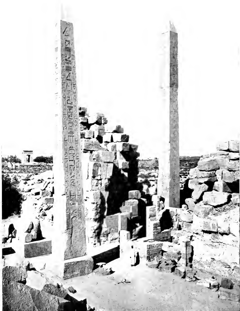
FIG. 1.—OBELISKS OF TUTHMÔSIS I ( left ) AND HATSHEPSOWET ( right ) AT KARNAK. ( The nearer obelisk leans to the left owing to soil-subsidence. )
