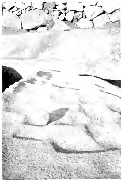
FIG. 5.—HAMMER-DRESSING ON PYRAMIDION OF ASWAN OBELISK. (Page 36)
