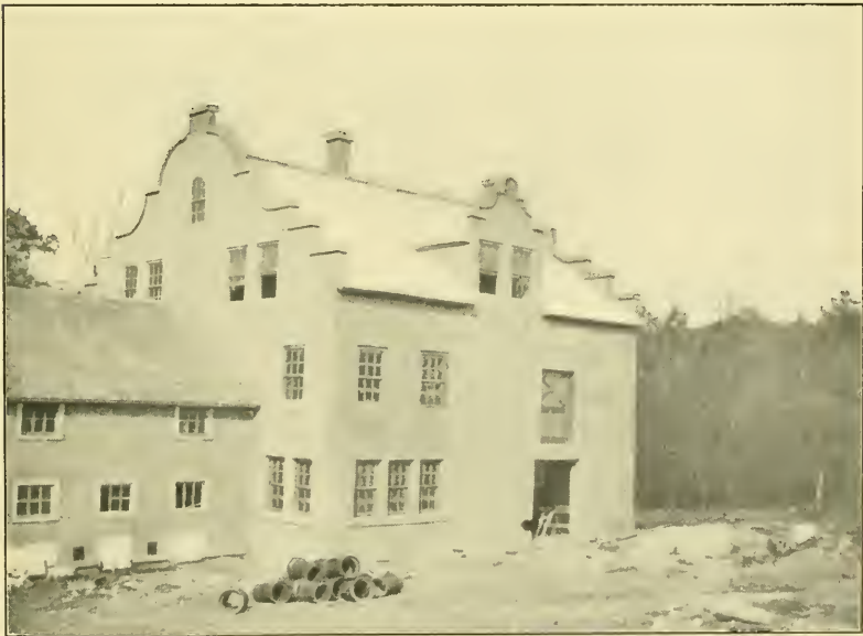
FIG. 2.—REINFORCED CONCRETE BUILDING.
