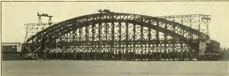
FIG. 3.—ERECTION OF THE DÜSSELDORF BRIDGE.
