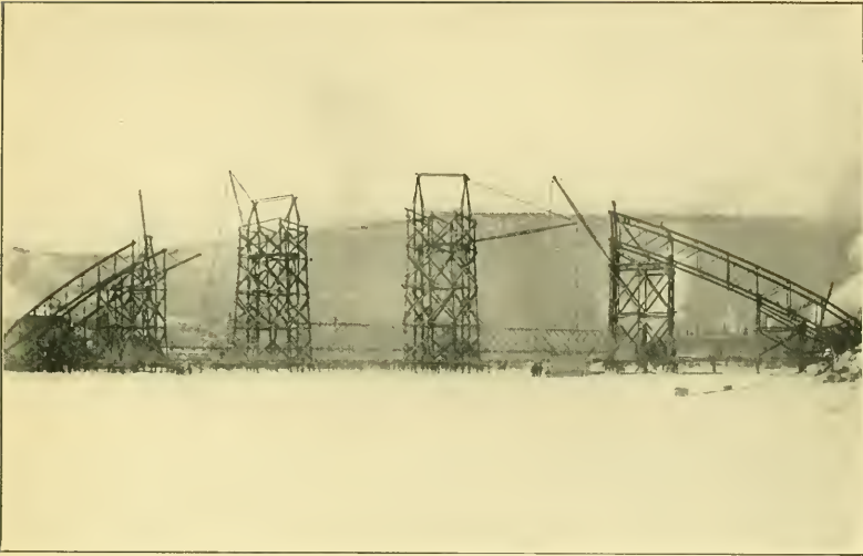
FIG. 1.—BELLOWS FALLS ARCH BRIDGE IN PROGRESS.
