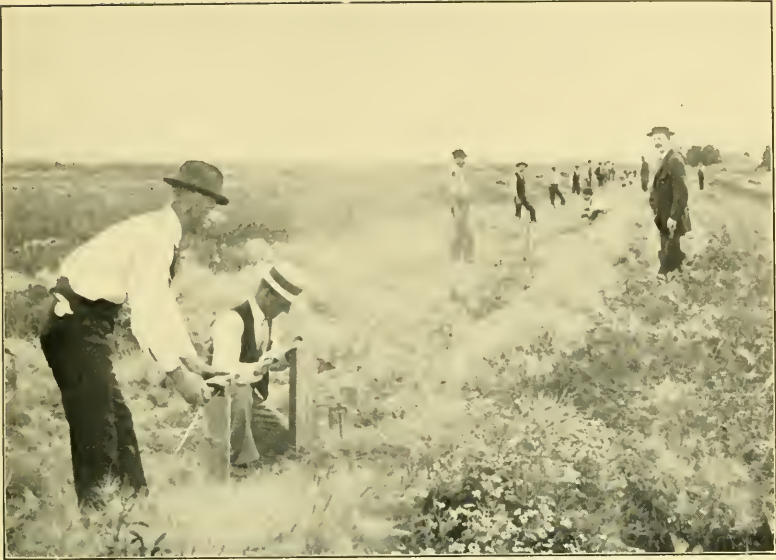
FIG. 1.—MEASURING FORT SNELLING BASE LINE WITH 900-FT. STEEL TAPE. REAR END OF TAPE.
