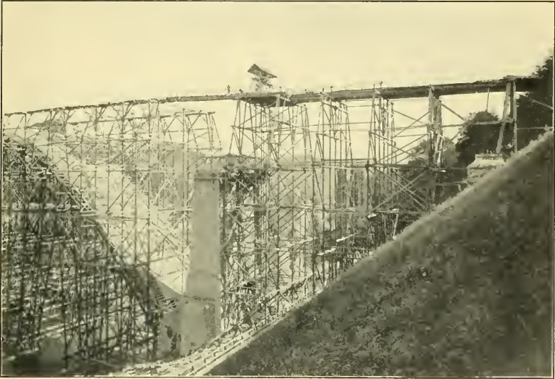
FIG. 1.—ERECTION OF THE KORNHAUS BRIDGE.
