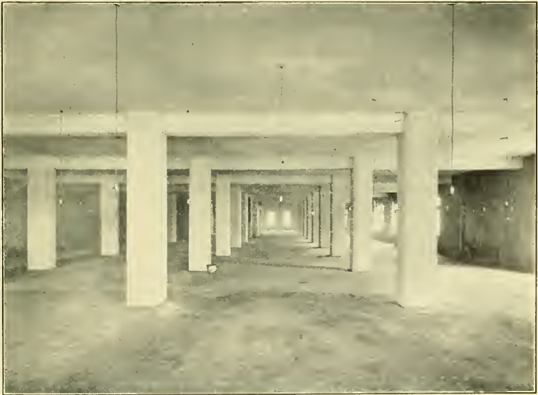
FIG. 2.—TYPICAL INTERIOR, SECOND TO SEVENTH STORIES, MANUFACTURERS' FURNITURE EXCHANGE BUILDING.
