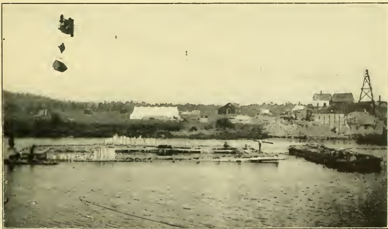
FIG. 2.—BUILDING COFFER-DAM OF PIER 3, SHOWING CABLEWAY.
