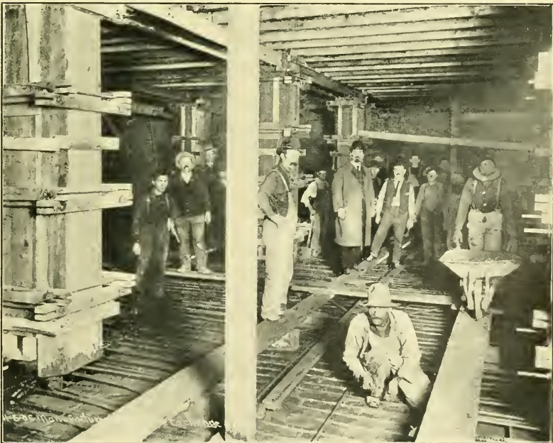
FIG. 2.—CONCRETING ON SECOND FLOOR, MANUFACTURERS' FURNITURE EXCHANGE BUILDING.
