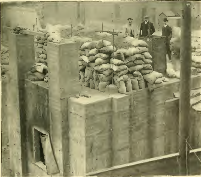
FIG. 2.—STONE CONCRETE HOUSE, WITH TEST LOAD, AFTER FOUR-HOUR FIRE TEST.
