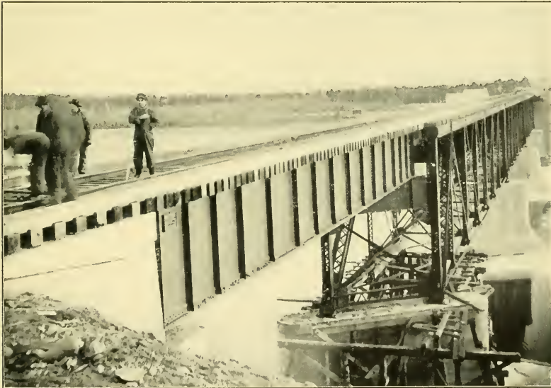
FIG. 2.—GENERAL VIEW OF COMPLETED BRIDGE.
