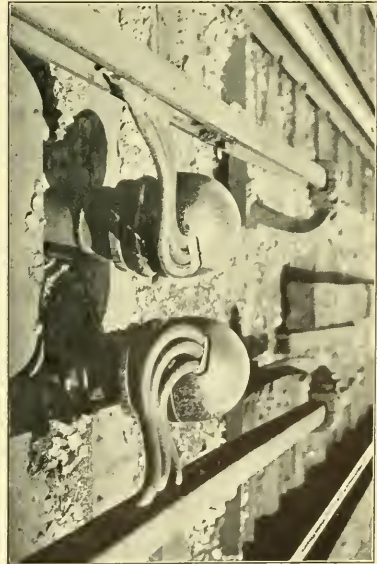
FIG. 3.—“Jumper” Connection between Direct-Current Feeder and Third-Rail.
