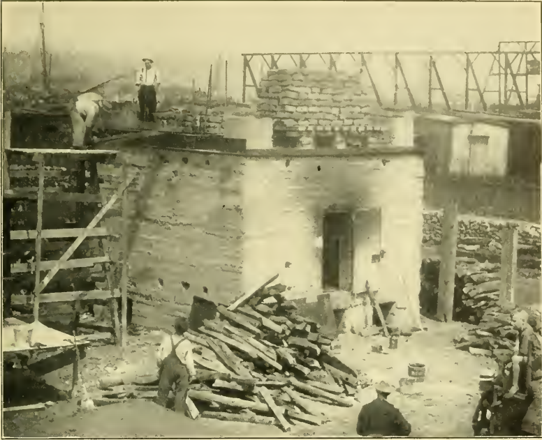
FIG. 1.—CINDER CONCRETE TEST HOUSE, AFTER FOURTH FIRE
