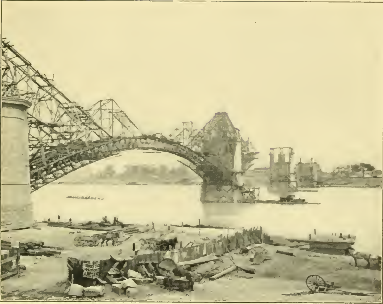
FIG. 1.—ERECTION OF THE EADS BRIDGE.
