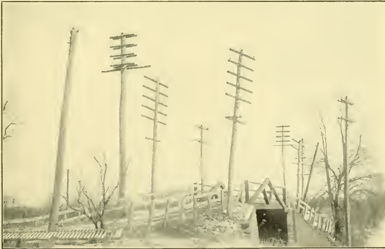
FIG. 2.—WIRE CRADLE OVER 11 000-VOLT TRANSMISSION LINE
