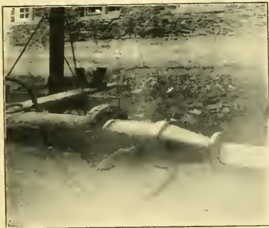
FIG. 3.—NOZZLE AT END OF 6-IN. PIPE LINE.
