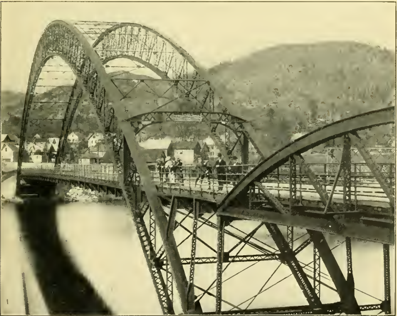
FIG. 2.—END VIEW, BELLOWS FALLS ARCH BRIDGE.
