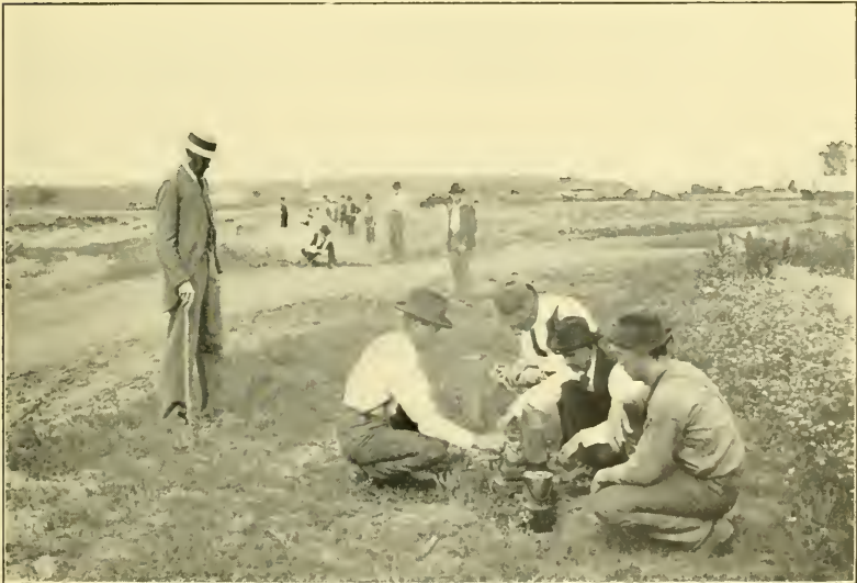
FIG. 2.—FRONT END OF TAPE. FORT SNELLING BASE LINE, SHOWING TENSION DEVICE.
