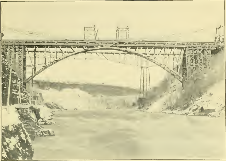
FIG. 1.—THE RAILROAD SUSPENSION, RAILROAD ARCH, AND CANTILEVER BRIDGES, AT NIAGARA.
