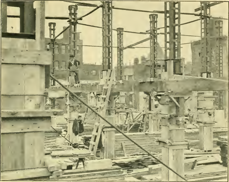
FIG. 1.—SECOND AND THIRD STORY COLUMN REINFORCING, WATSON BUILDING.
