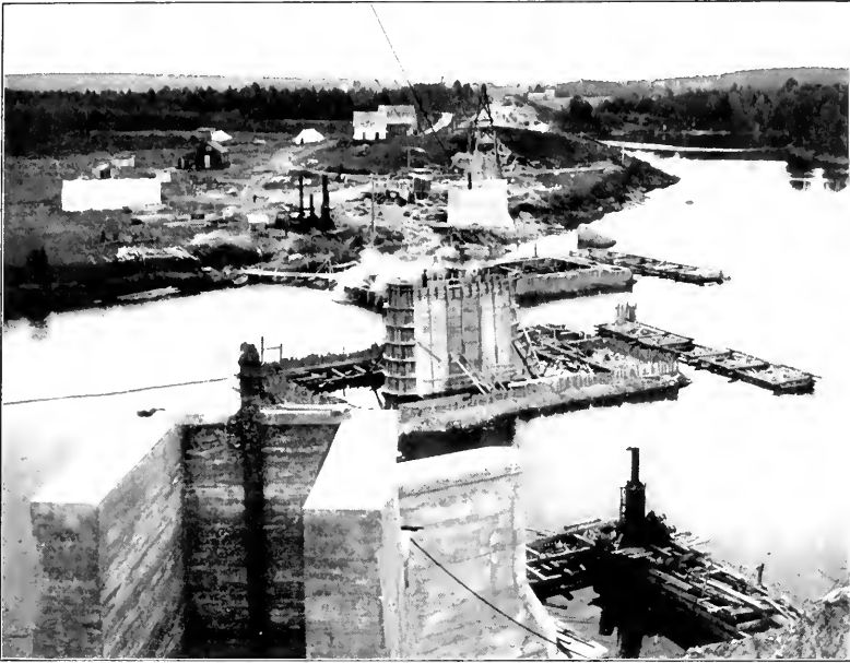
FIG. 1.—GENERAL VIEW, LOOKING SOUTH. NORTH ABUTMENT AND PIERS 1 AND 4 FINISHED, PIER 2 NEARLY COMPLETE, AND PIER 4 BEING EXCAVATED.
