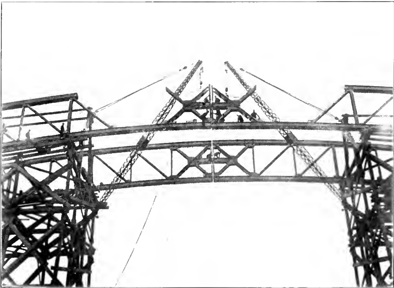
FIG. 2.- CONNECTING ARCH AT THE CENTER. (CAMERA POINTED UPWARD AT AN ANGLE OF 15 DEGREES.)
