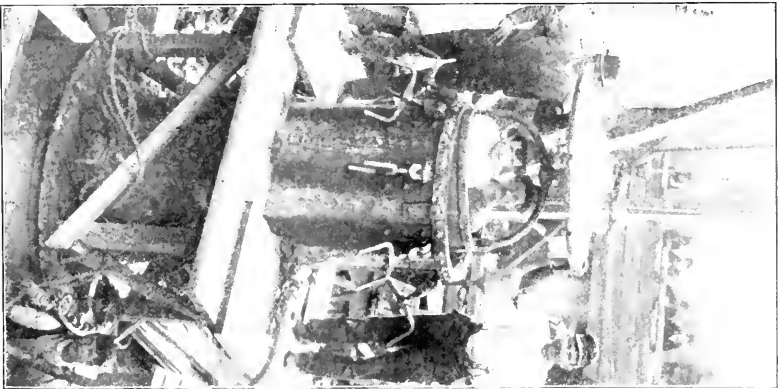
FIG. 3.—DETACHABLE AIR-LOCK DOOR.
