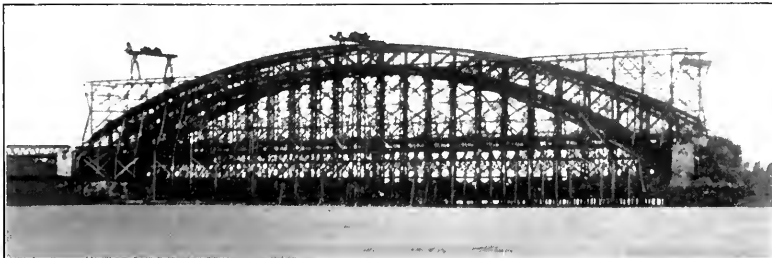
FIG. 3.—ERECTION OF THE DÜSSELDORF BRIDGE.
