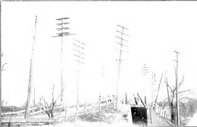
FIG. 2.—WIRE CRADLE OVER 11 000-VOLT TRANSMISSION LINE
