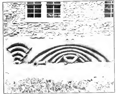
FIG. 4.—SIX-INCH, 90° CURVES, NOS. 1 TO 12.
