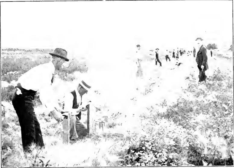
FIG. 1. MEASURING FORT SNELLING BASE LINE WITH 300-FT. STEEL TAPE. REAR END OF TAPE.
