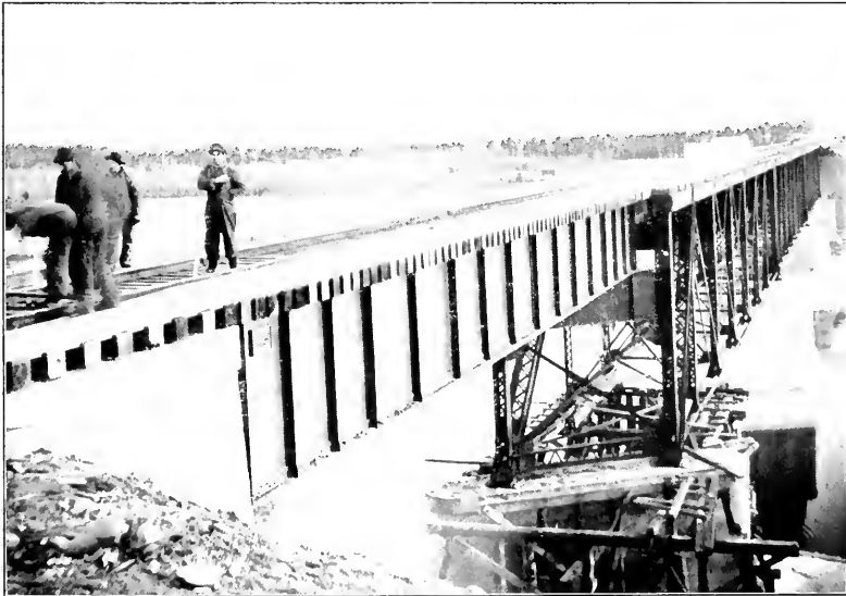
FIG. 2.—GENERAL VIEW OF COMPLETED BRIDGE.
