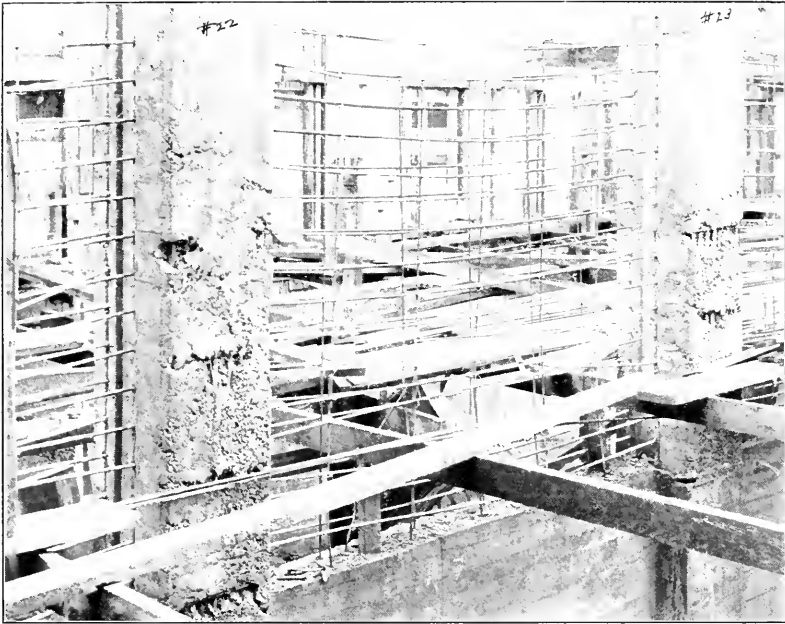
FIG. 1.— REINFORCEMENT OF WALLS AND COLUMNS.
