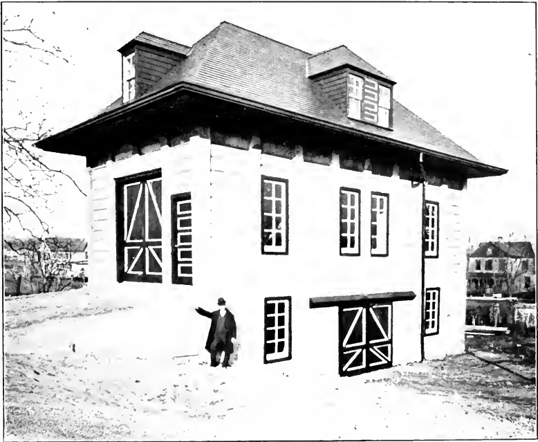
REINFORCED CONCRETE GARAGE AT WHITESTONE, LONG ISLAND
