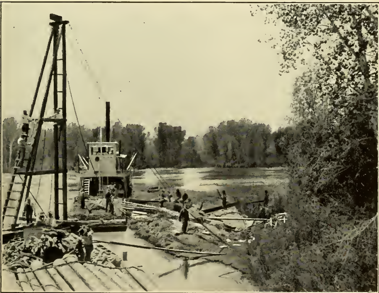
FIG. 2.—THIRD ATTEMPT TO CLOSE BREAK AT LOWER MEXICAN INTAKE, JUNE 1ST, 1905.
