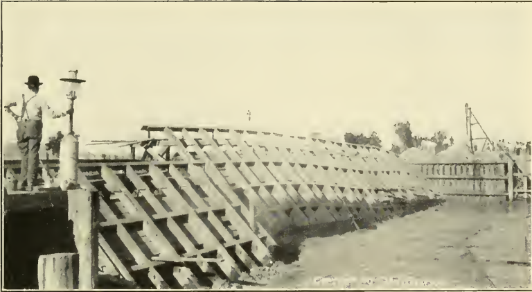
FIG. 1.—FAILURE OF ROCKWOOD GATE, OCTOBER 11TH, 1906.
