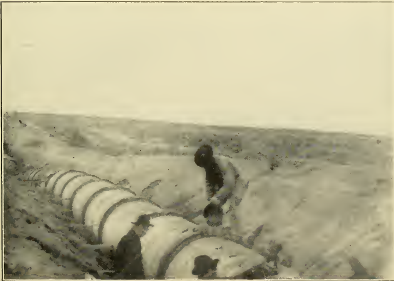
FIG. 2.—JOINTING 46-INCH CONCRETE PIPE, UMATILLA PROJECT.
