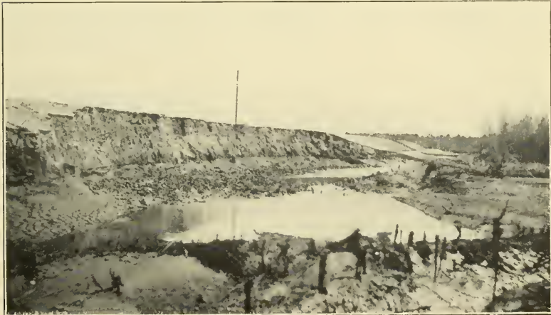
FIG. 2.—EFFECT OF FLOOD OF DECEMBER 7TH, 1906, ON LEVEE OF U. S. RECLAMATION SERVICE, OPPOSITE LOWER HEADING.
