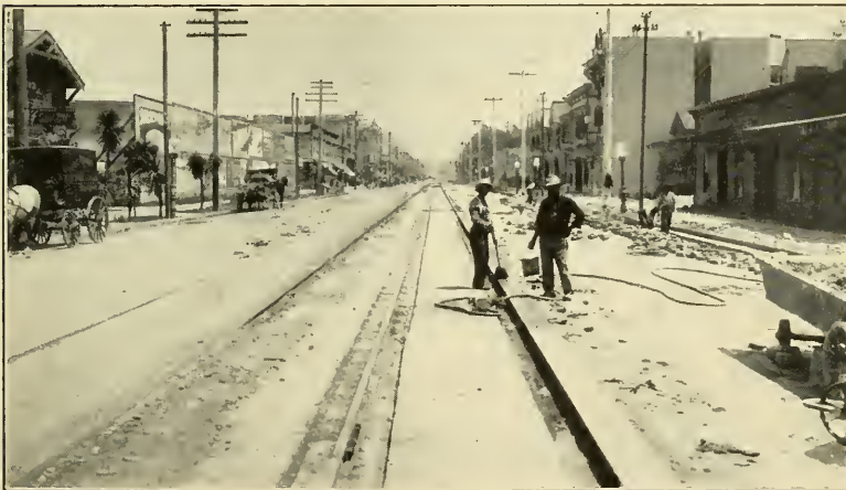
FIG. 2.—ASPHALT PAVING, BROADWAY, OAKLAND, CAL. BASALT BLOCK LINERS TOOTHING THE RAILS.
