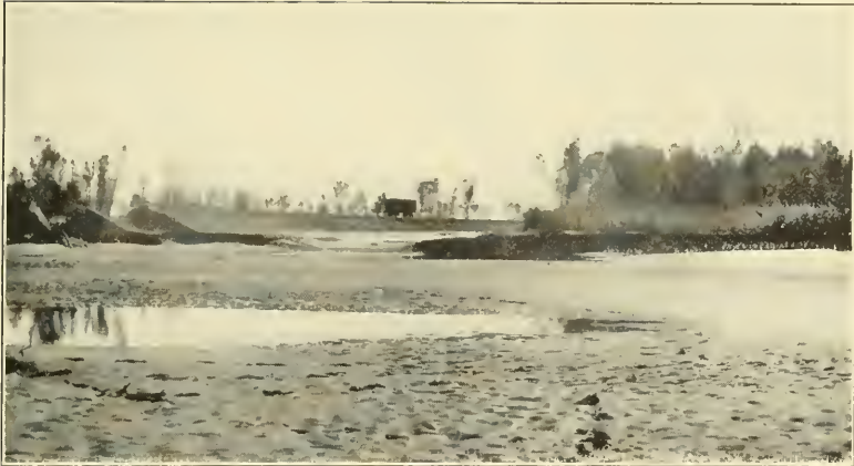
FIG. 1.—LEVEE FAILURES RESULTING IN SECOND BREAK, DECEMBER 7TH, 1906. NOTE THE SHORT LENGTH OF THE TWO GAPS.
