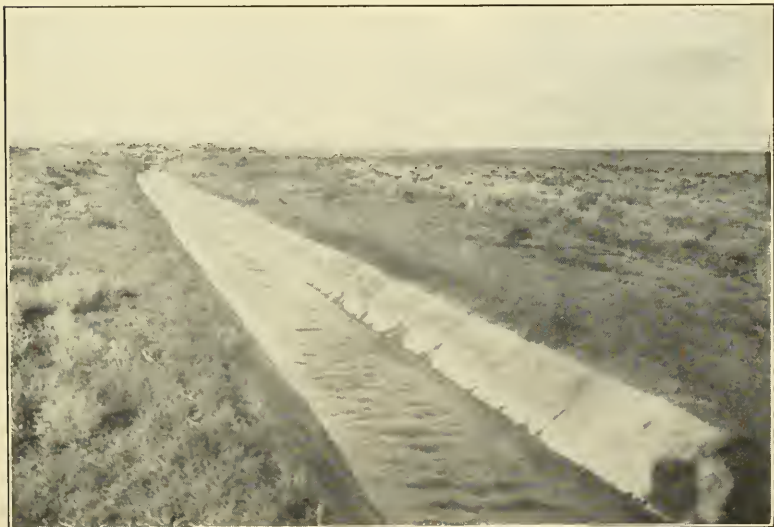
FIG. 2.—MORTAR-LINED LATERAL, UMATILLA PROJECT.
