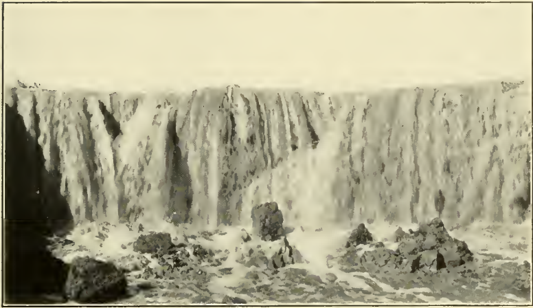
FIG. 1.—GRADE RECESSION IN NEW RIVER NEAR CALEXICO. MAXIMUM RATE OF RECESSION, 1 FOOT PER MINUTE. DROP, 28 FEET. JUNE, 1906.
