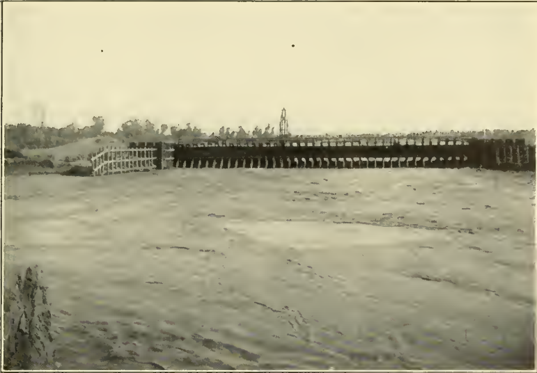
FIG. 1.—ROCKWOOD HEAD-GATE, OCTOBER 6TH, 1906, PASSING 12 000 SECOND-FEET.
