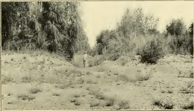
FIG. 2.—CONNECTING CHANNEL ERODED BETWEEN INTERRUPTED BORROW-PITS DURING SUMMER FLOOD, 1907.
