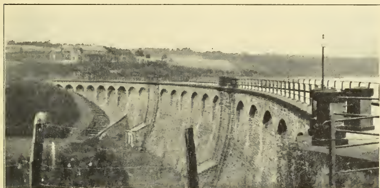
FIG. 2.—DAM BUILT BY ASSOCIATION FOR CONTROLLING FLOODS AND INCREASING LOW-WATER FLOW OF WUPPER RIVER, GERMANY.
