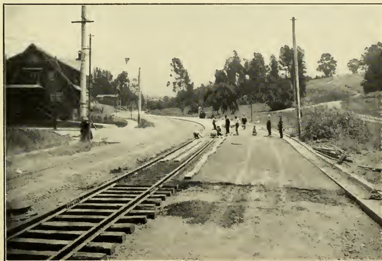
FIG. 2.—ASPHALT PAVING, FOURTH AVENUE, OAKLAND, CAL. VITRIFIED BRICK LINERS. ASPHALTIC CONCRETE BETWEEN TIES, INSTEAD OF HYDRAULIC CONCRETE.
