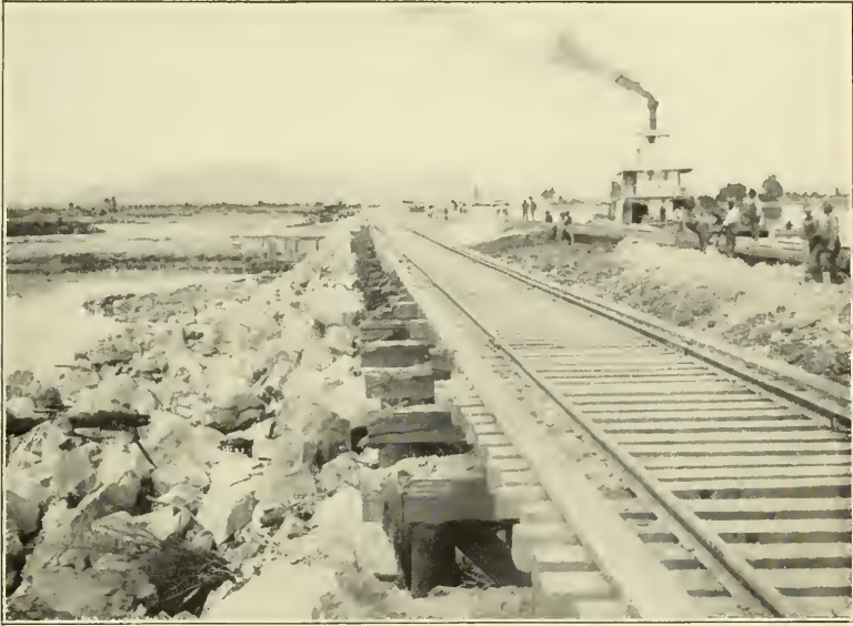
FIG. 1.—SEALING THE HIND DAM WITH GRAVEL AND CLAY BY HYDRAULIC JETS, NOVEMBER, 1906. NOTE SLOPE OF DOWN-STREAM SIDE OF ROCK FILL DAM.
