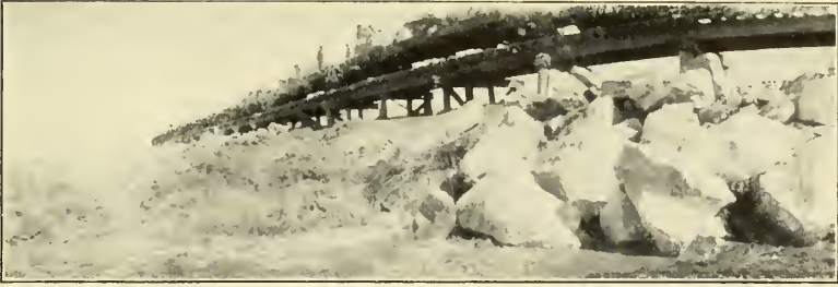
FIG. 1.—SECOND CLOSING. HEAD DEVELOPED, 8 FEET.
