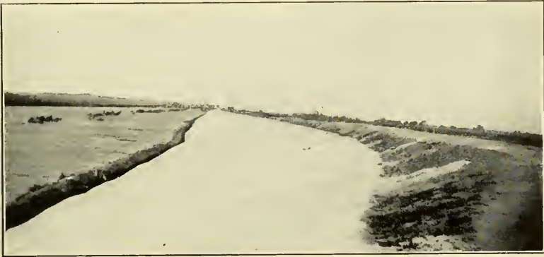
FIG. 2.—REINFORCED CONCRETE FACING, ON LEVEE 25 FEET HIGH, NEAR SACRAMENTO, CAL.
