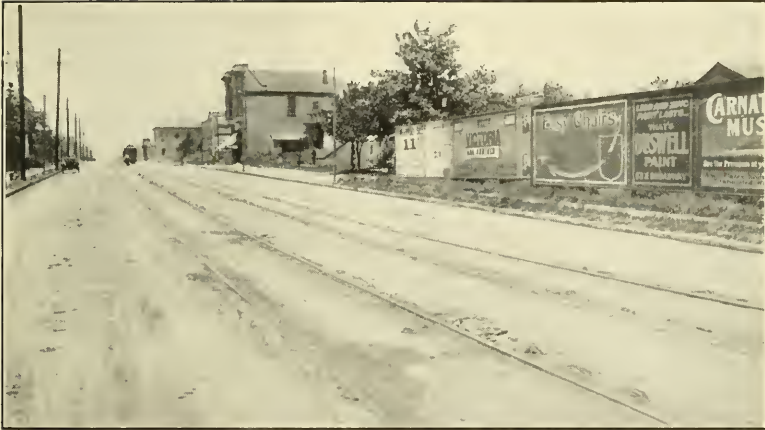
FIG. 1.—CONDITION OF ASPHALT PAVEMENTS ADJOINING CAR TRACKS WHERE NO LINERS ARE USED. OLD TYPE T-RAIL, AND LIGHT CONCRETE FOUNDATION BETWEEN TRACKS.
