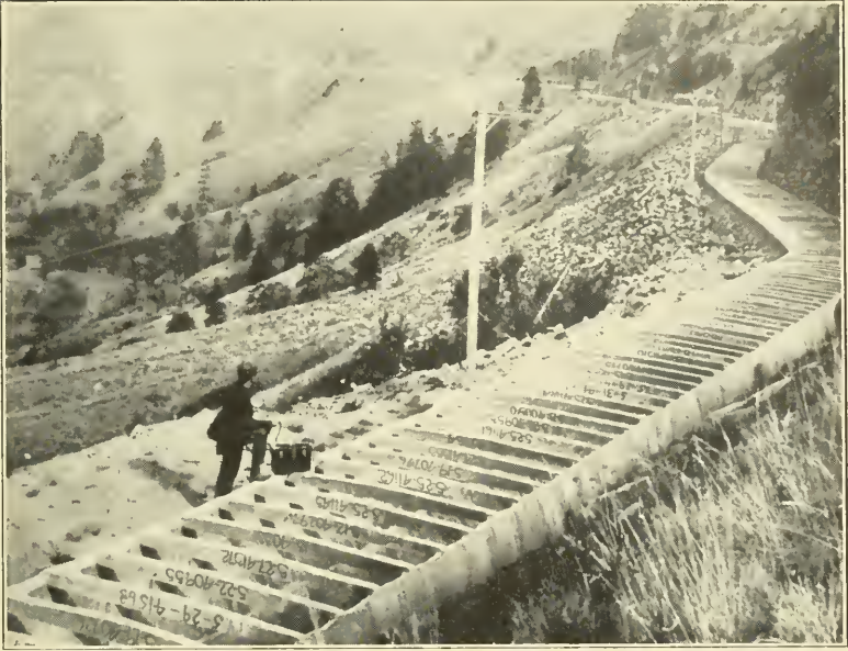
FIG. 1.—TETON MAIN CANAL, CONCRETE LINED.
