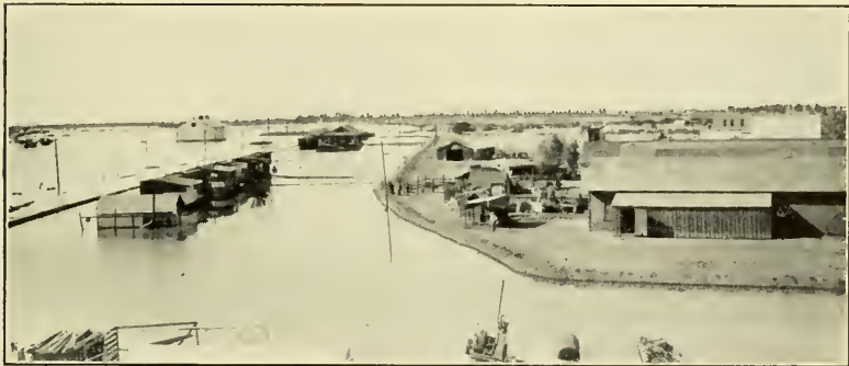
FIG. 2.—PORTION OF 4-MILE LEVEE PROTECTING CALEXICO AND MEXICALI, IN FLOOD OF JUNE, 1906.
