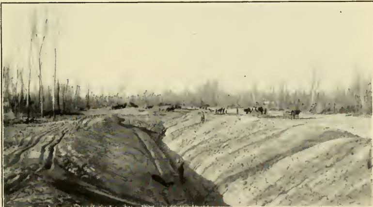
FIG. 2.—MUCK-DITCH CONSTRUCTION IN LEVEE EXTENSION WORK, 1907.
