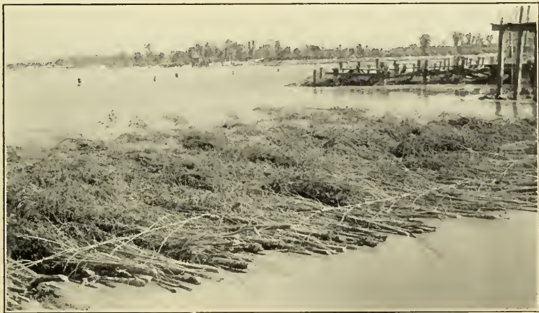
FIG. 2.—DOWN-STREAM END OF BRUSH MATTRESS ABOVE WATER BECAUSE OF SILTING ACTION.
