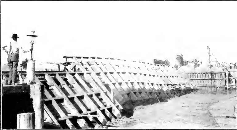
FIG. 1.—FAILURE OF ROCKWOOD GATE. OCTOBER 11TH, 1906.
