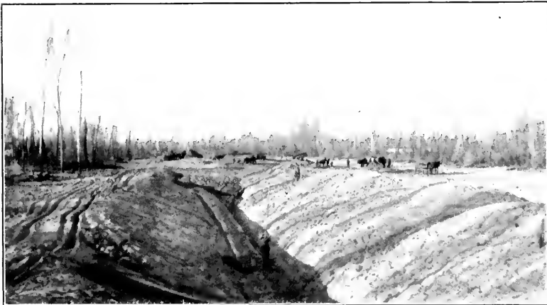
FIG. 2.—MUCK-DITCH CONSTRUCTION IN LEVEE EXTENSION WORK, 1907.
