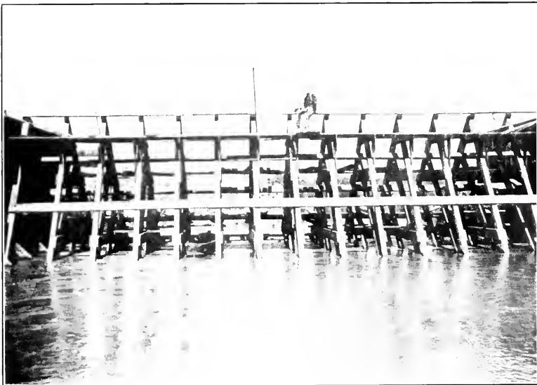
FIG. 2.—ORIGINAL INTAKE (CHAFFEY) GATE, IMPERIAL CANAL, COMPLETED IN 1901.
