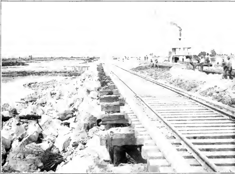
FIG. 1.—SEALING THE HIND DAM WITH GRAVEL AND CLAY BY HYDRAULIC JETS, NOVEMBER, 1906. NOTE SLOPE OF DOWN-STREAM SIDE OF ROCK FILL DAM.
