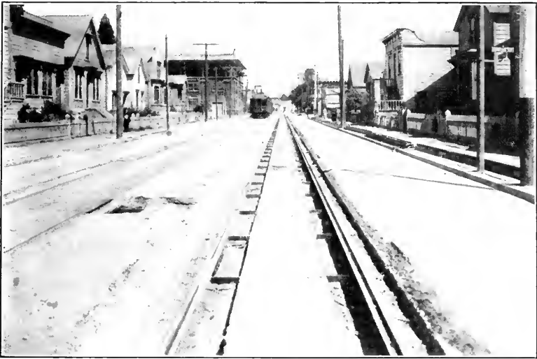
FIG. 1.—ASPHALT PAVING, TWENTY-SECOND STREET, OAKLAND, CAL. GIRDER-RAILS, STEEL TIE-PLATES, WOODEN TIES, CONCRETE TO BASE OF TIE, BASALT BLOCK LINERS ON 1\frac{1}{2} -IN. SAND CUSHION.
