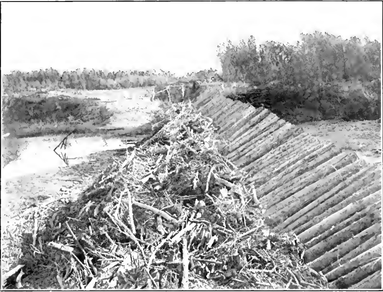
FIG. 1.—TYPICAL ABATIS WORK ON LEVEES OF YUMA PROJECT. U. S. RECLAMATION SERVICE.
