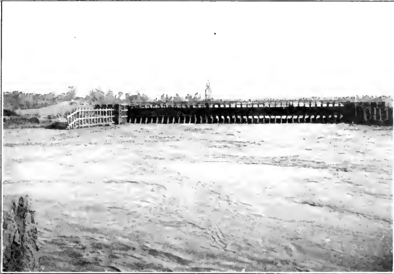
FIG. 1.—ROCKWOOD HEAD-GATE, OCTOBER 6TH, 1906, PASSING 12 000 SECOND-FEET.
