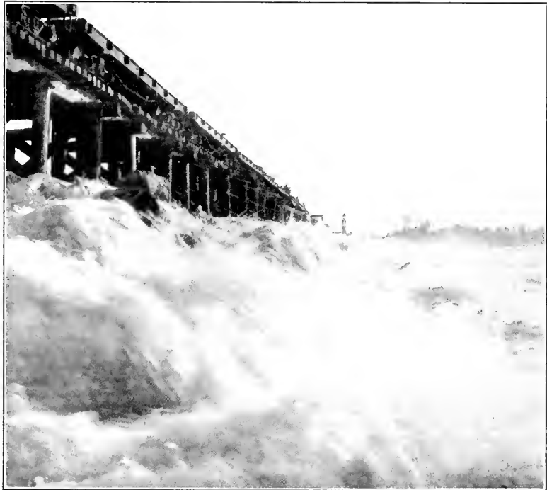
FIG. 2.—THE HIND DAM, PASSING 7 000 SECOND-FEET. HEAD, 10 FEET.
