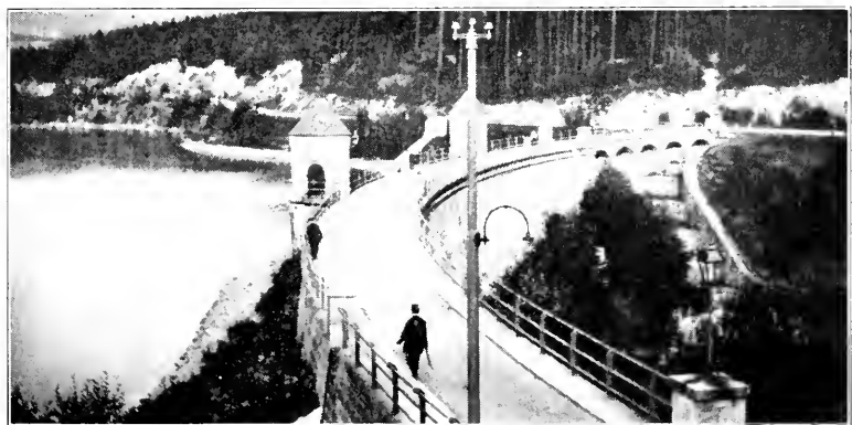
FIG. 3.—DAM BUILT BY ASSOCIATION FOR CONTROLLING FLOODS AND INCREASING LOW-WATER FLOW AT REICHENBERG, BOHEMIA.
