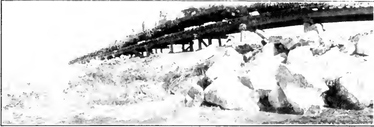
FIG. 1.—SECOND CLOSING. HEAD DEVELOPED, 8 FEET.
