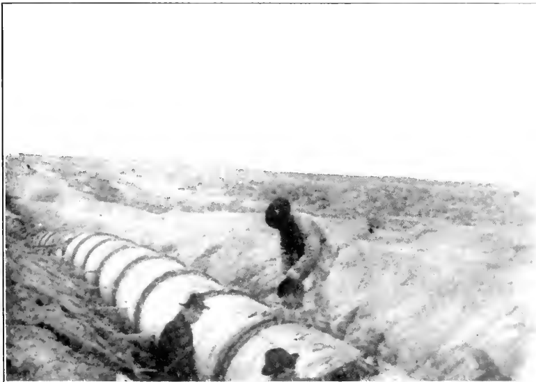
FIG. 2.—JOINTING 46-INCH CONCRETE PIPE, UMATILLA PROJECT.
