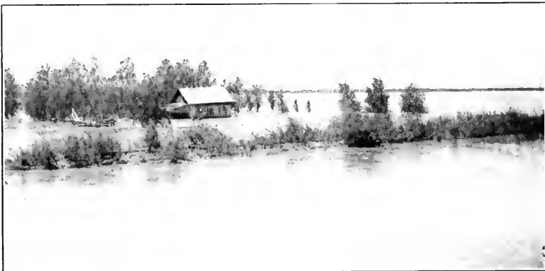
FIG. 3.—OVERFLOW AGAINST WEST AND SOUTH BANKS OF MAIN CANAL NEAR FIVE GATES, 2½ MILES NORTHWEST OF CALENICO.
