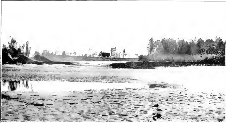
FIG. 1.—LEVEE FAILURES RESULTING IN SECOND BREAK, DECEMBER 7TH, 1906. NOTE THE SHORT LENGTH OF THE TWO GAPS.
