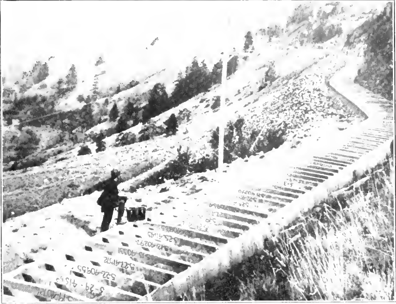
FIG. 1.—TIETON MAIN CANAL, CONCRETE LINED.
