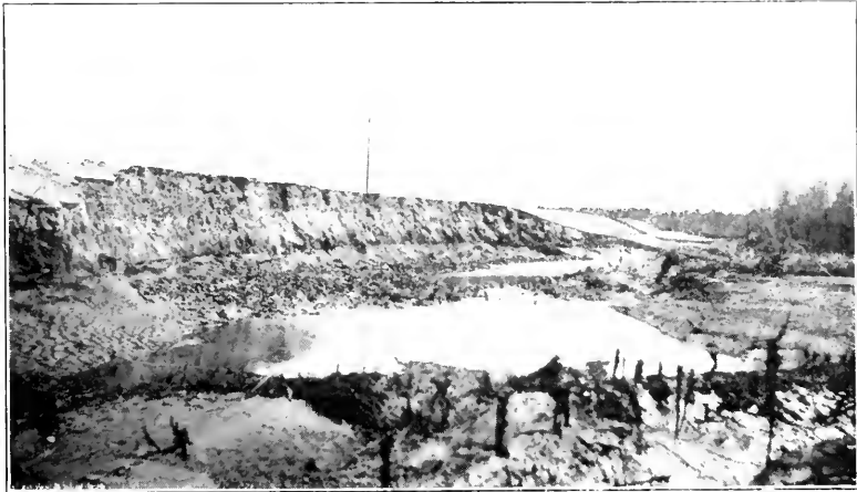
FIG. 2.—EFFECT OF FLOOD OF DECEMBER 7TH, 1906, ON LEVEE OF U. S. RECLAMATION SERVICE, OPPOSITE LOWER HEADING.
