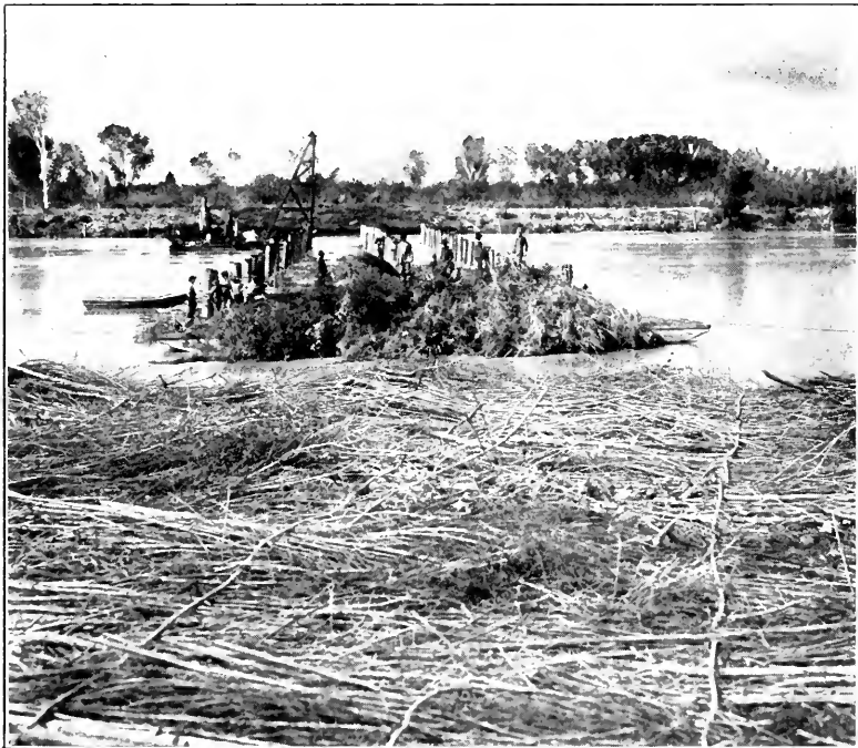
FIG. 2.—EDINGER DAM, NOVEMBER 8TH, 1905. BRUSH AND WIRE MAT IN FOREGROUND, READY TO BE PLACED.
