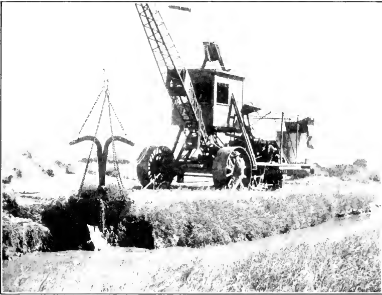
FIG. 1.—STOCKTON CLAM-SHELL DREDGE CLEANING CANALS IN IMPERIAL VALLEY.
