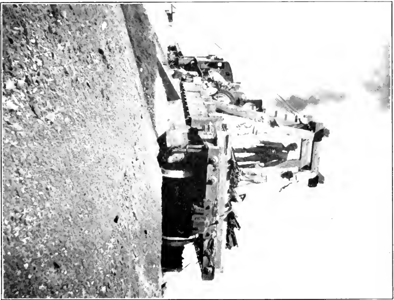
FIG. 2.—GRAVEL SPREADER IN OPERATION.
