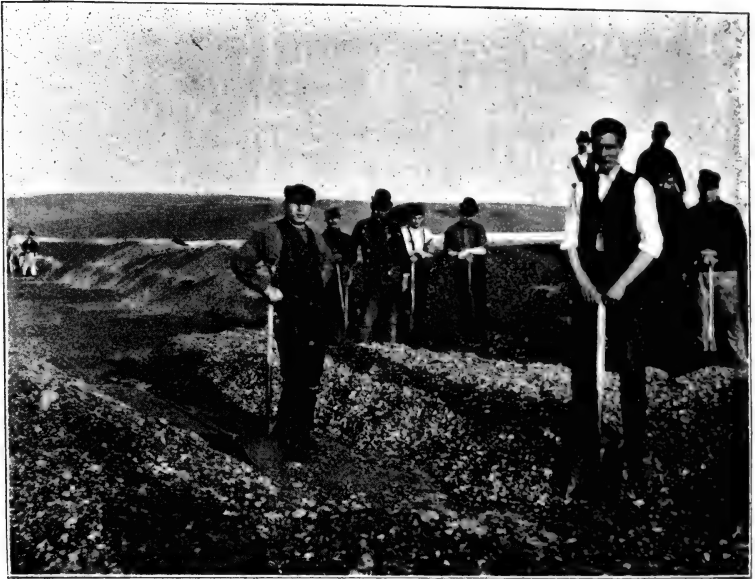
3.—MEN CLEARING SHINGLE FROM ROAD ABOUT HALF WAY BETWEEN OLD GATEHOUSE AND COASTGUARD STATION AFTER STORM OF FEB. 13TH, 1899. PHOTO FEB. 16TH, 1899.
