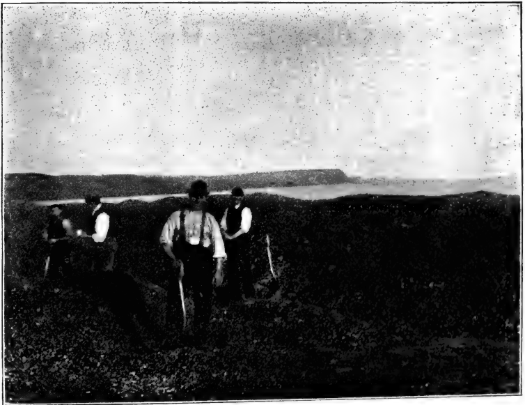
4.—MEN CLEARING SHINGLE FROM ROAD (NEARER COASTGUARD STATION THAN 3). SHINGLE 3FT. DEEP OR MORE OVER ROAD.
