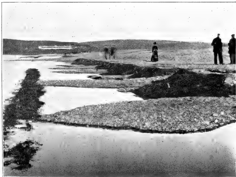
2.—VIEW OF LODMOOR SIDE OF BEACH, SHEWING DAMAGE TO ROAD AND SHINGLE PROMONTORIES WASHED INTO LODMOOR.
