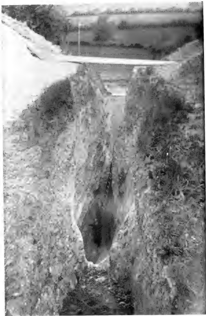
View of Excavation looking West, showing River in valley.
