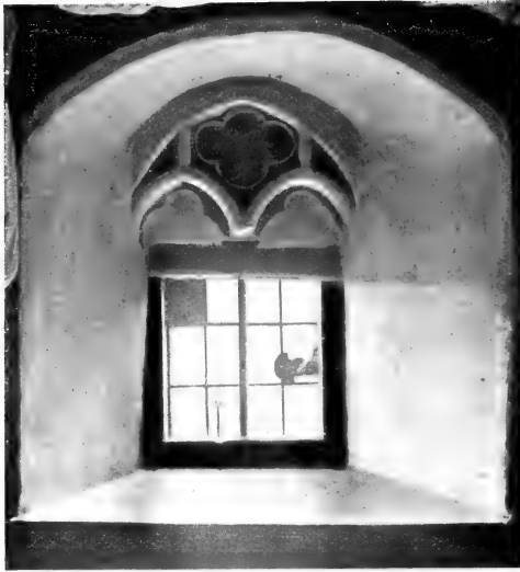
“The Lodge Farm,” Kingston Lacy. Window on 1st Floor of S. Front (from inside).
