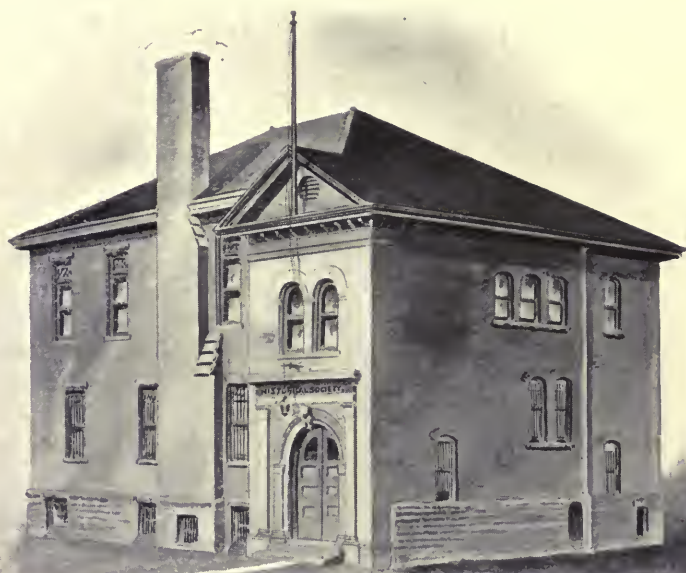
No. 4. The Wyoming Historical and Geological Society Building, Wilkes-Barre, Pa., 1908.
