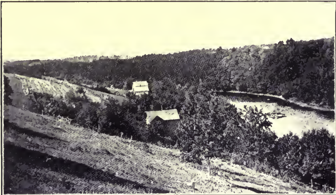
Site of the Wachusett Dam on the Nashua River near Clinton, Mass.
