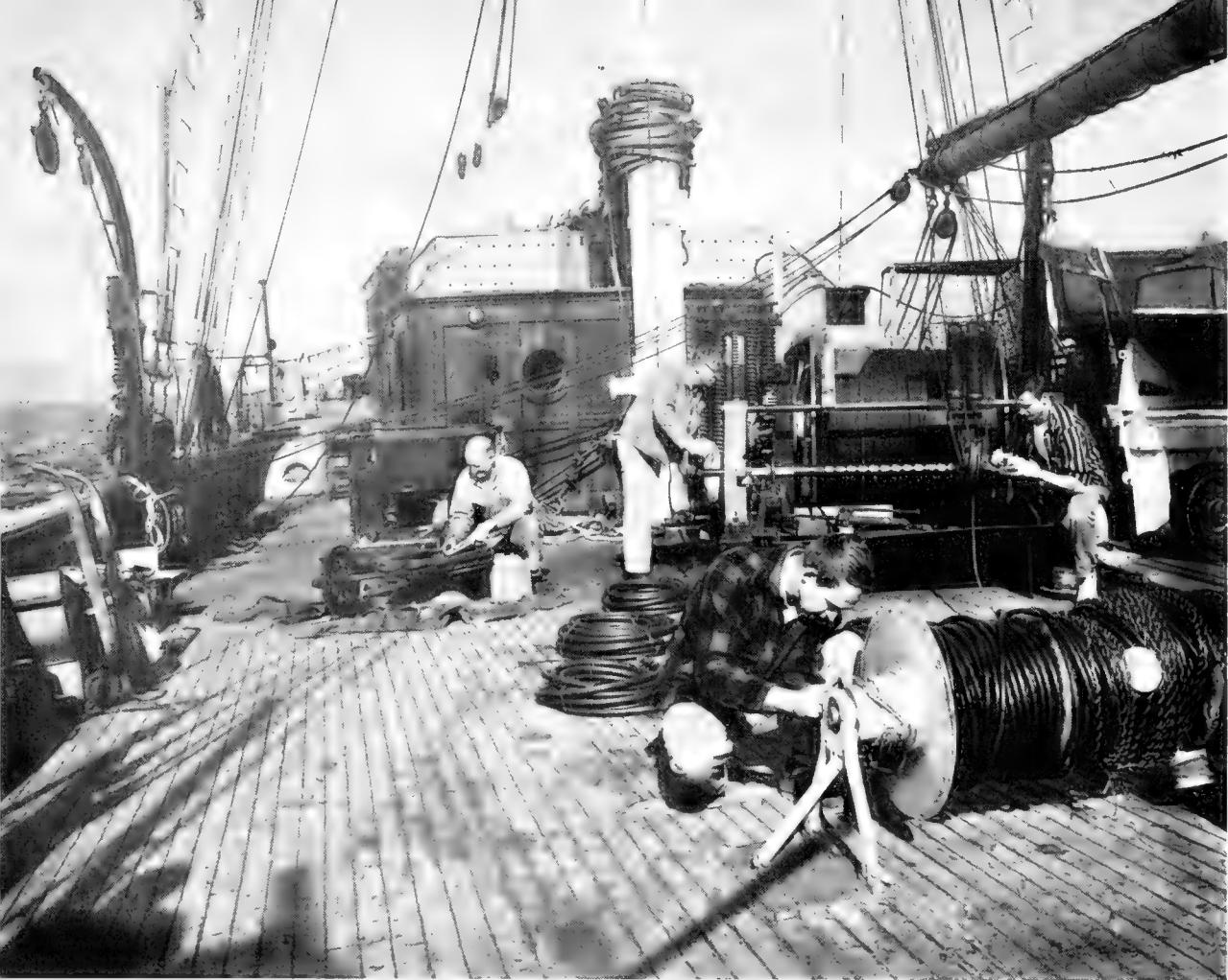
FIGURE 17.1 DEEP SEA TRAWL WINCH
