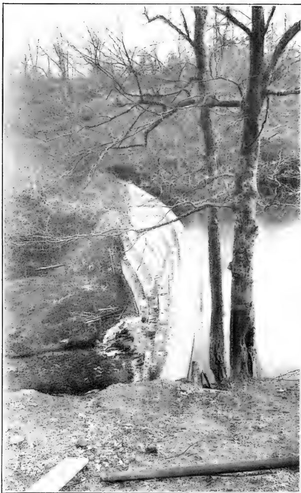
Fig. 3. Indiana University water-works dam from above north end, showing arching up-stream.
