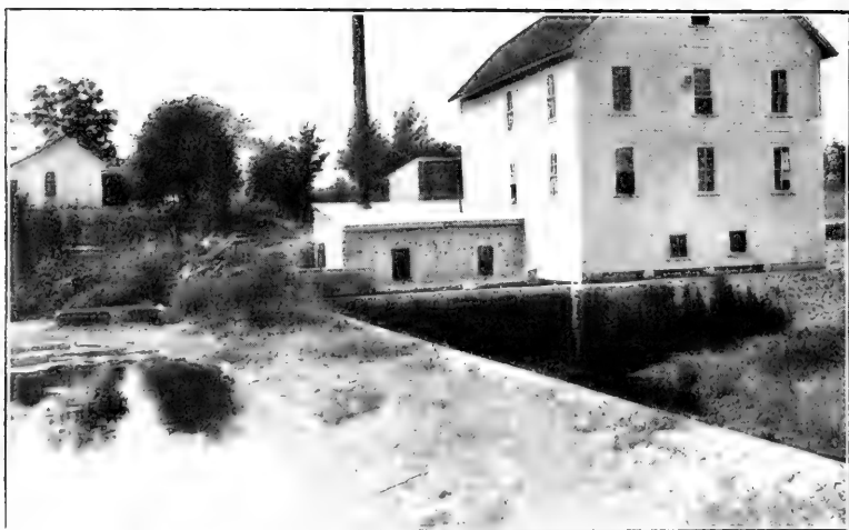
The Dam From Above.
