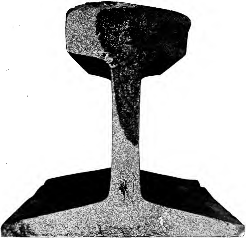
FAILED RAIL (CARNEGIE) ROLLED 7-96. FROM WRECK AT SHENANDOAH JUNCTION.
