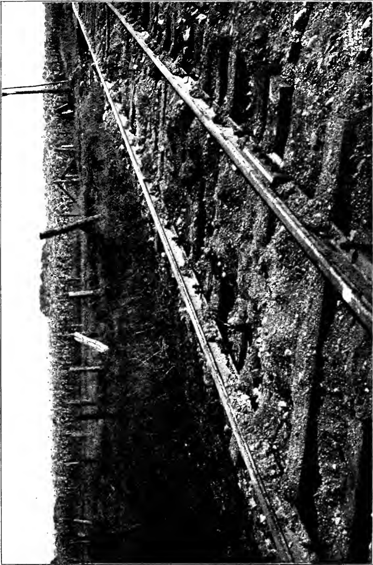
Screw-Spikes Ready to Be Driven by Machine.
