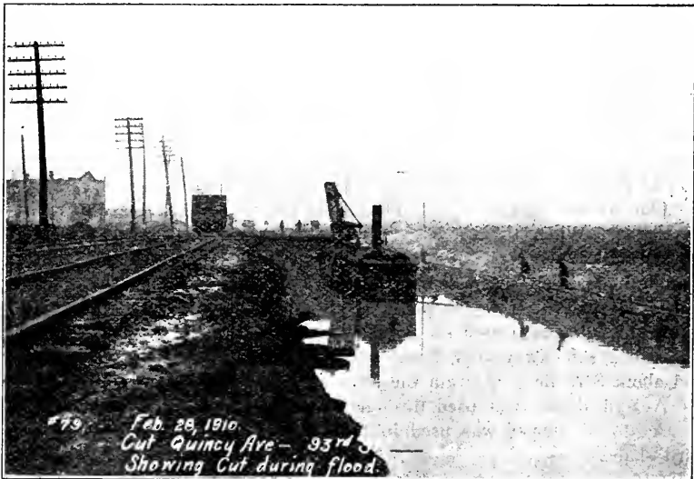
FIG. 4—FLOOD IN STEAM SHOVEL CUT.
