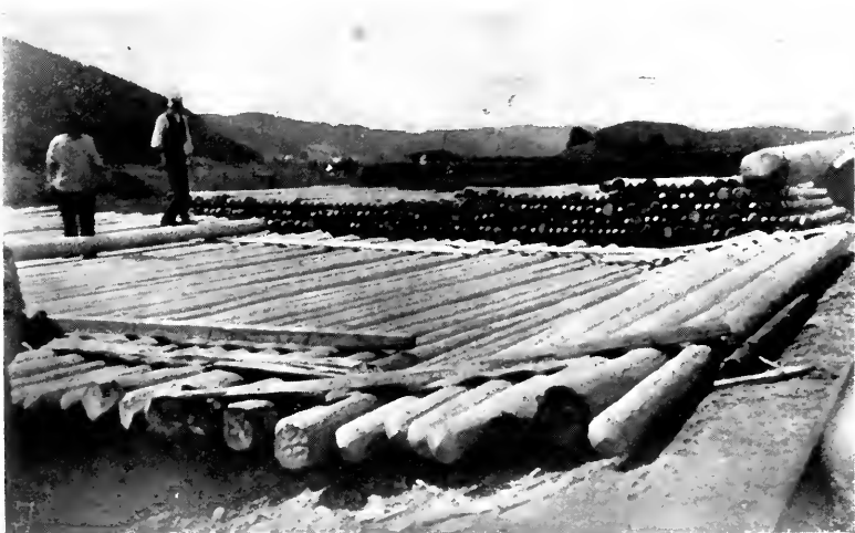
Fig. 2.—Right Method of Piling Poles for Seasoning.
