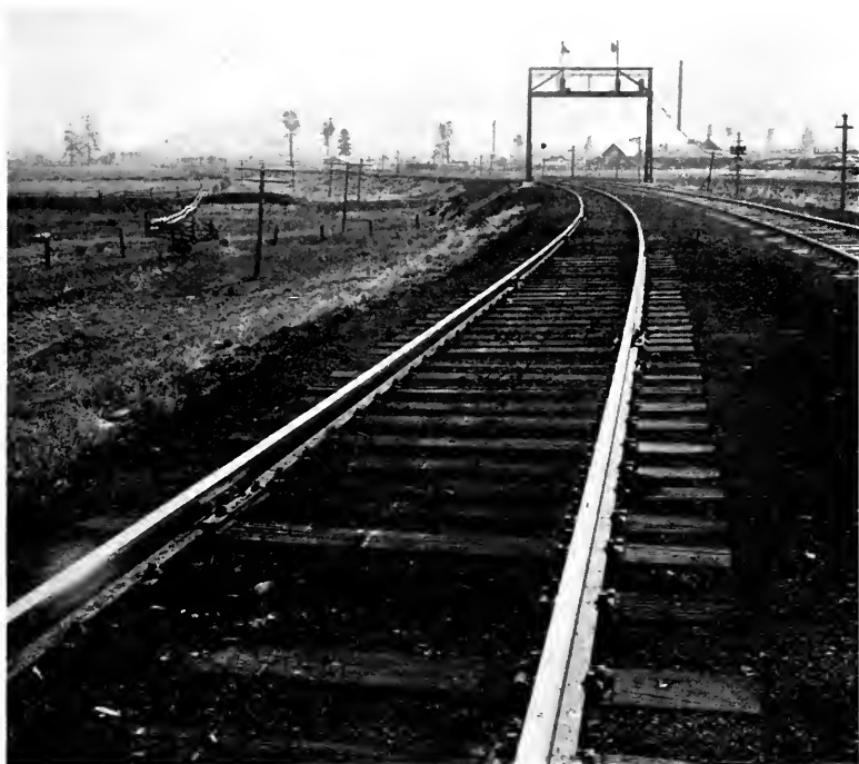
View 24, Albuquerque Division. Eucalyptus ties, standard construction screw spikes.
