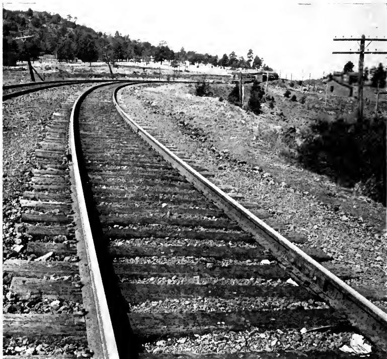
View 12, Albuquerque Division. Japanese oak, standard construction screw spikes.
