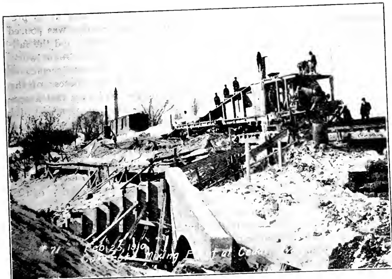
FIG. 8—SERVING MIXER WITH WHEELBARROWS.
