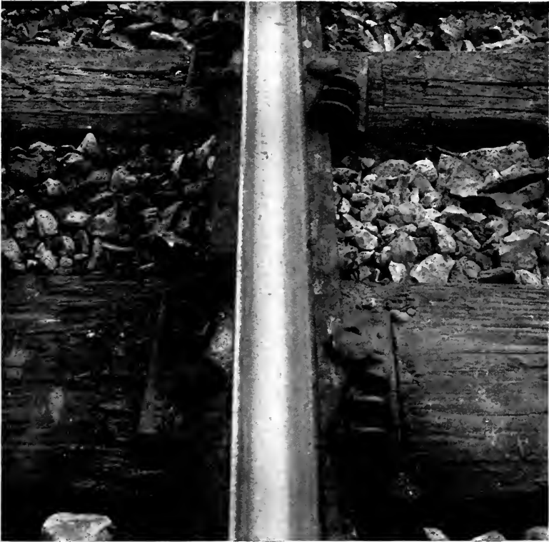
Betts anti-creeper tie plate, just outside Holliday Station.
