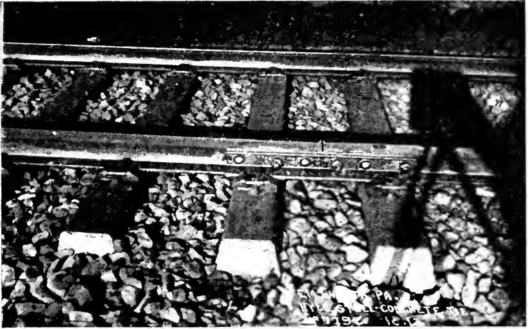
FIG. 14—HYLE STEEL-CONCRETE TIE, PENNSYLVANIA LINES, EMSWORTH, PA.
