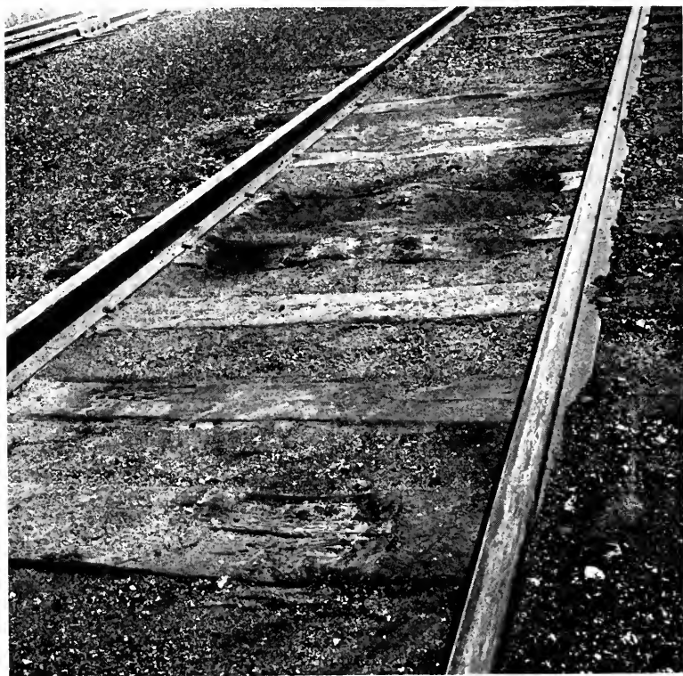
No. 2, View 24, Colorado Division. Oil-treated ties, inserted 1909.
