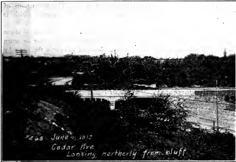
FIG. 22—CEDAR AVENUE BRIDGE.
