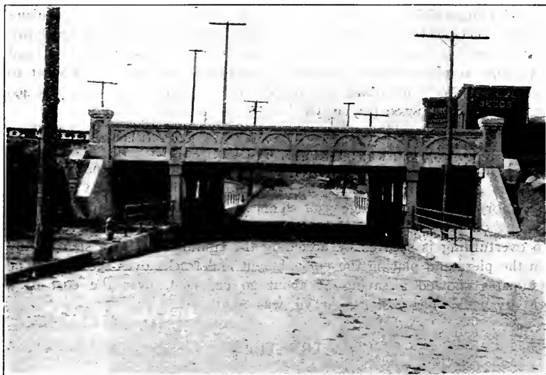
FIG. 24—MAYFIELD ROAD BRIDGE.
