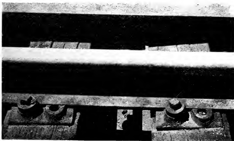
SCREW SPIKES AND MALLEABLE IRON TIE PLATES APPLIED JUNE, 1910. WEST END BRIDGE No. 42, WESTBOUND TRACK, OUTSIDE SOUTH RAIL.
