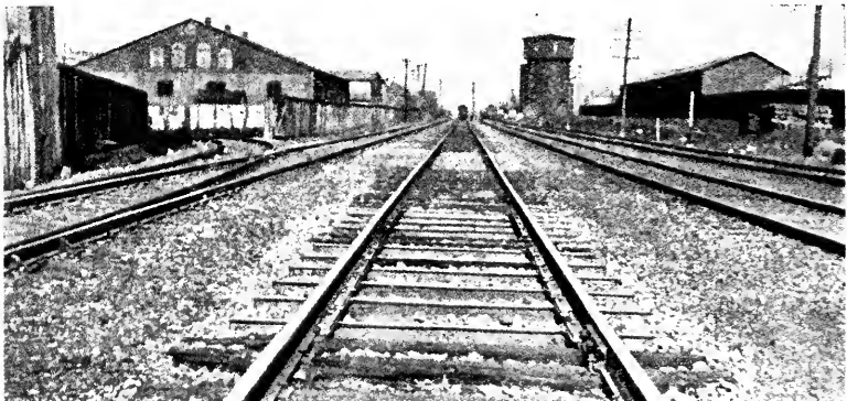
FIG. 19—MAXEY STEEL TIE, PITTSBURGH & LAKE ERIE RAILROAD.
