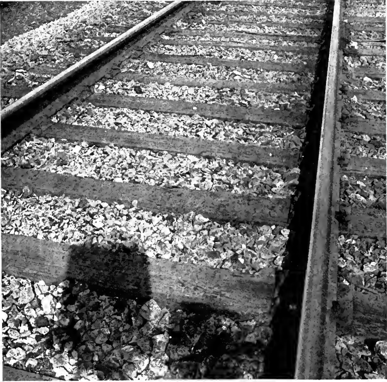
View 1, Western Division. Ohia hewn ties, standard construction screw spikes.
