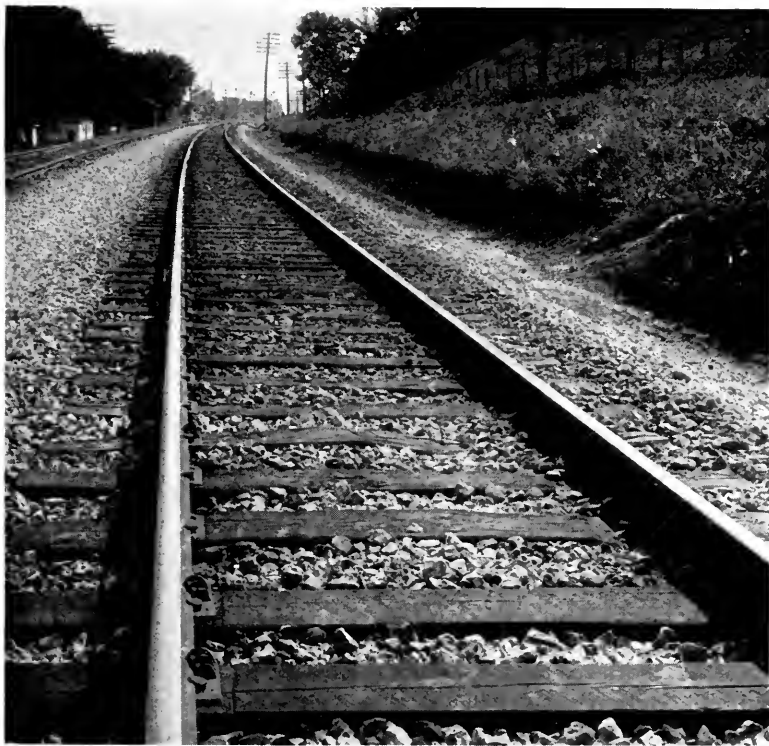
Betts anti-creeper tie plate, on curve just west of Turner Station.
