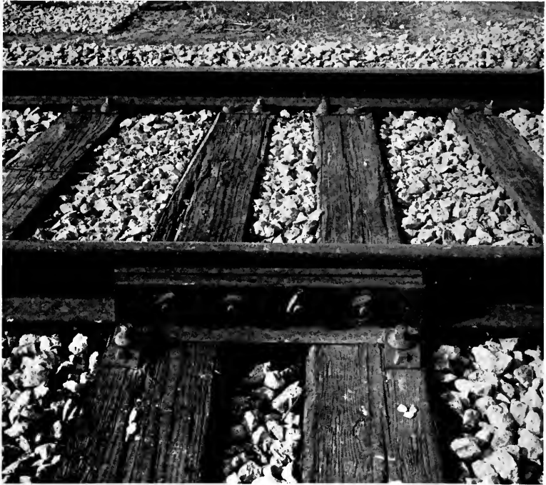
Specialties used in Experimental Track, Sylvania to Kinsley. View 21. Western Division, Weber Joint with screw spike requiring lugs.
