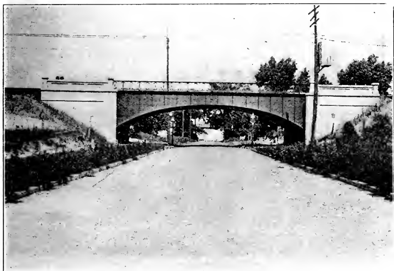
FIG. 18—ARCH BRIDGE AT EDDY ROAD.
