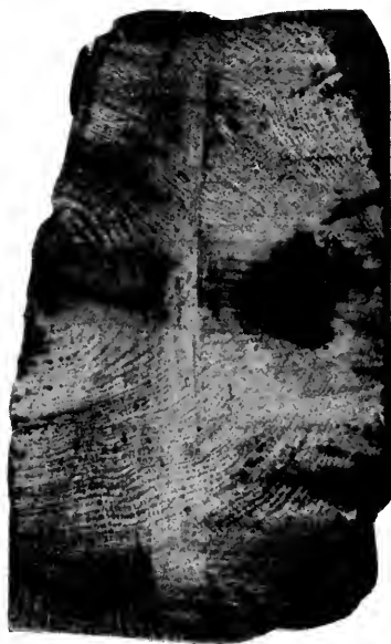
Creosote and Tar. Weight, 126 lbs. Absorption, 111 lbs.
