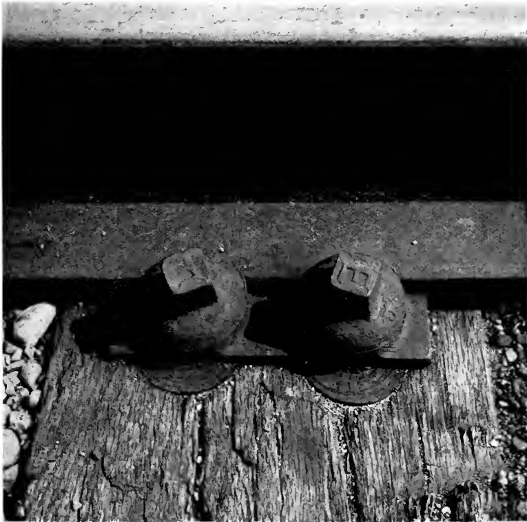
No. 1, View 22. Red Oak Tie. Second-hand, dowelled with oak dowels in the field by the Kendrick Dowelling Machine.
