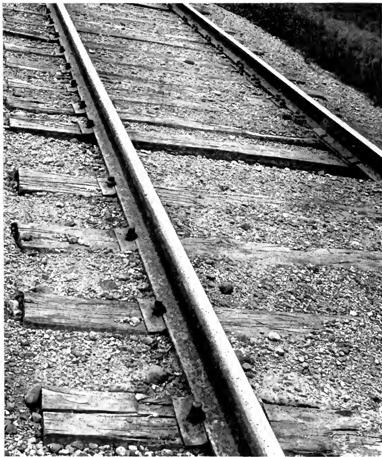
View 20, Illinois Division, same as above. Note, these were inserted 1909, and ties have to be spaced once a year.
