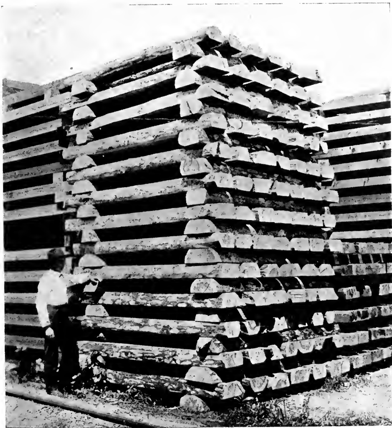
Plate I. Fig. 1.—7x2 Form. TIES PILED FOR RAPID SEASONING.
