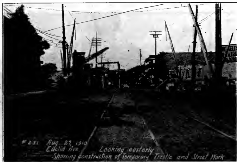
FIG. 35—TRESTLE OVER EUCLID AVENUE.
