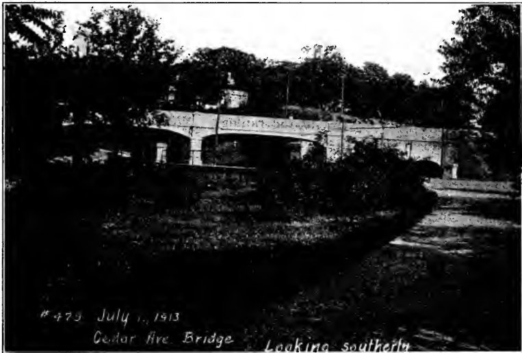
FIG. 23—CEDAR AVENUE BRIDGE.
