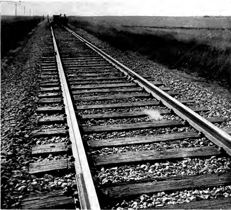
View 22, Western Division. Hewn gum, standard construction screw spikes.
