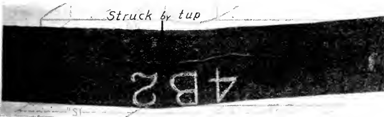
FIG. 6—VIEW OF BASE OF RAIL TESTED WITH THE HEAD IN TENSION IN THE DROP TEST, SHOWING HOW A SEAM IN THE BASE OPENED WHERE STRUCK BY THE TUP, SPLITTING THE BASE.
