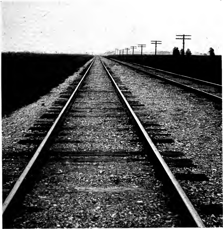
No. 1, View 11, Illinois Division. Screw spikes inserted with plates, without shoulder.
