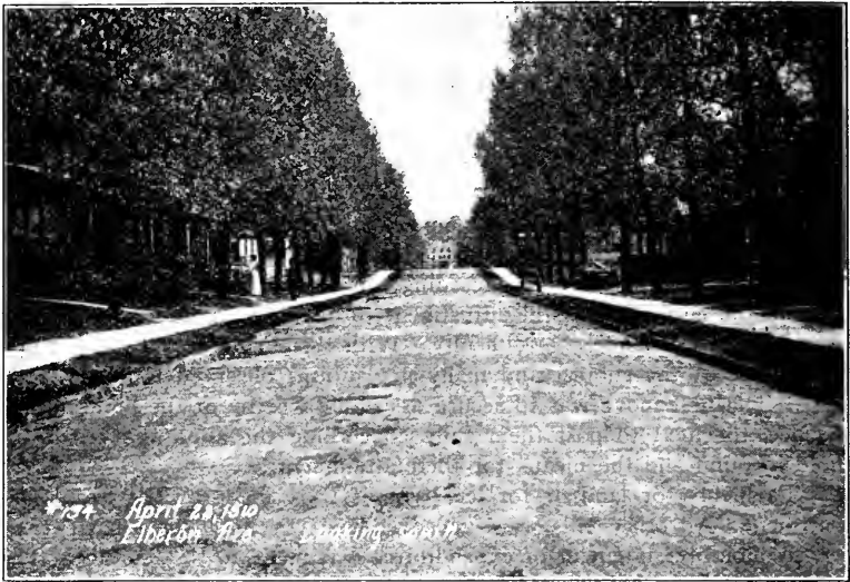
FIG. 38—ELBERON AVENUE, EAST CLEVELAND, BEFORE SEPARATION OF GRADES.
