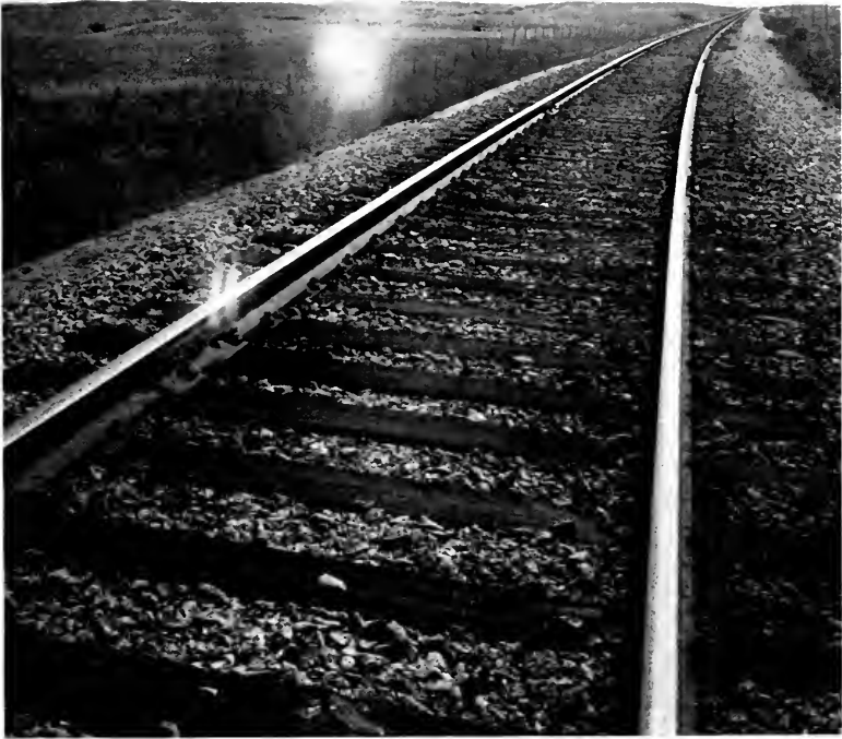
No. 6. View 11, Western Division, showing stretch of sawn pine ties, doweled in 1910.
