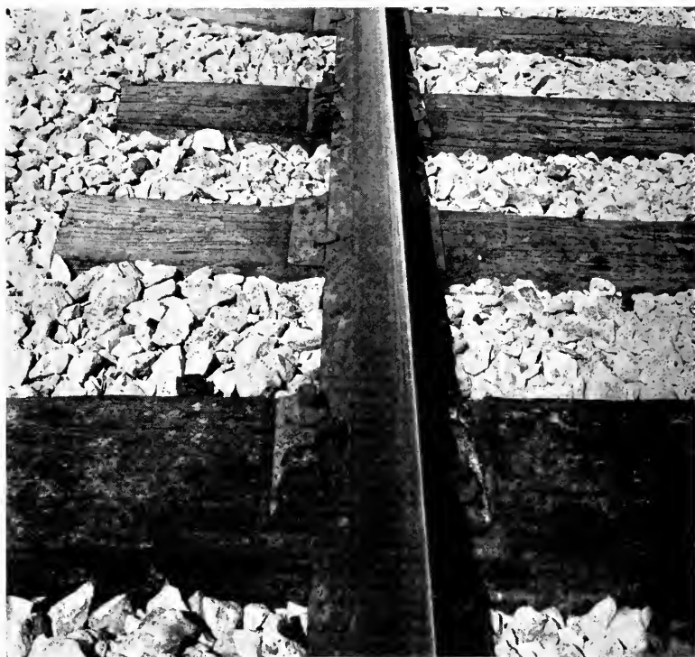
No. 5, View 2, Western Division, showing Positive tie plate with screw spike.
