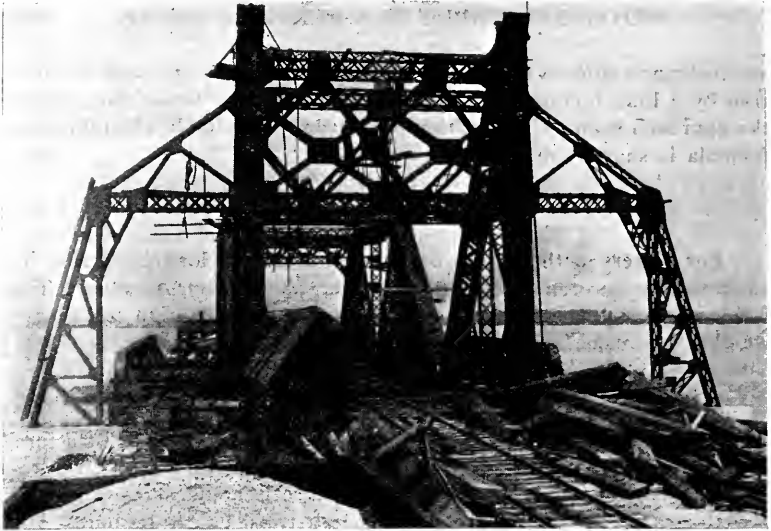
BASCULE BRIDGE OVER PORTAGE RIVER, PORT CLINTON, OHIO.
