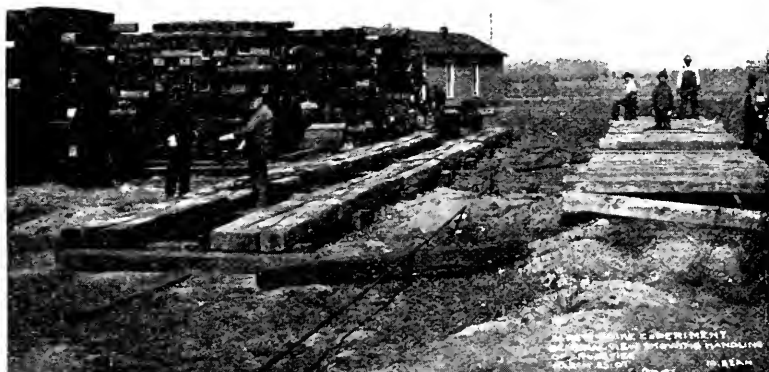
GENERAL VIEW SHOWING HANDLING OF CROSS-TIES.
