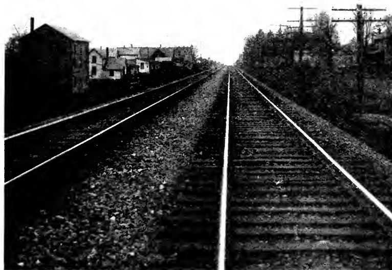
STANDARD BALLAST SECTION, PENNSYLVANIA LINES, EASTERN DIVISION.
