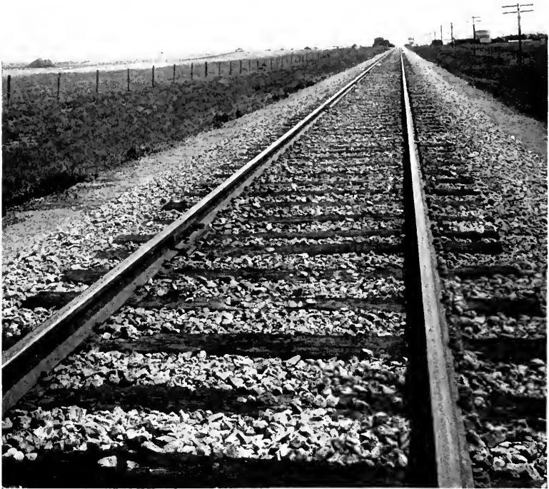
View 19, Western Division. Hewn pine, standard construction screw spike.
