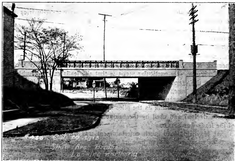
FIG. 25—SHAW AVENUE BRIDGE, EAST CLEVELAND.
