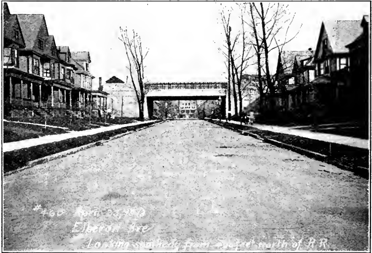
FIG. 39—ELBERON AVENUE, EAST CLEVELAND, AFTER SEPARATION OF GRADES.
