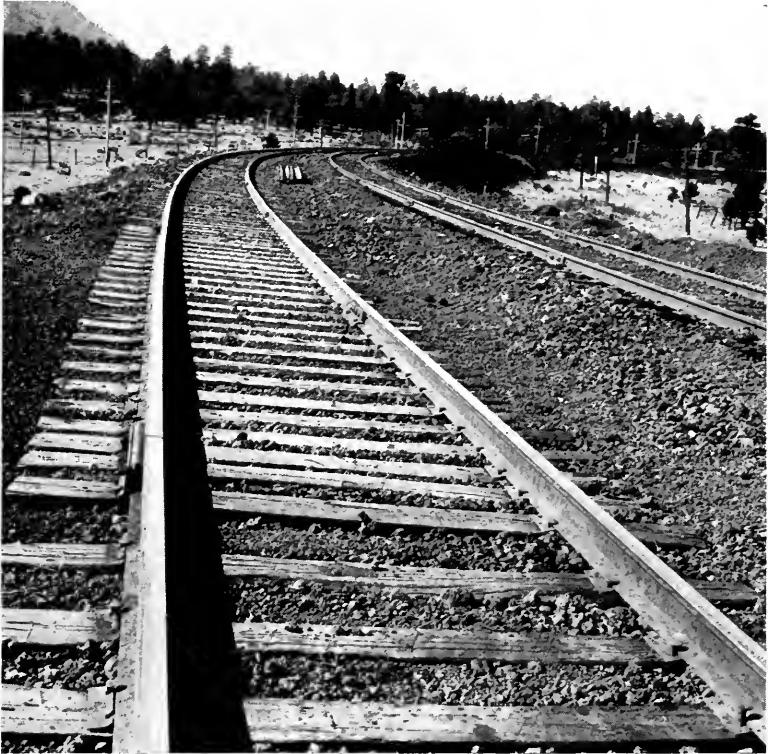
View 1, Albuquerque Division, cut spikes, tie plates, Japanese oak ties. Note the skewing.
