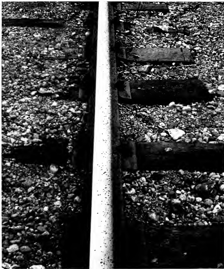
View 19, Illinois Division. Screw spikes inserted with plates without shoulder.
