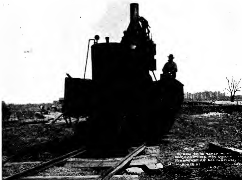
CAR CARRYING AIR COMPRESSOR FOR OPERATING BORING MACHINE.
