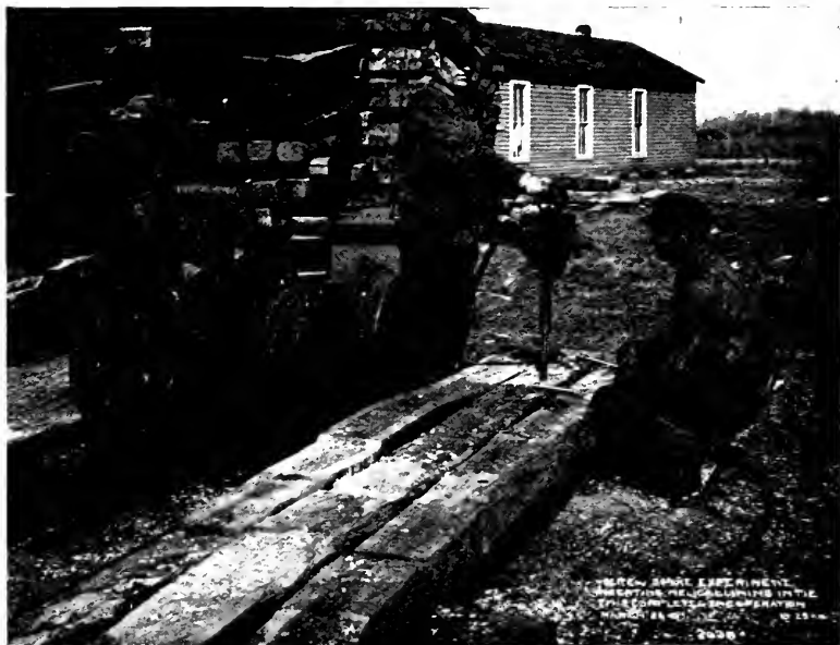
SCREW SPIKE EXPERIMENT. INSERTING THE HELICAL LINING IN TIE. THIS COMPLETES THE OPERATION.
