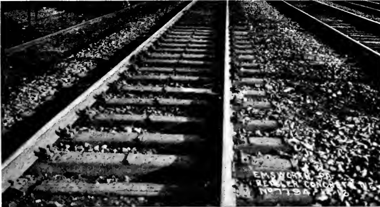
FIG. 16—REIGLER CONCRETE-STEEL TIE, PENNSYLVANIA LINES, EMSWORTH, PA.
