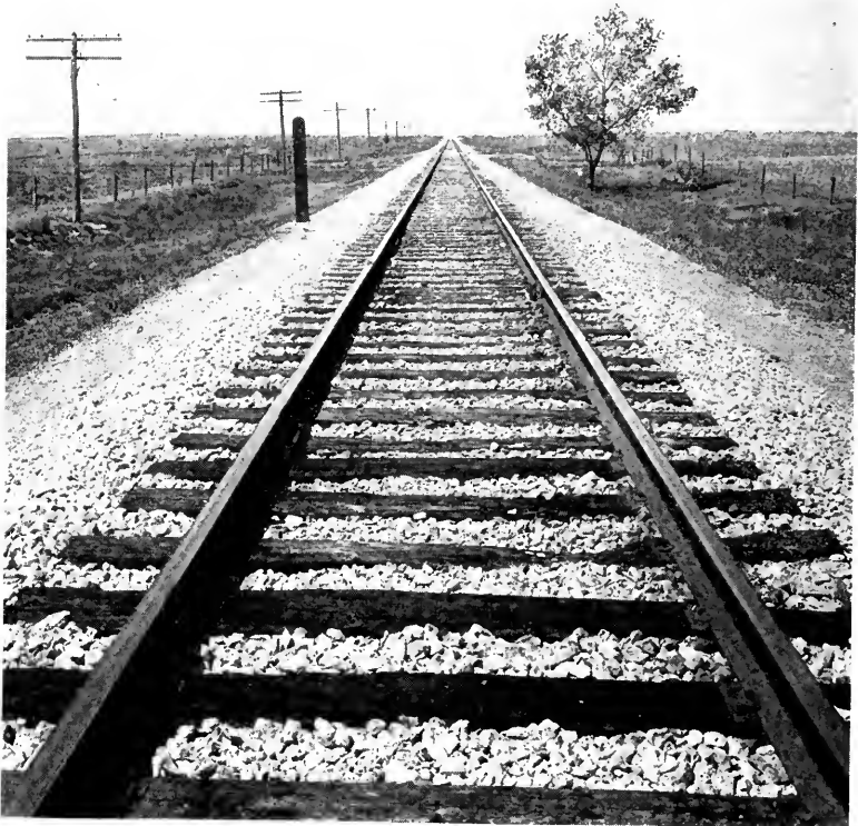
View 24, Western Division. Standard screw spike construction, installed 1910, upon which wreck occurred, account brake beam being down, in 1911.
