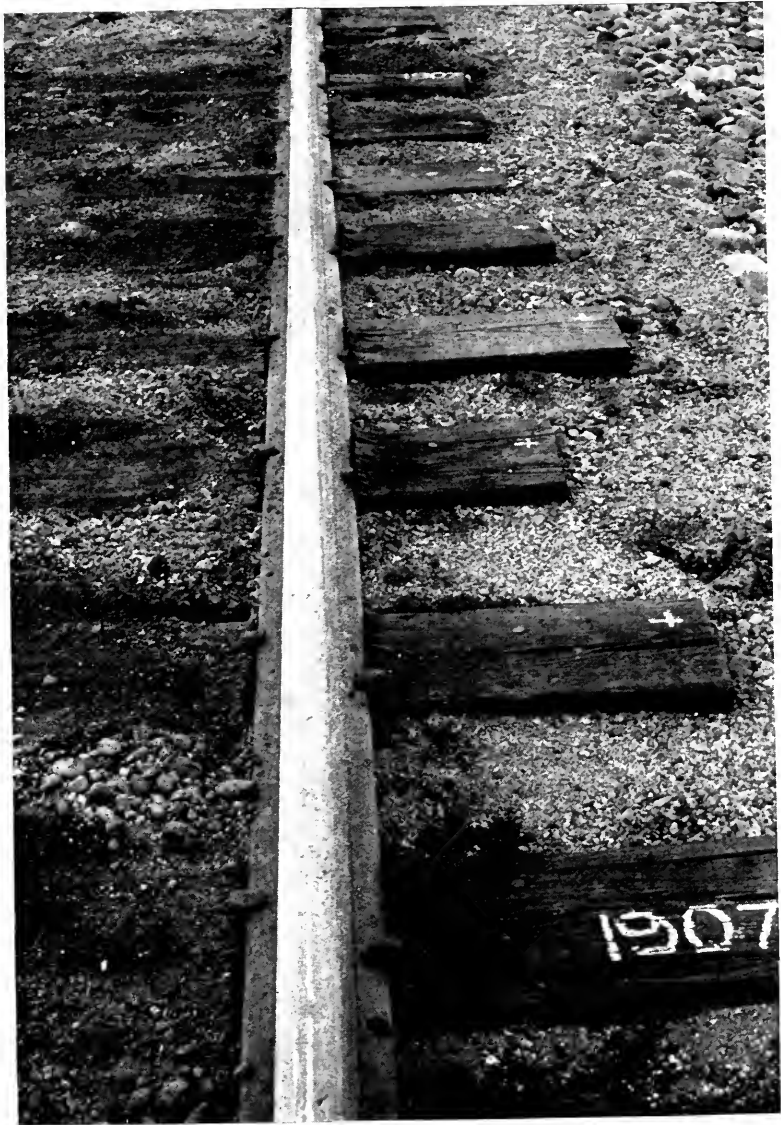
View showing injury to ties by rail cutting and spike driving. View 1, Arkansas River Division, 1907 ties, cut spikes without plates.
