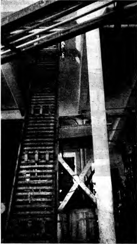
FIG. 4—ELEVATOR, TEXAS CITY TRANSPORTATION COMPANY.
