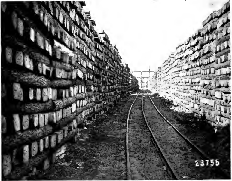
Fig. 2.—Unpeeled Mine Props Closely Ranked and in Contact With Ground.
