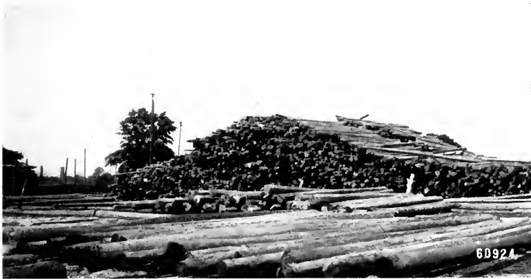
Plate III. Fig. 1.—Wrong Method of Piling Poles for Seasoning.
