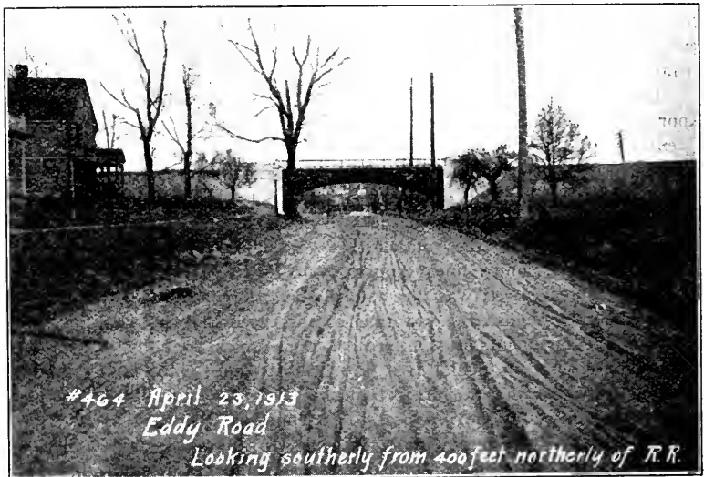
FIG. 41—EDDY ROAD, EAST CLEVELAND, AFTER SEPARATION OF GRADES.
