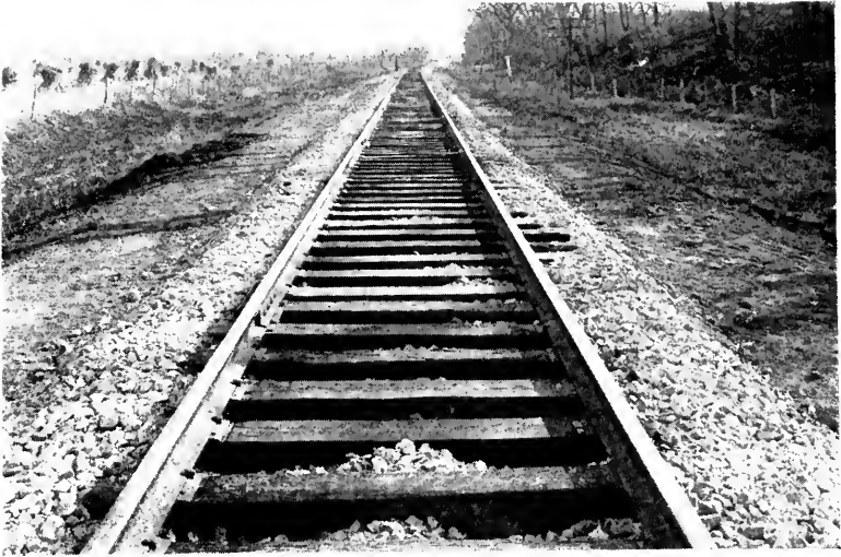
FIG. 21. TRACK SKELETONIZED READY FOR DROPPING BALLAST.
