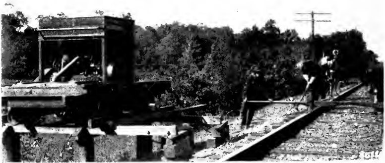
FIG. 12. PNEUMATIC TAMPERS IN OPERATION.
