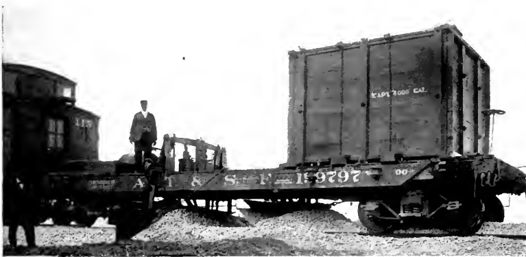
FIG. 20. BALLAST SPREADER AND FORMER IN OPERATION, SHOWING JET OF WATER USED TO SPRINKLE BALLAST AFTER PASSING OVER IT.
