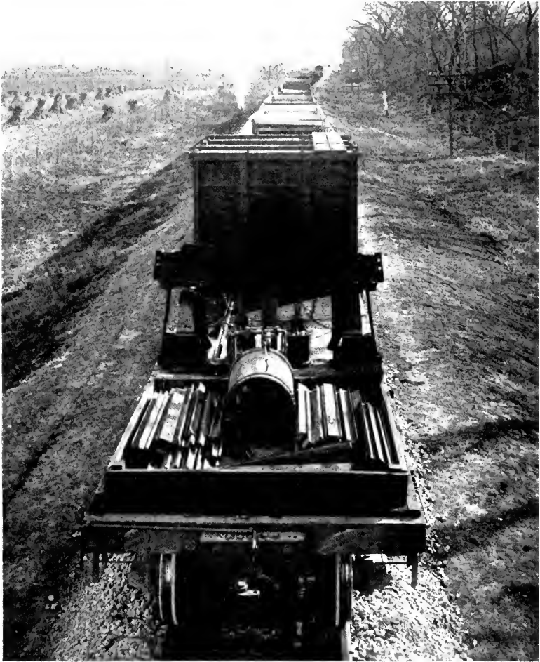
FIG. 18. END VIEW OF BALLAST SPREADER AND FORMER.
