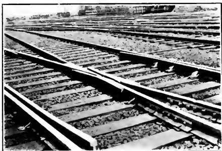
Manganese Steel No. 8 frog, 85-lb. rail. Put in track March 11, 1900. Removed from track April 27, 1904. In service 4 years, 47 days. Maximum life of ordinary frog in same place, three months. Photograph taken April 27, 1904.
