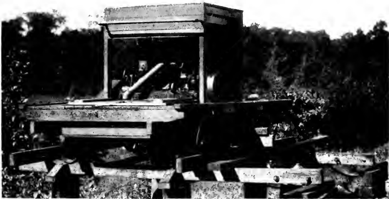
FIG. 10. MOTOR CAR REMOVED FROM MAIN TRACK.
