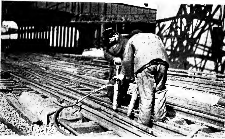
FIG. 13. TAMPING A CROSSOVER IN YARDS.
