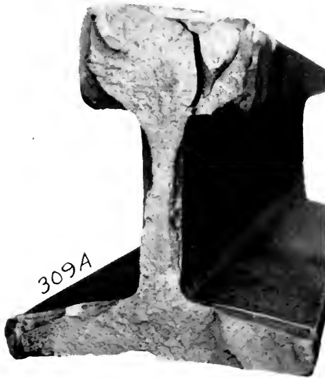
FIG. 309A. SHOWING SPLIT IN HEAD OF RAIL 309, WHICH FAILED DUE TO "FLOW OF METAL."
