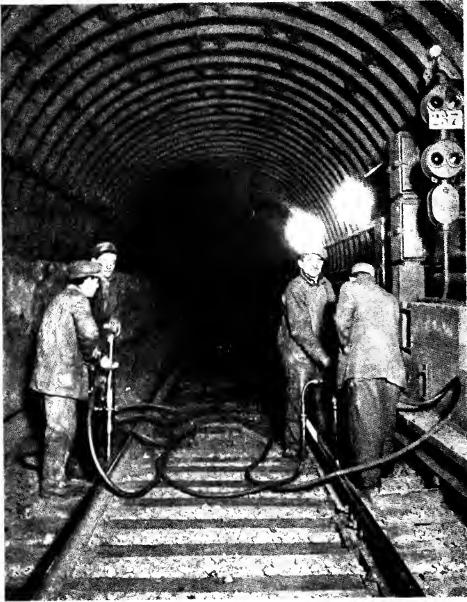
FIG. 14. A NIGHT GANG TAMPING TIES IN THE RIVER TUBES.
