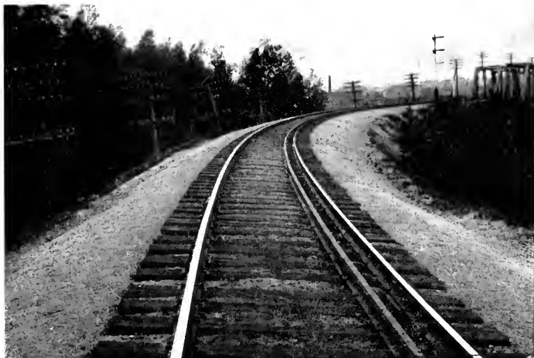
FIG. 62. MAINE CENTRAL RAILROAD. SEVEN-DEGREE CURVE NEAR WATERVILLE, ME. FRICTIONLESS, OR NARROW HEAD RAIL, ON THE INSIDE OF CURVE.
