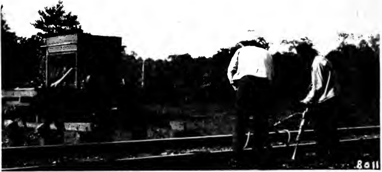
FIG. 11. PNEUMATIC TAMPERS IN OPERATION.
