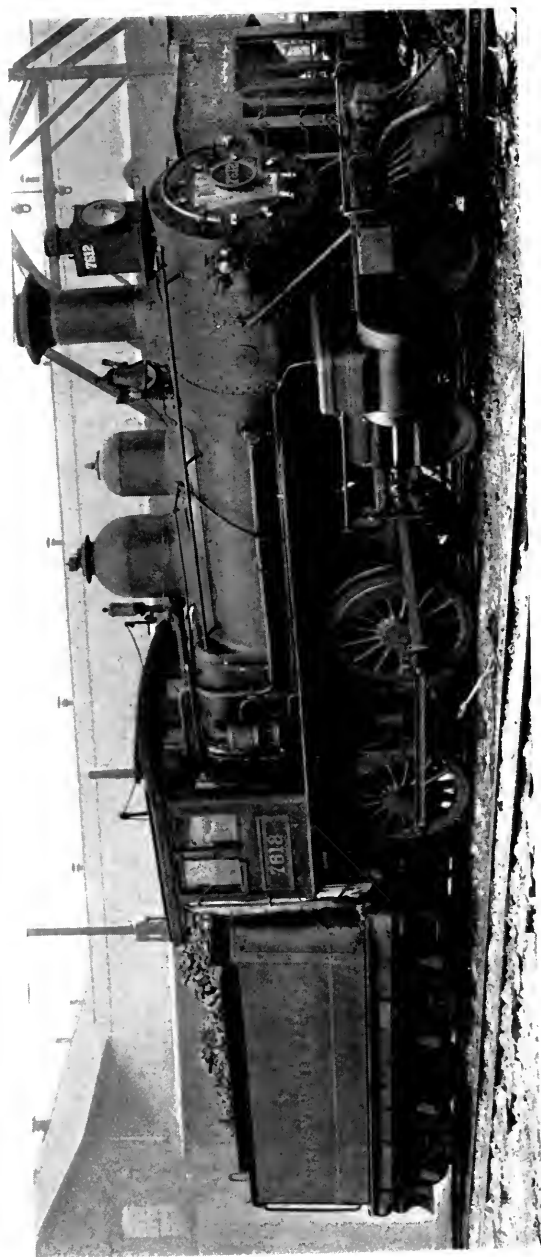
FIG. 5. PENNSYLVANIA LINES WEST OF PITTSBURGH. PASSENGER LOCOMOTIVE, CLASS D-10, TYPE OF THE YEAR 1892. BOILER PRESSURE, 160 LBS. TRACTIVE POWER, 17,060 LBS. TOTAL WEIGHT, INCLUDING TENDER, 183,000 LBS.
