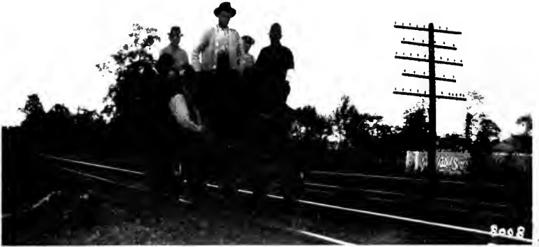
FIG. 8. TRACK GANG RIDING ON MOTOR CAR THAT PRODUCES POWER TO OPERATE MECHANICAL TAMPER.
