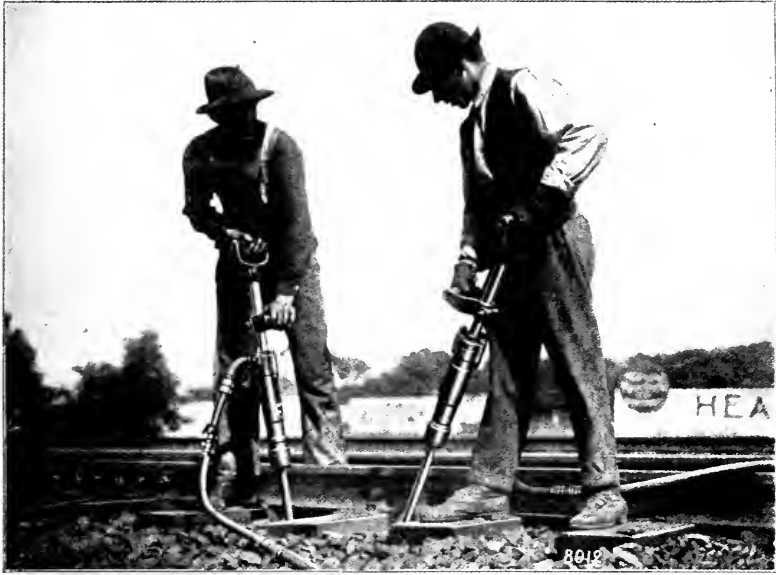
FIG. 5. RESURFACING WITH PNEUMATIC TAMPERS.
