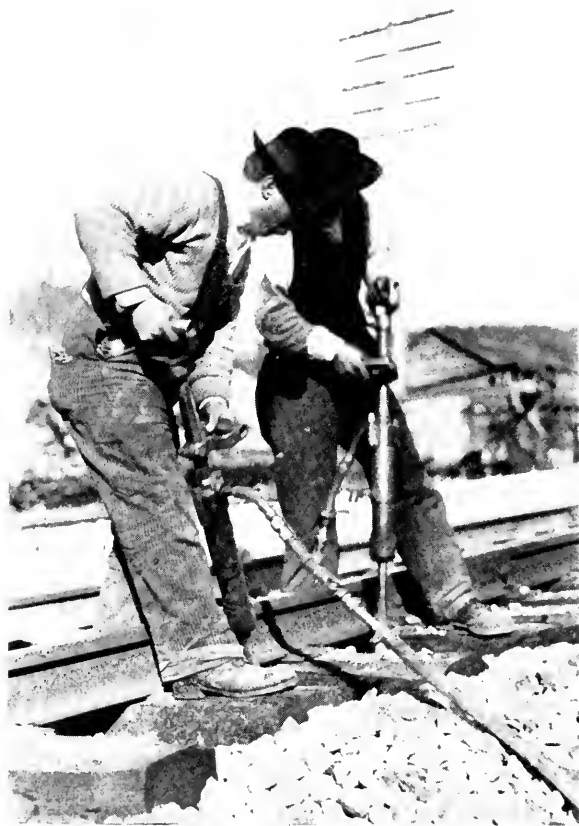
FIG. 4. THE PNEUMATIC TIE TAMPER AT WORK.
