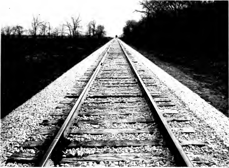
FIG. 23. TRACK SHOWING BALLAST AFTER IT HAS BEEN DRESSED.
