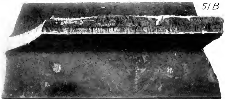
FIG. 51B. SHOWING FLAW IN WEB OF RAIL 51, DARK PORTION SHOWING OLD CRACK.
