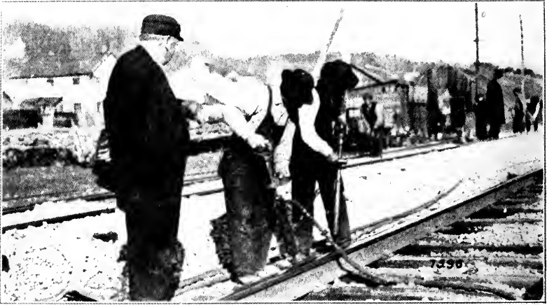
FIG. 7. THE PNEUMATIC TAMPER PERMITS TAMPING IN PLACES MORE OR LESS INACCESSIBLE BY OTHER METHODS.
