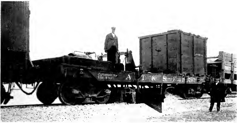
FIG. 19. BALLAST SPREADER AND FORMER IN OPERATION.
