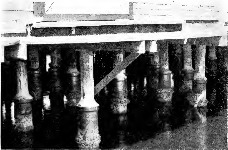
FIG. 2—VITRIFIED PIPE CASINGS.
