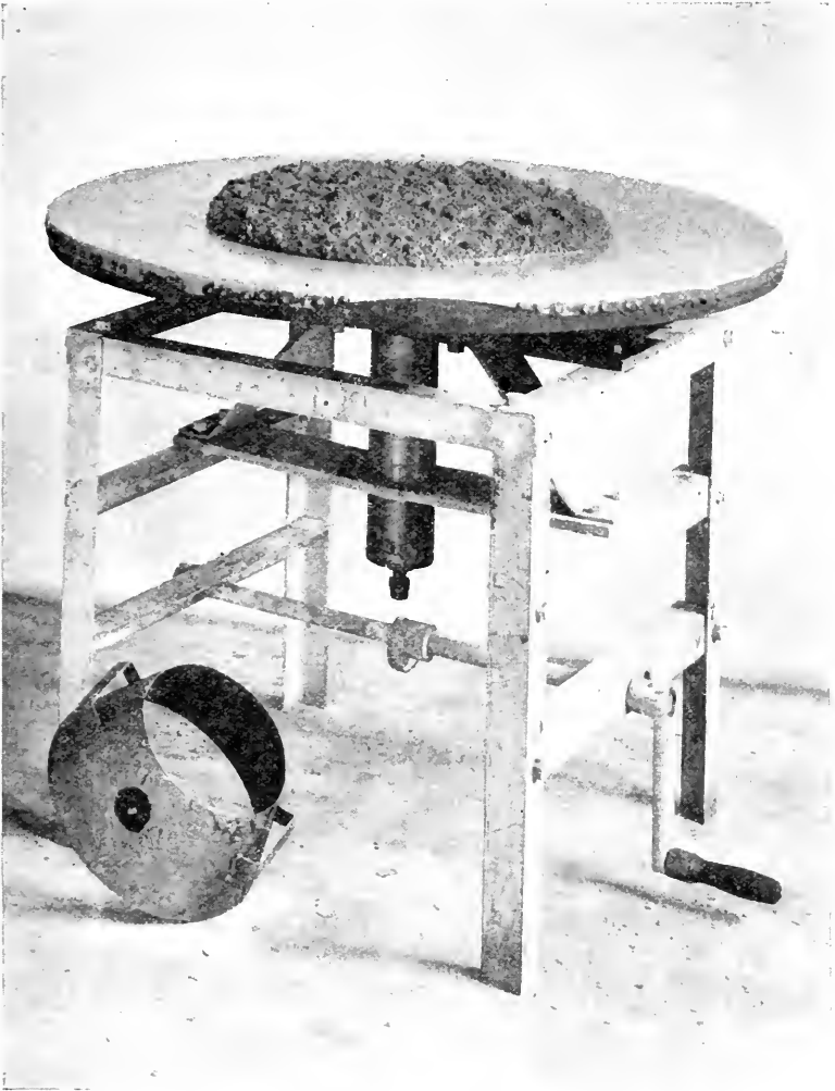
FIG. 8—FLOW-TABLE FOR CONSISTENCY OF CONCRETE.
