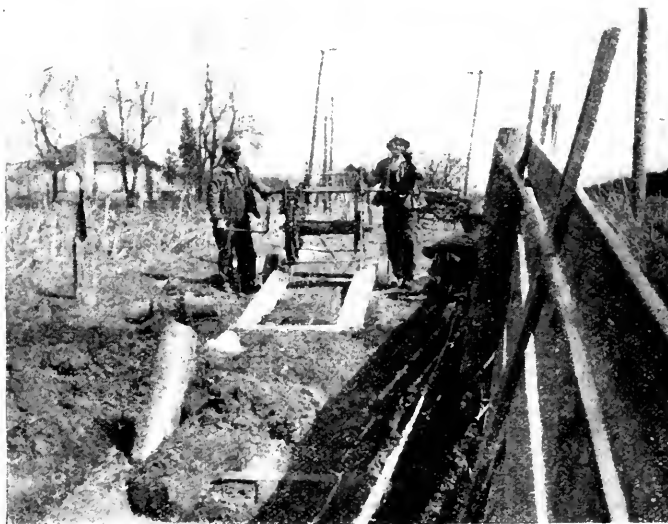
FIG. 9—WINCH FOR PULLING CABLE IN PLACE.
