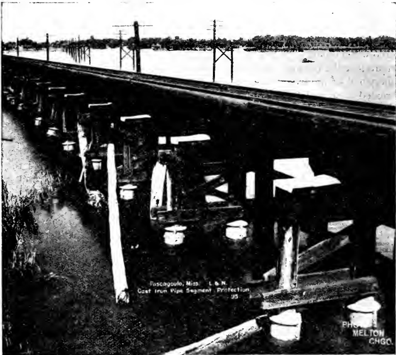
FIG. 1—CAST IRON PROTECTION ON LOUISVILLE & NASHVILLE RAILROAD.
