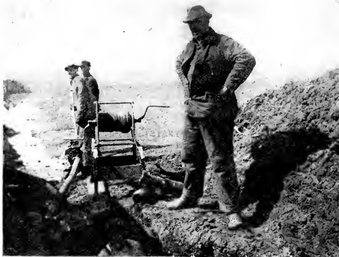
FIG. 12—WINCH AND TRENCH PUMP IN POSITION.
