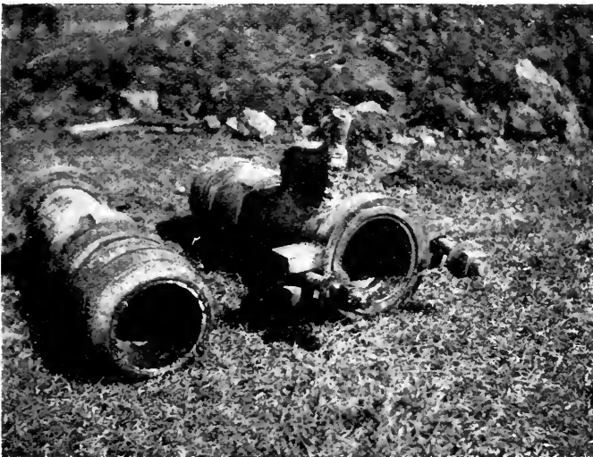
FIG. 11—SPECIAL RISER DEVICE.
