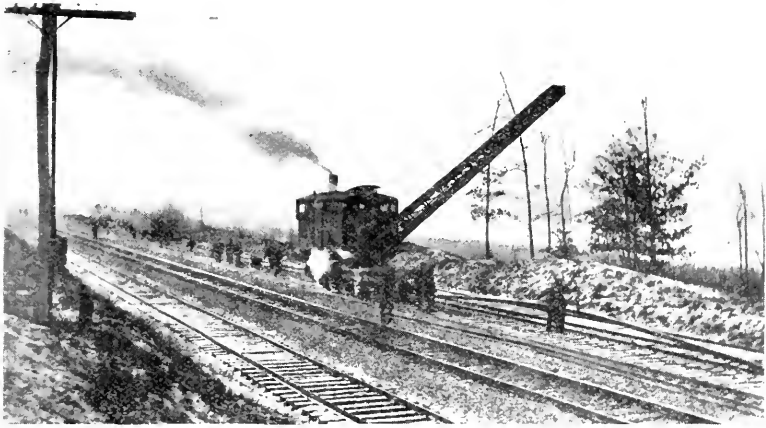
FIG. 1—CRANE THROWING OLD RAIL OUT, AHEAD.
