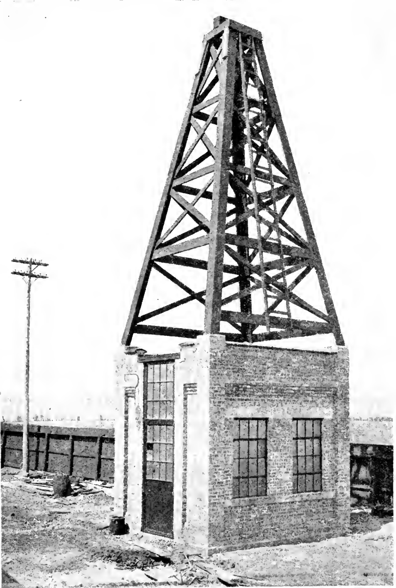
BRICK PUMP-HOUSE AND DERRICK FOR MOTOR-DRIVEN DEEP-WELL CENTRIFUGAL PUMP.
