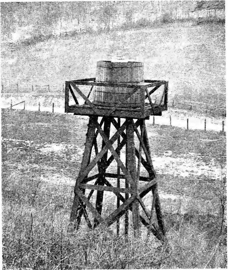
AIR-LIFT DISCHARGING INTO TANK DIRECT FROM UMBRELLA TOP
