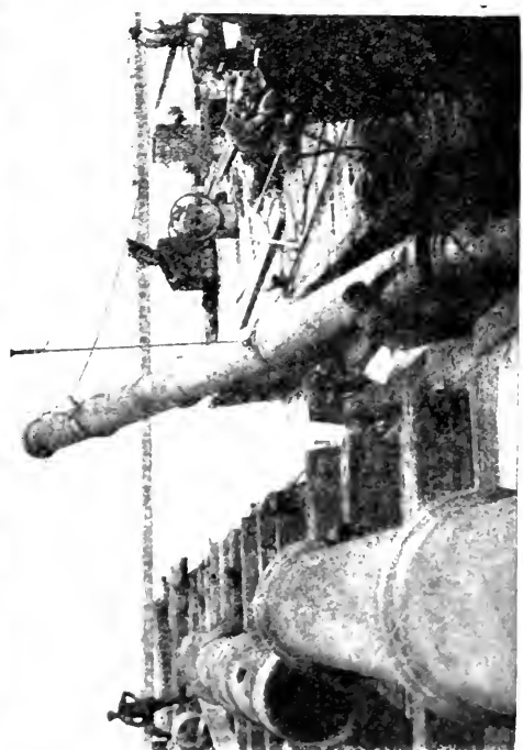
ILLUSTRATING METHOD USED FOR POURING JOINTS ON INTAKE PIPE FOR ILLINOIS CENTRAL RAILROAD, AT 27TH STREET, CHICAGO.
