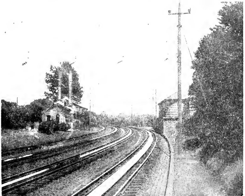
FIG. 4—WATER PANS AT RADNOR, PA., FOUR-TRACK SYSTEM OF PANS ON CURVE
