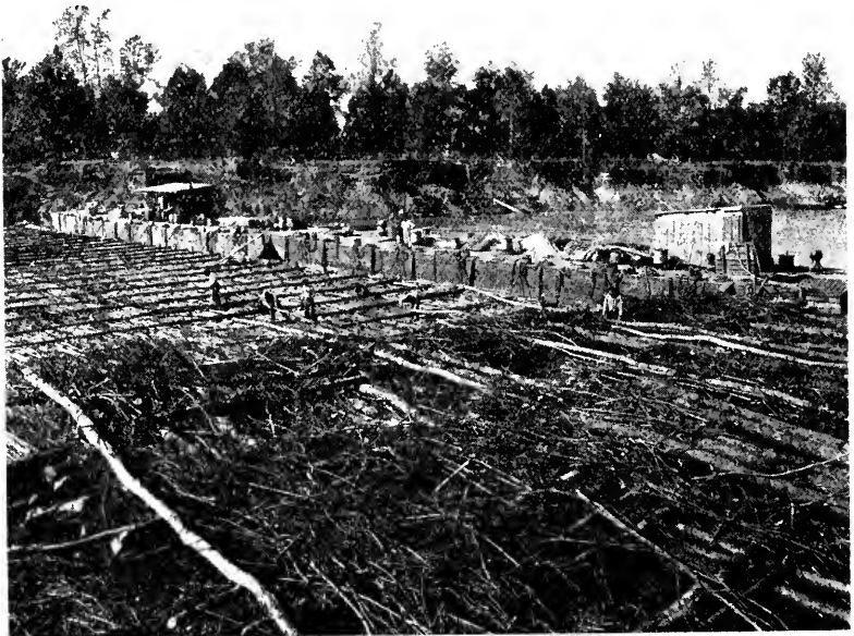
FIG. 2—WILLOW MATTRESS IN POSITION BEFORE SINKING
