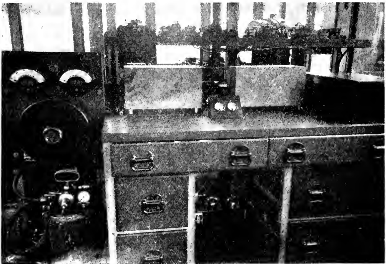
FIG. 5. AMPLIFIER TABLE SHOWING SHIELDED AMPLIFIERS AND RELAYS.
