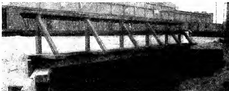
Picture 60. Trestle 9-D, Southern Pacific, at Berkeley, Calif., 12 feet, CSB-4, constructed 1897. Entire bridge is as originally constructed except that the sidewalk has been added. Sidewalk is of untreated fir. Photographed August 7, 1928.
