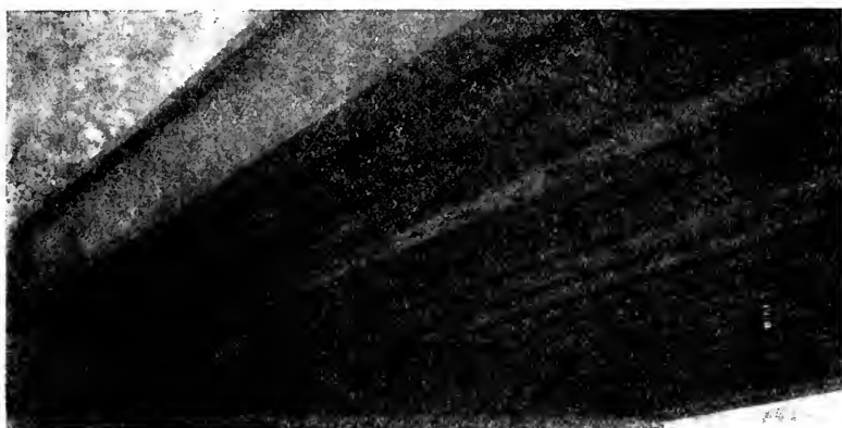
Picture 89. Bridge 513-K, Southern Pacific, Genesha Park, Pomona, Calif. This bridge has two 17-foot spans, each with 21 7 x 16—18 creosoted fir stringers which have been in service since 1896. All in excellent condition. Photographed August 9, 1928.
