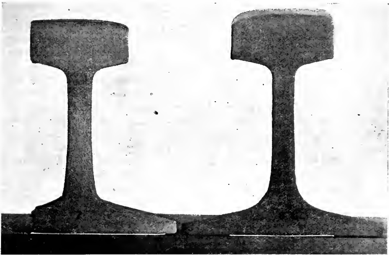
RAILS BUILT UP BY OXY-ACETYLENE WELDING PROCESS
