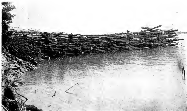
FIG. 6—SHORE PROTECTION MISSOURI RIVER—ILLINOIS CENTRAL SYSTEM— RETARD No. 1
