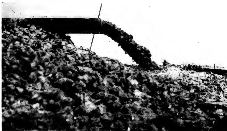
FIG. 10—HYDRAULIC FILL SHOWING ANGLE OF SLOPE
