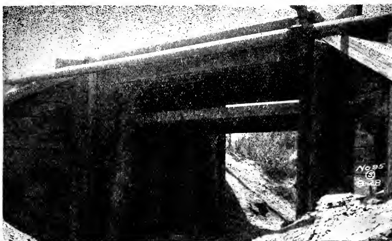
Picture 95. Bridge 460-A, Southern Pacific, east of Sylmar. Length 15 feet, constructed of creosoted Douglas fir 1897. No replacements of original timbers made. Creosoted timber spreaders put in in recent years. All timbers in excellent condition. Photographed August 10, 1928.
