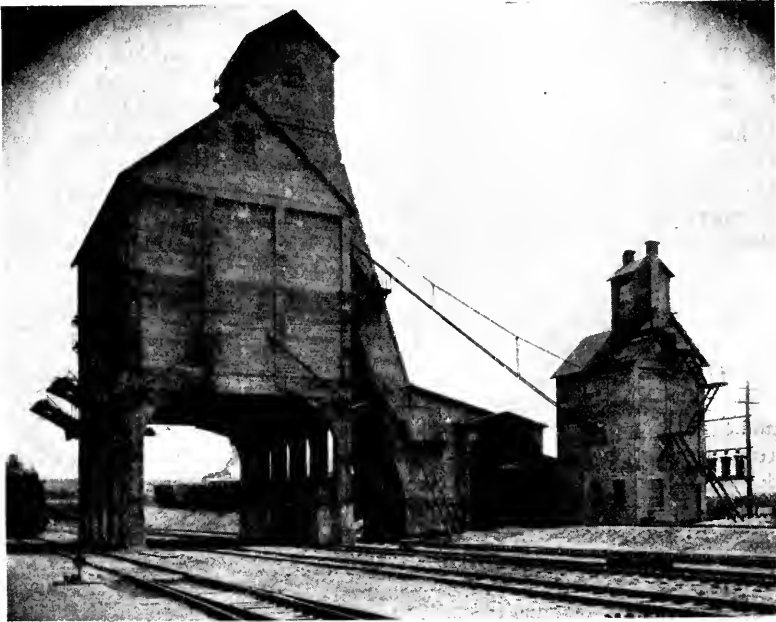
COALING STATION WITH INDEPENDENT SANDING FACILITIES, CHESAPEAKE & OHIO RAILWAY
