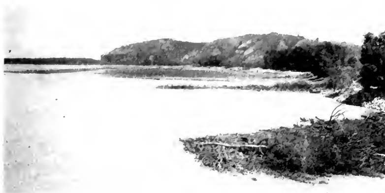
FIG. 8—SHORE PROTECTION MISSOURI RIVER—ILLINOIS CENTRAL SYSTEM. RETARDS No. 6-7-8-9-10 AND 14
