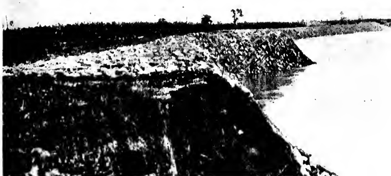
FIG. 4—BRUSH MATTRESS IN WIRE ENVELOPE APPLIED TO CAVING BANK
