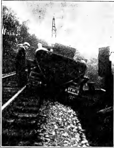
TRACK TYPE TRACTOR PASSING BY A SIGNAL AND OVER THE CONDUIT.
