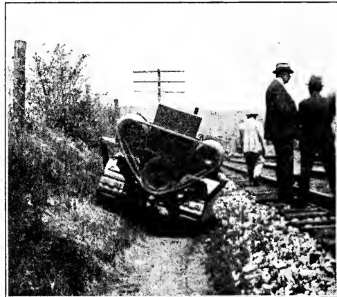
SHOWING TRACK TYPE TRACTOR OPERATING AT A 45 DEGREE ANGLE.
