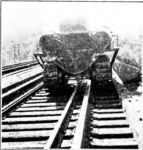
TRACK TYPE TRACTOR MOVING OVER AN OPEN DECK TRESTLE.
