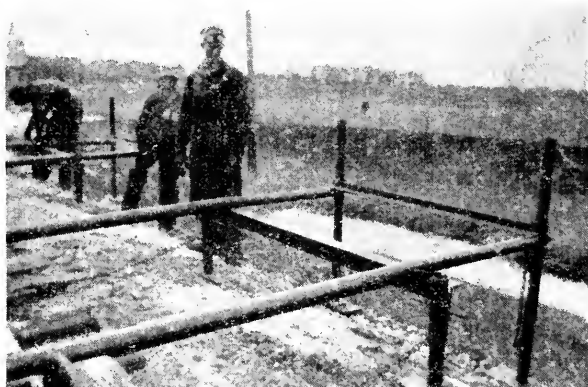
Fig. 12.—Track-Mounted Quick Take-off Set Up on Shoulder.
