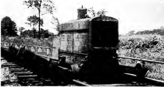
Fig. 4.—Track-Mounted Power Unit.
