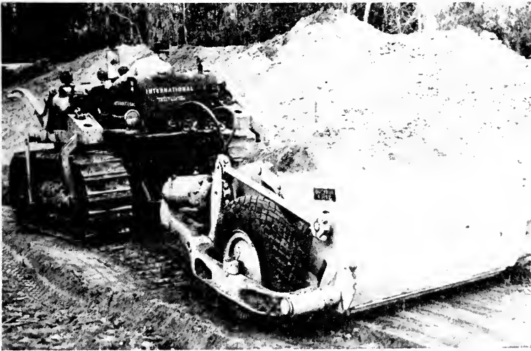
Two-Wheel Scraper—Capacity 4 Cu. Yd., Loading.
