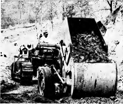
Two-Wheel Scraper — Capacity 4 Cu. Yd., Un- loading Position.
