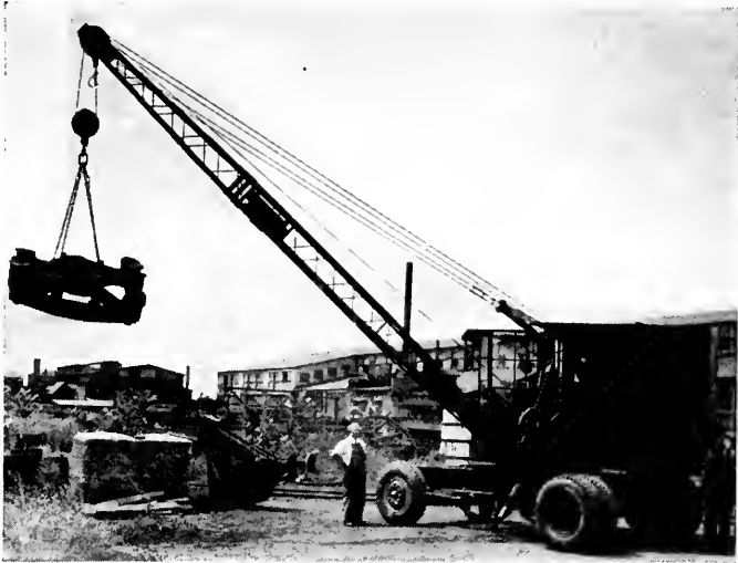
Crane Mounted on Pneumatic Tired Truck Frame.
