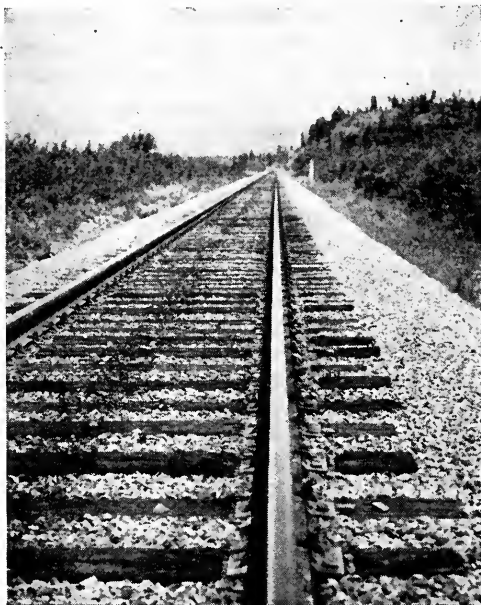
View of the Welded Rail on the Great Northern at Rexford
