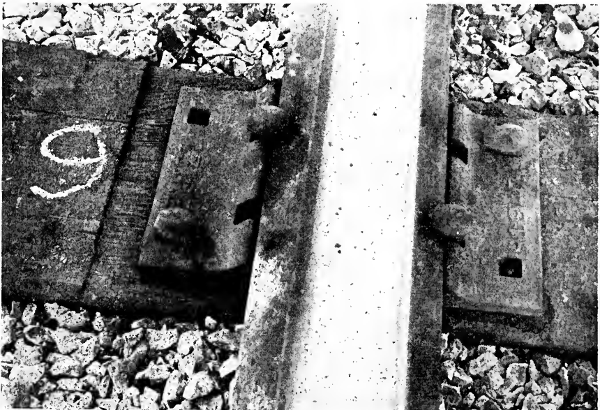
Fig. 10.—Section 9, Two each of Standard Cut Spikes for Line and Anchors.
