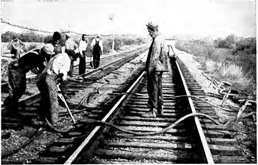
Fig. 5.—Grouting in Area of Pressure Cell Installation.
