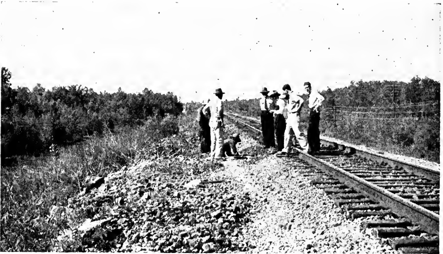
Fig. 6.—Soft Track Across Reservoir Area. Illinois Central Railroad, Coldwater, Miss.
