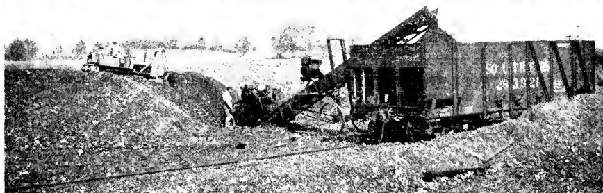
Fig. 2.—Views Showing Loading and Unloading Operations.
