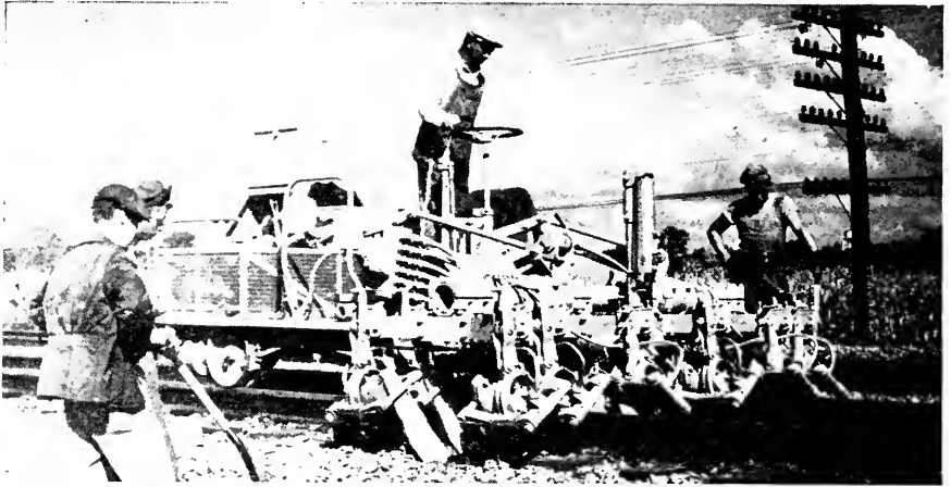
Fig. 1.—The Electric Vibratory Ballaster.
