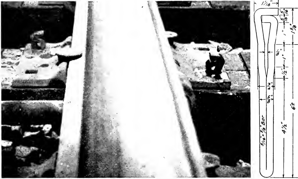
Fig. 15.—Section 13. Tie Plate Lock Spike on the North 12 Ties of the Elastic Spike Section on the Curve.
