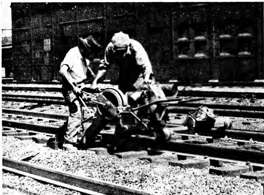
Fig. 1.—Power Bolt Tightener.
