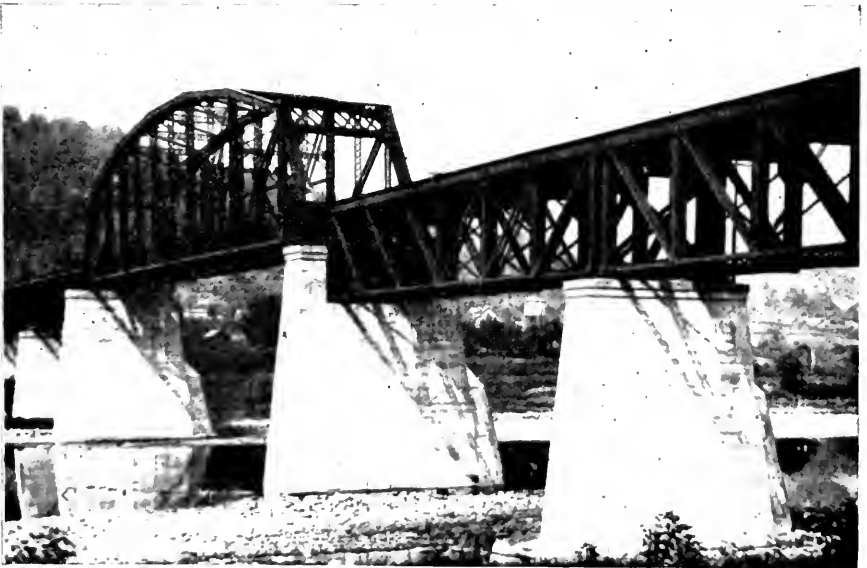
Fig. 4.—Piers Restored by Applying Shotcrete.
