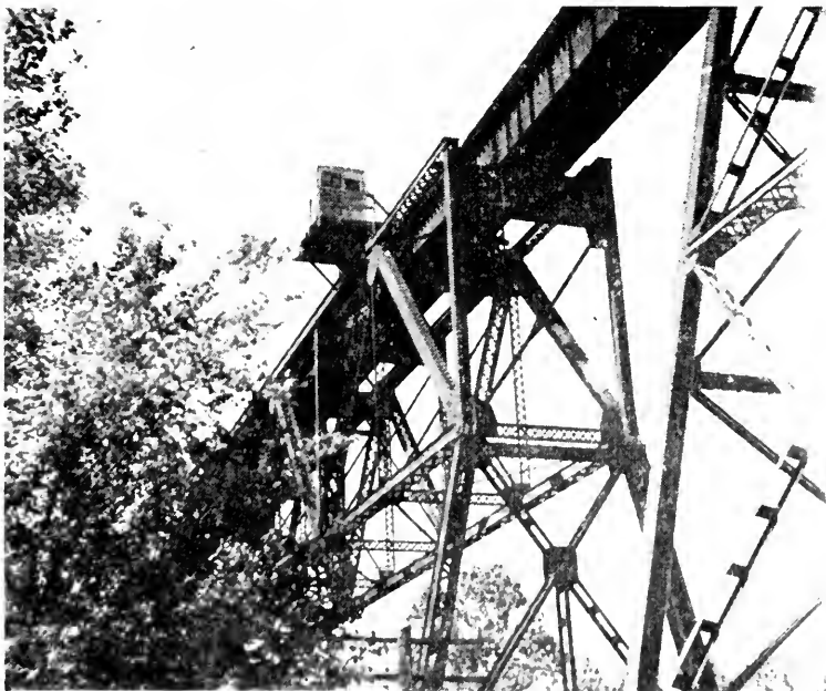
Fig. 3.—Location of the Test Building.
