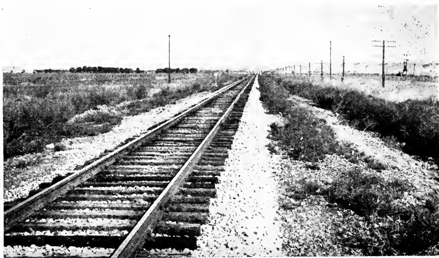
Fig. 12.—Regouted Track on the Northern Pacific in Eastern Montana.
