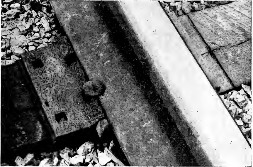
Fig. 21.—Section 21. Fabco Track Pad.
