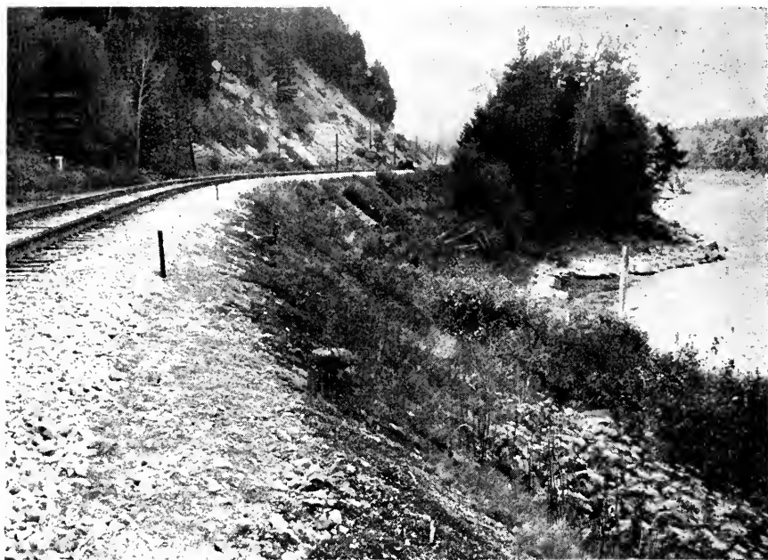
Fig. 16.—Fill Stabilized by Piling. Northern Pacific, Noxon, Mont.
