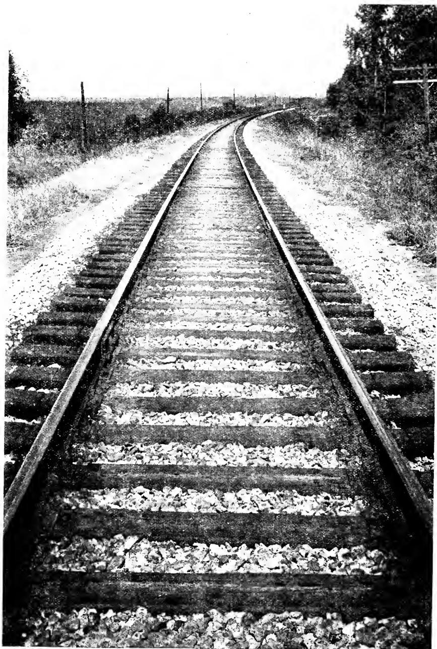
Fig. 12.—Vapor-Dried Ties After Five Years.
