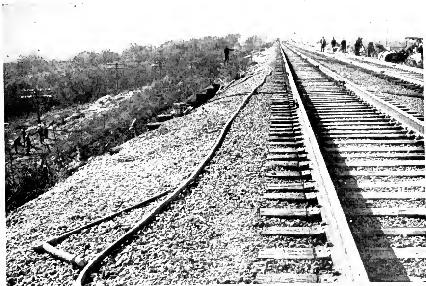
Fig. 9.—Grouting Sliding Fill. Burlington, Red Oak, Iowa.
