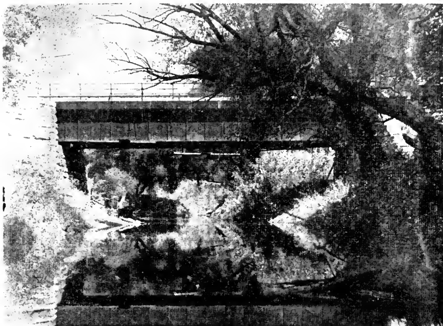
Fig. 5. General view of 78-ft. deck girder span near Morrison, Ill.
