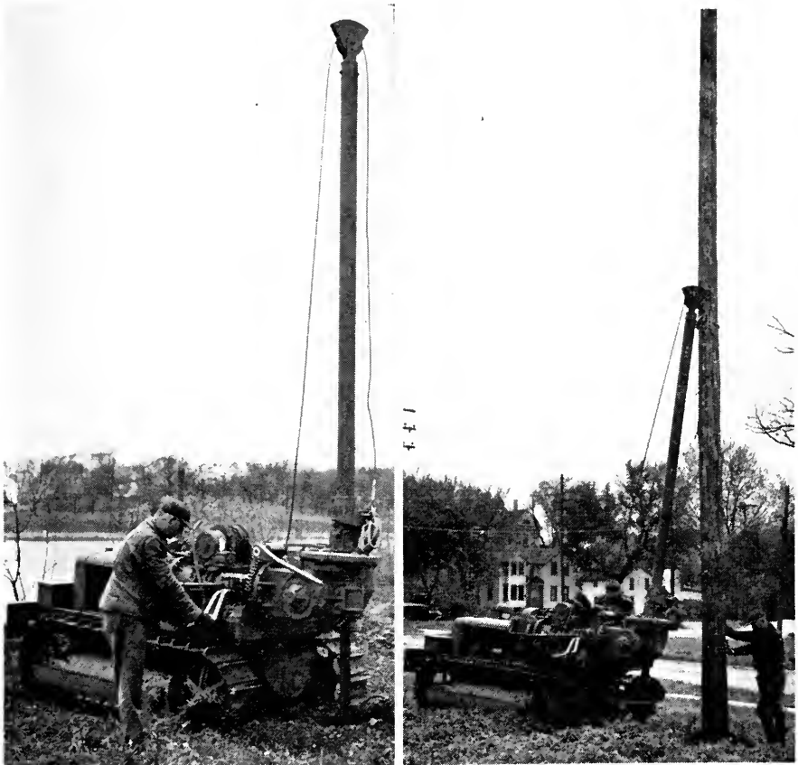
Fig. 1. (left above) Earth boring machine digging hole.
