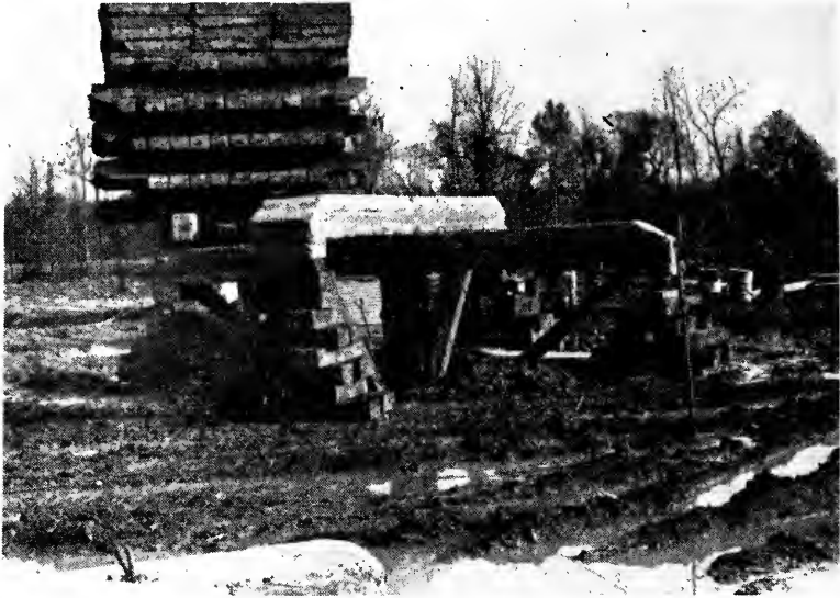
Fig. 10. Method of carrying load on single piles.
