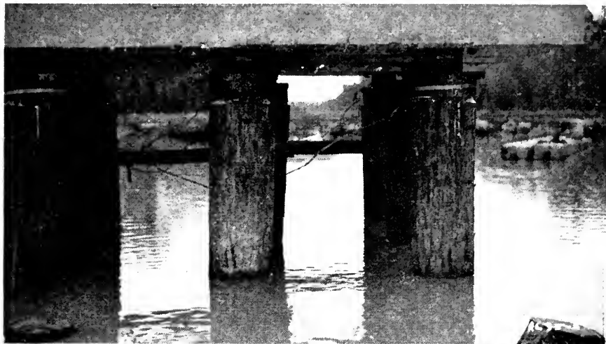
Fig. 11. Timber pile group at Half Moon Bayou.
