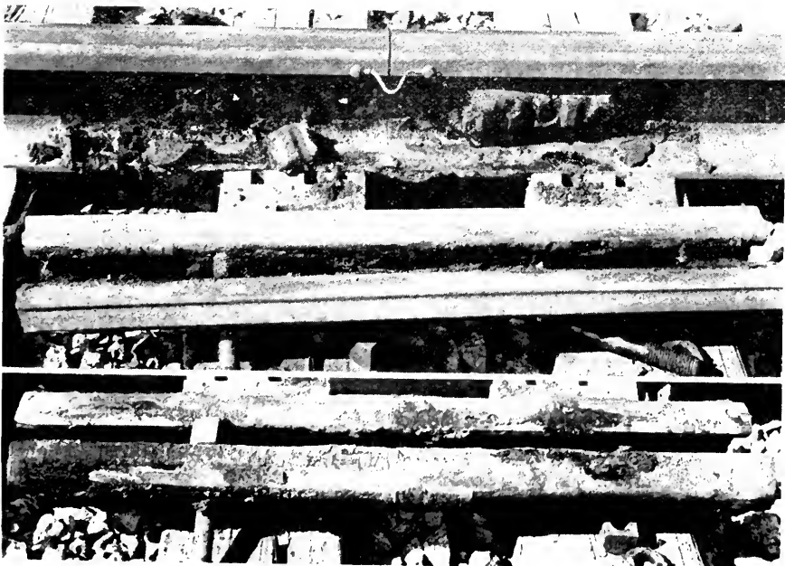
Fig. 6. R. M. C. plastic joint packing.
