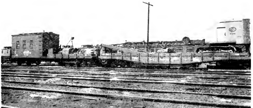
Fig. 3. Half flat—half box, and crane-carrying flat car.
