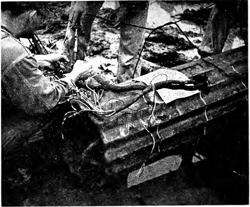
Fig. 13. Butt end of pile, showing leads from recording instruments being connected to leads from wire gages.
