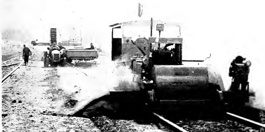
Fig. 3. The track cleaning machine in action. Note windrows of debris plowed outward from the rails.
