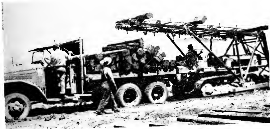
Fig. 6. Tie loading attachment loading ties on truck direct from roadbed.
