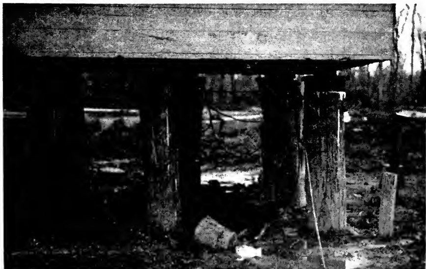
Fig. 12. Timber pile group at Two O'Clock Bayou.
