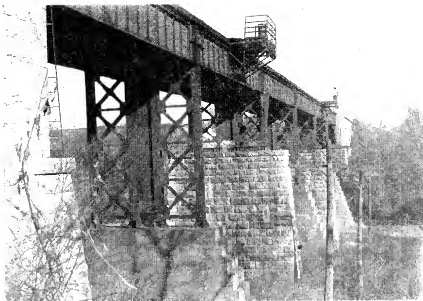
Fig. 1. General views of 70-ft. \frac{1}{4} -in. girder viaduct near Jefferson, Iowa.
