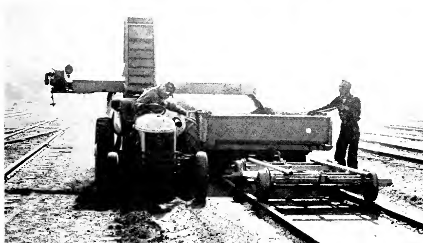
Fig. 4. The tractor-mounted loader, picking up the windrowed debris and loading it into hydraulic dump boxes.
