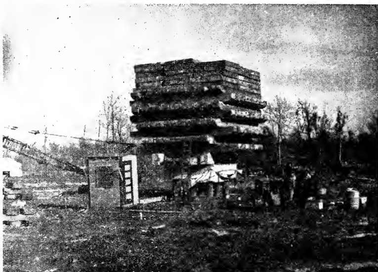
Fig. 14. Loading the steel pile group with 1,183,000 lb. of concrete blocks.
