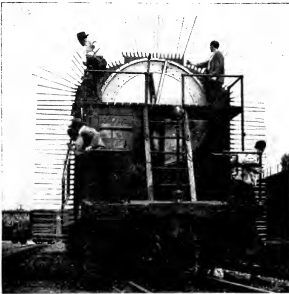
View showing outside pantograph with feelers in position to register outline of a fixed structure—New York Central clearance car.
