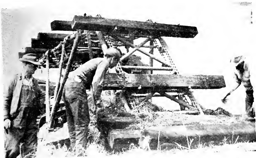
Fig. 5. Tie loading attachment lifting ties from roadbed for sorting and loading.
