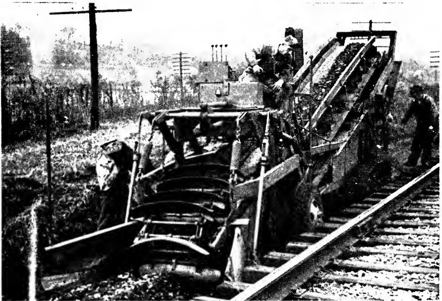
Fig. 9. Crawler mounted, off-track ballast cleaner.
