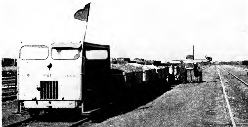
Fig. 1. Beginning in 1943 motor-car-hauled hydraulic dump-box trains were used to dispose of the yard debris.
