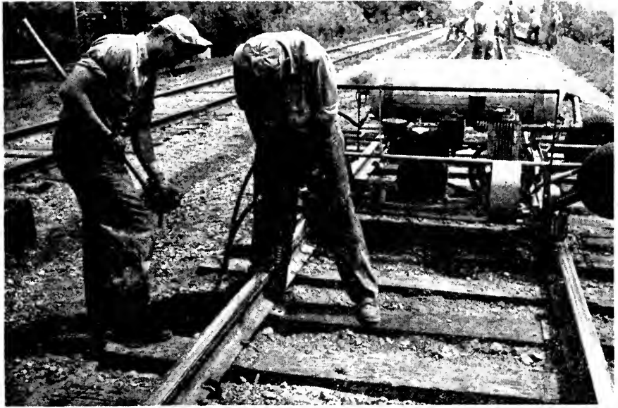
Fig. 8—Pneumatic spike-driving unit.
