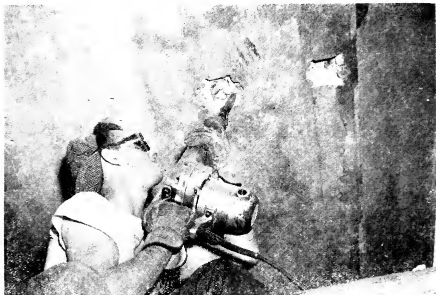
Fig. 5—Cutting out concrete covering on reinforcing bars.
