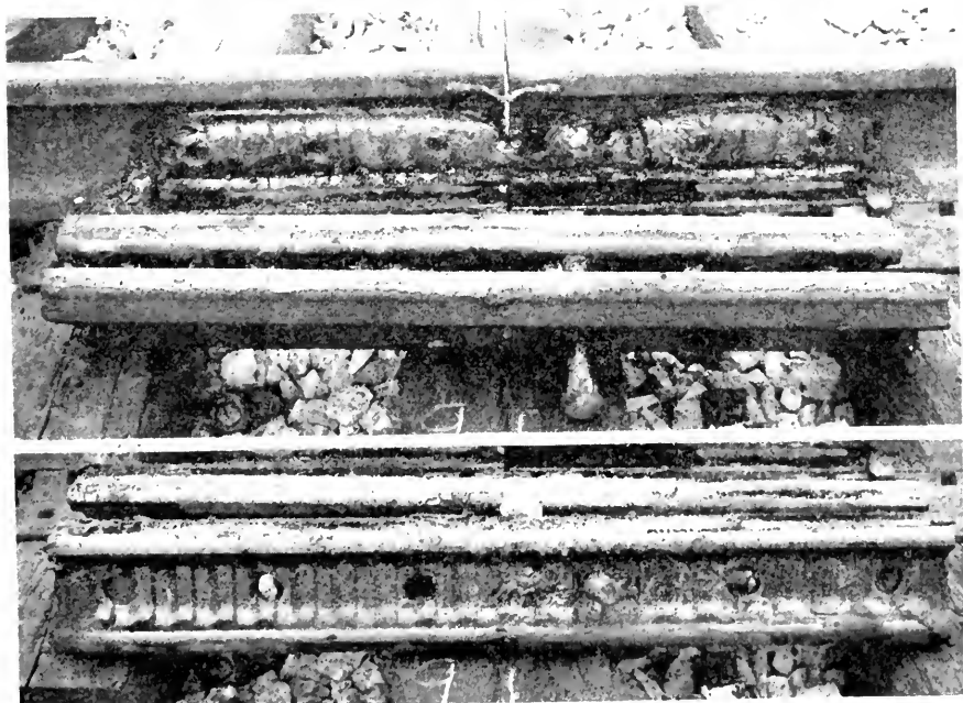
Fig. 6. South Portion Section 1, R.M.C. Plastic Joint Packing (new formula).
