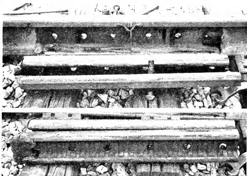
Fig. 21. Both sections of Section 5, 16 lubrication plastic tubes, both ends.
