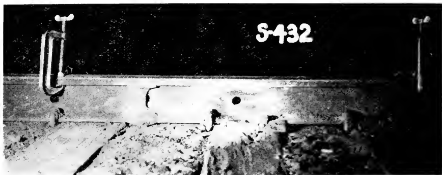
Fig. 3—The 112 RE rail laid in the tunnel in 1938 was welded by the Thermit method, which required one bolt hole in each rail length for welding clamping purposes. After only two years stress corrosion cracks showed up in the web of the rail at these bolt holes, as shown here.
