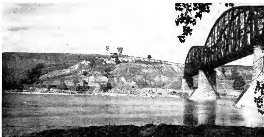
Fig. 9—General view of Bismarck slide.
