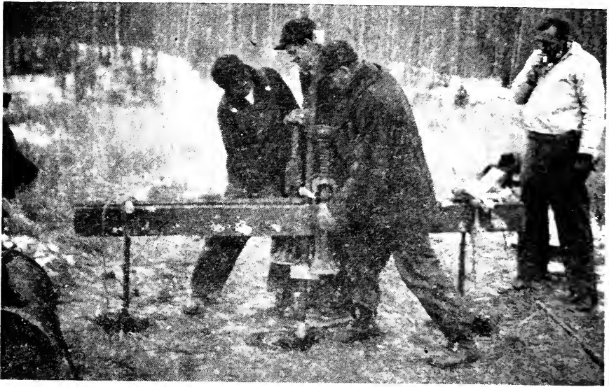
Fig. 5—Jacking vane auger and its casing into the ground.
