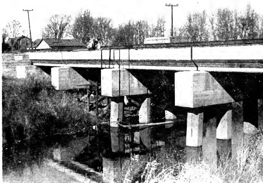
Fig. 1—General views of reinforced concrete pile trestle near Adams, Wis.
