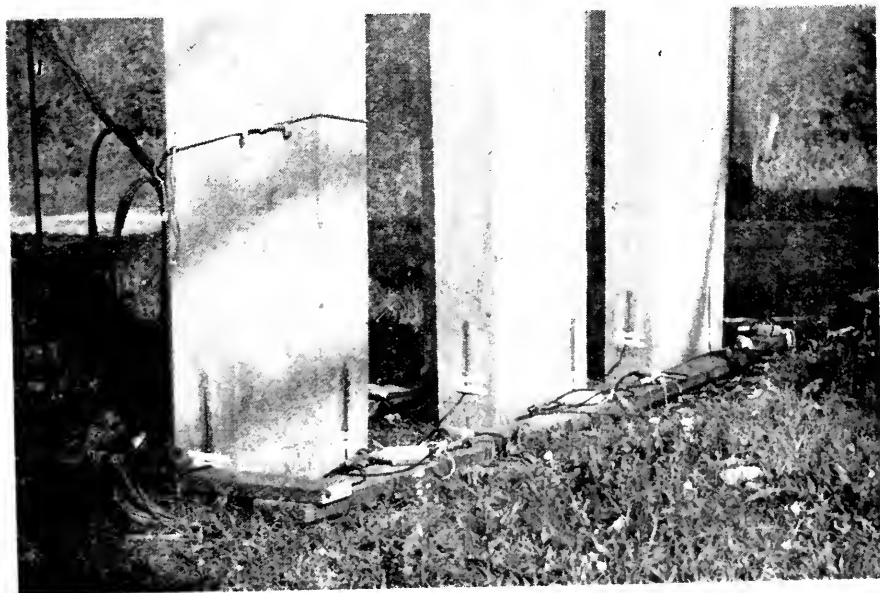
Fig. 10—Location of SR4 wire gages on piles.
