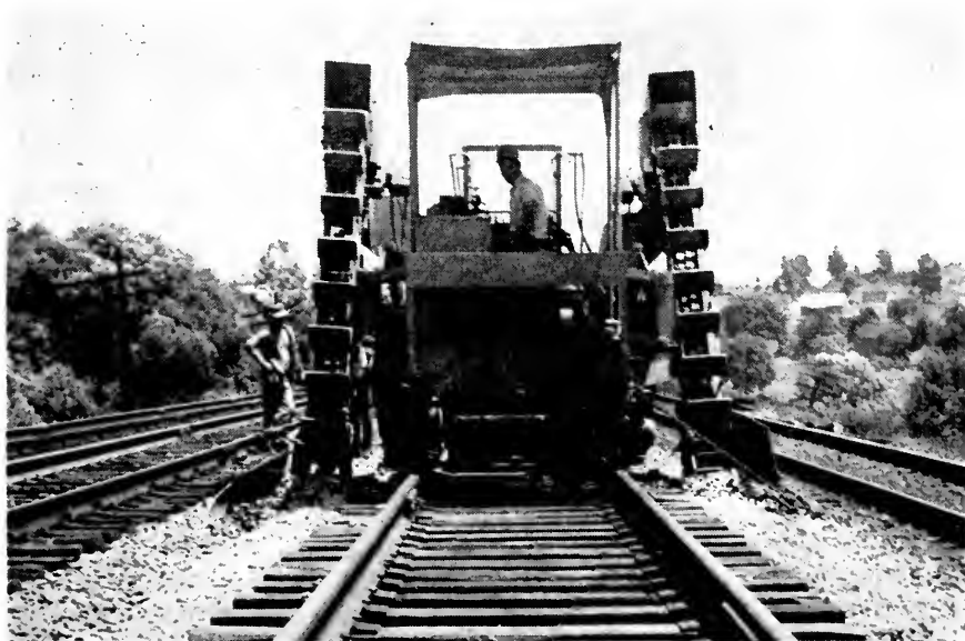
Fig. 2—Bucket-conveyor ballast distributor.
