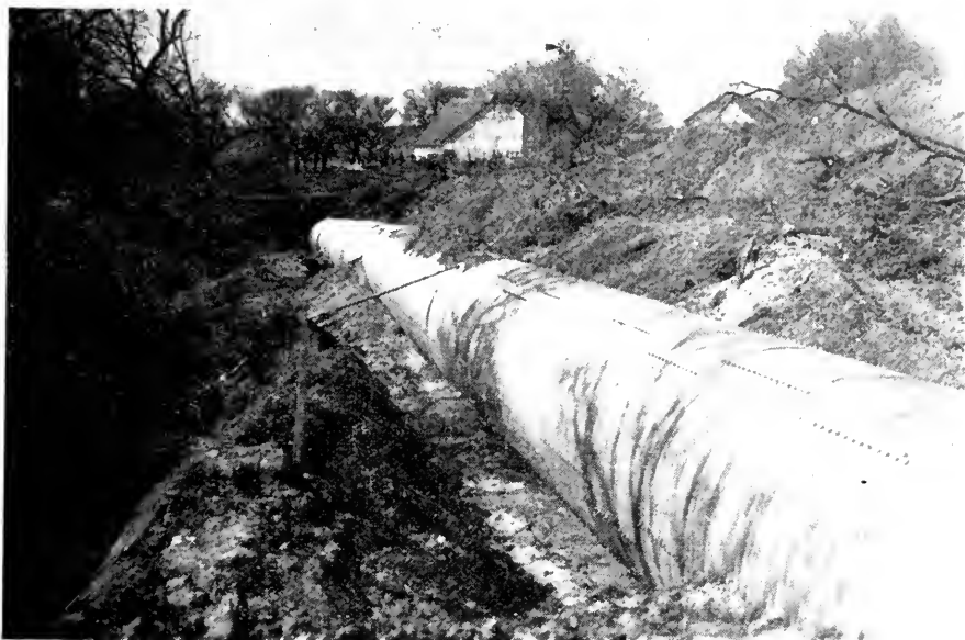
Fig. 1—Poor backfilling.
