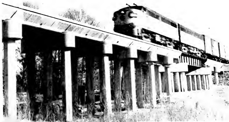
Fig. 7—General views of reinforced concrete pile trestle near Rochelle, La.
