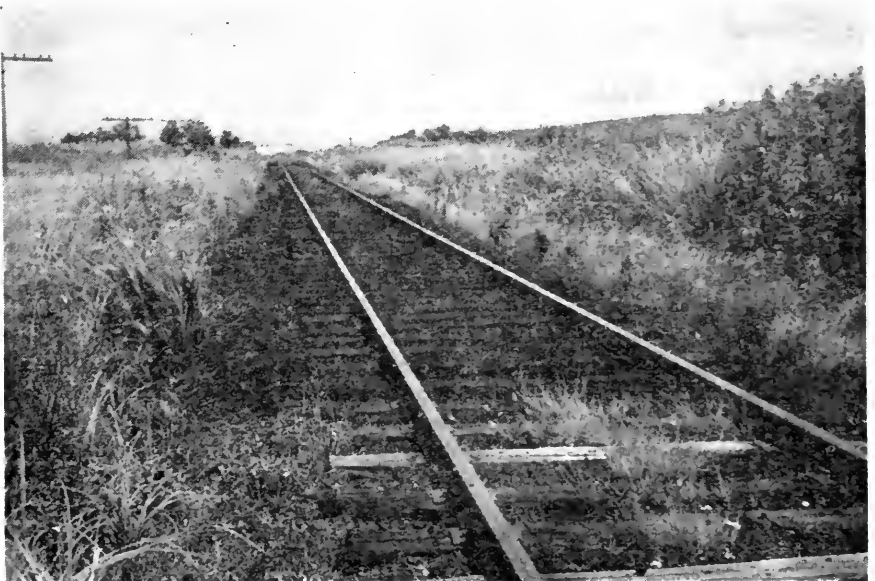
Fig. 2—The heavier aromatic oils will control annual weeds and retard perennials. One to three treatments at a chemical cost of $12 per mile each will be required. These treatments are safe, easily applied, and are recommended for many roadbed conditions.
