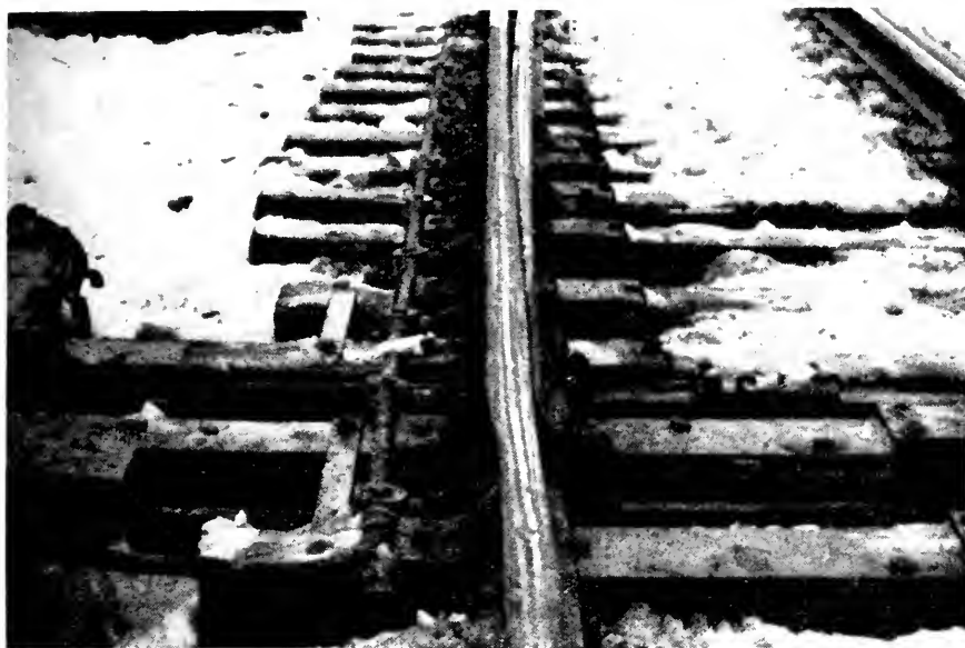
Fig. 3—Electric heater with timing device, showing conduit connections.
