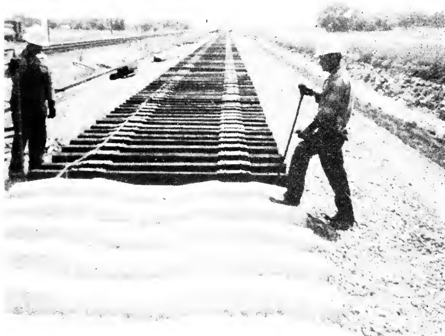
Looking west from concrete tie section No. 8 to Section No. 9 which is built with wood ties according to Santa Fe standards.
