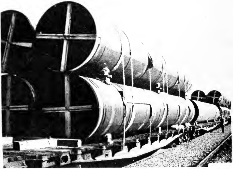
Pipe loads on 54-ft flat cars.
