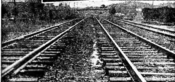
Cross-Section showing little or poor drainage before Ballast Cleaning.
