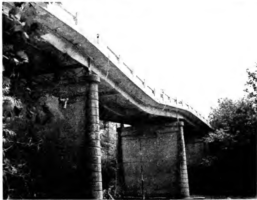
Fig. 11—Photographs illustrating mode of failure of Bridge 4.
