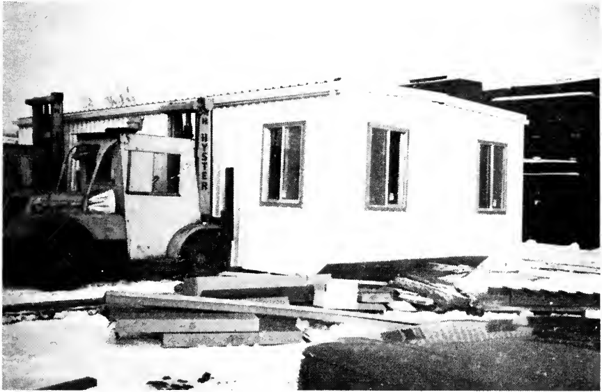
Typical small section building (12 ft wide) ready to load on flat car.
