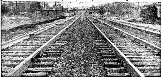
Cross-Section showing little or poor drainage before Ballast Cleaning.
