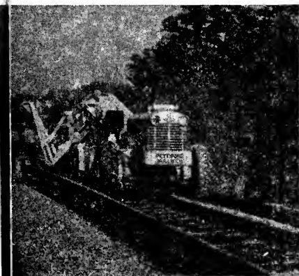
LAYING WELDED RAIL
