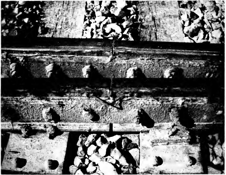
Fig. 4—Two non-insulated 36 in. adhesive-bonded joints applied to 132-lb rail. This installation was made in track to existing rail ends and adjacent to a frog.
