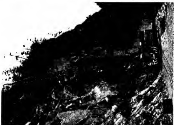
(b) Scaling a very high slope from a platform held by a long crane
