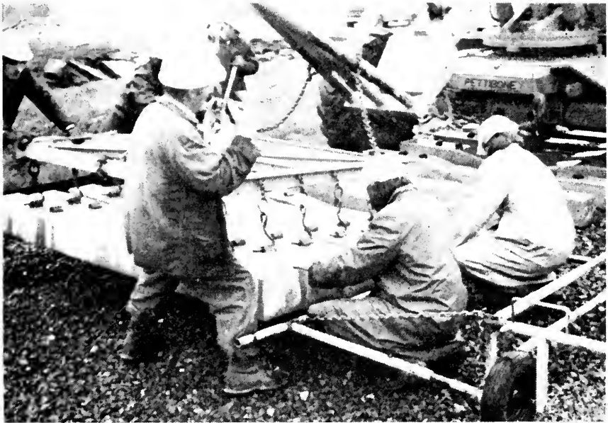
Fig. 7—Distributing and spacing concrete crossies.
