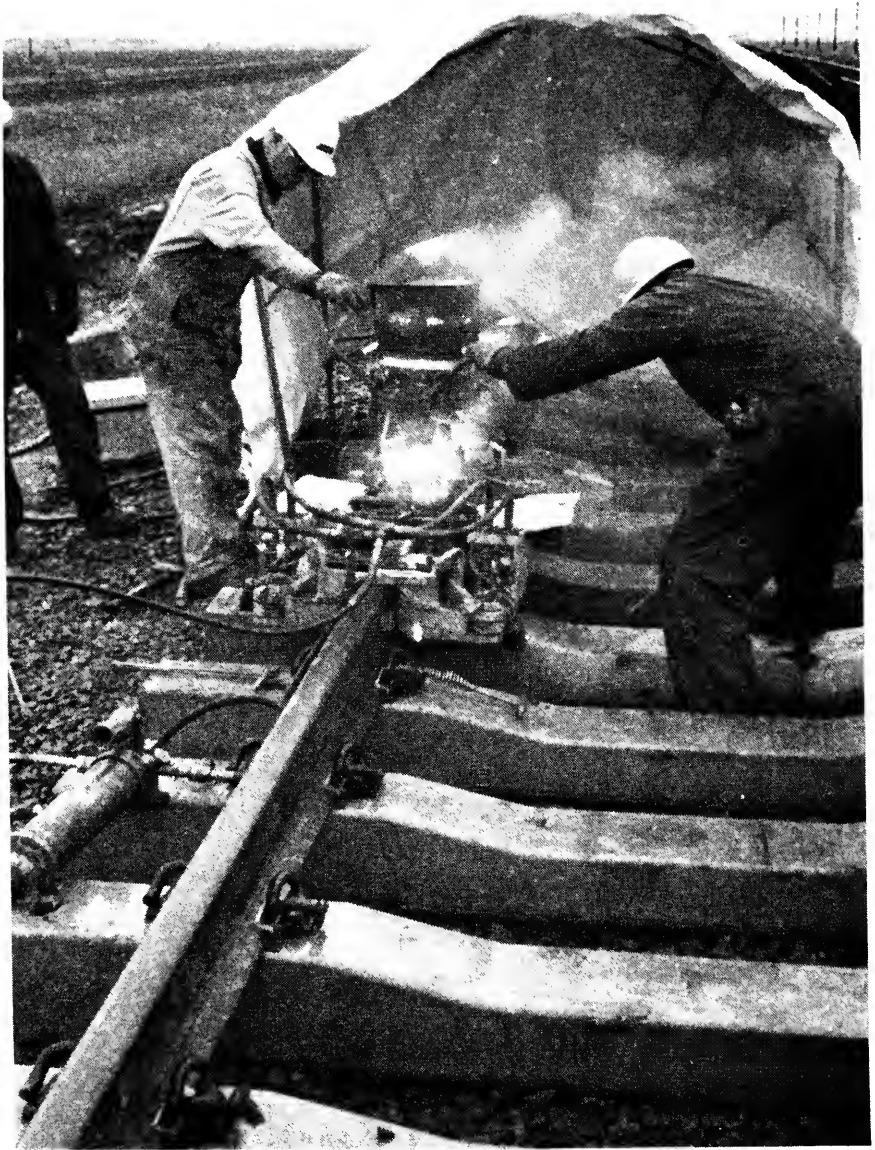
Fig. 4—Thermite welding on the CN.
