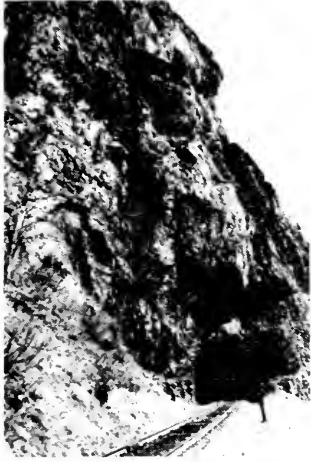
(a) Massive granite rock. Joints have random orientation. This slope can be cut vertically with controlled blasting.
