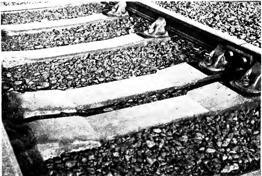
Photograph 2—Early "E1" type concrete sleepers for bull-head rail.
