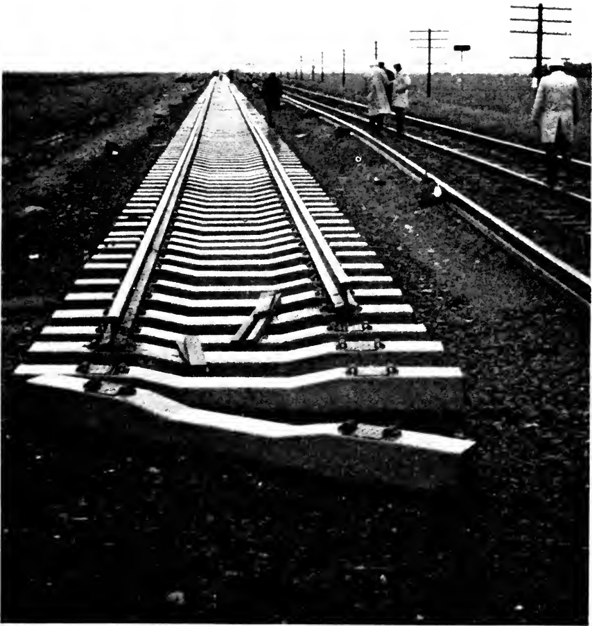
Fig. 3—Concrete ties and welded rail on the CN.
