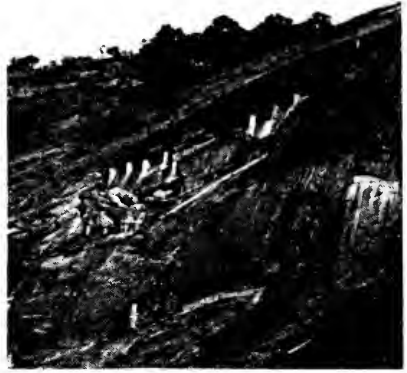
(b) Anchored reinforced concrete buttresses placed to support foliated granite rock high up on a slope.
