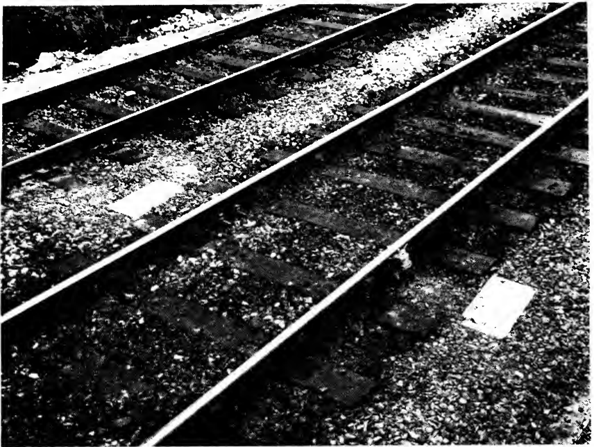
Photograph 1—(Foreground) BS 95-lb bull-head rail, softwood sleepers, cast-iron chairs, steel keys. (Background) BS 109-lb flat-bottom rail, softwood sleepers, base plates, Elastic Spikes.
