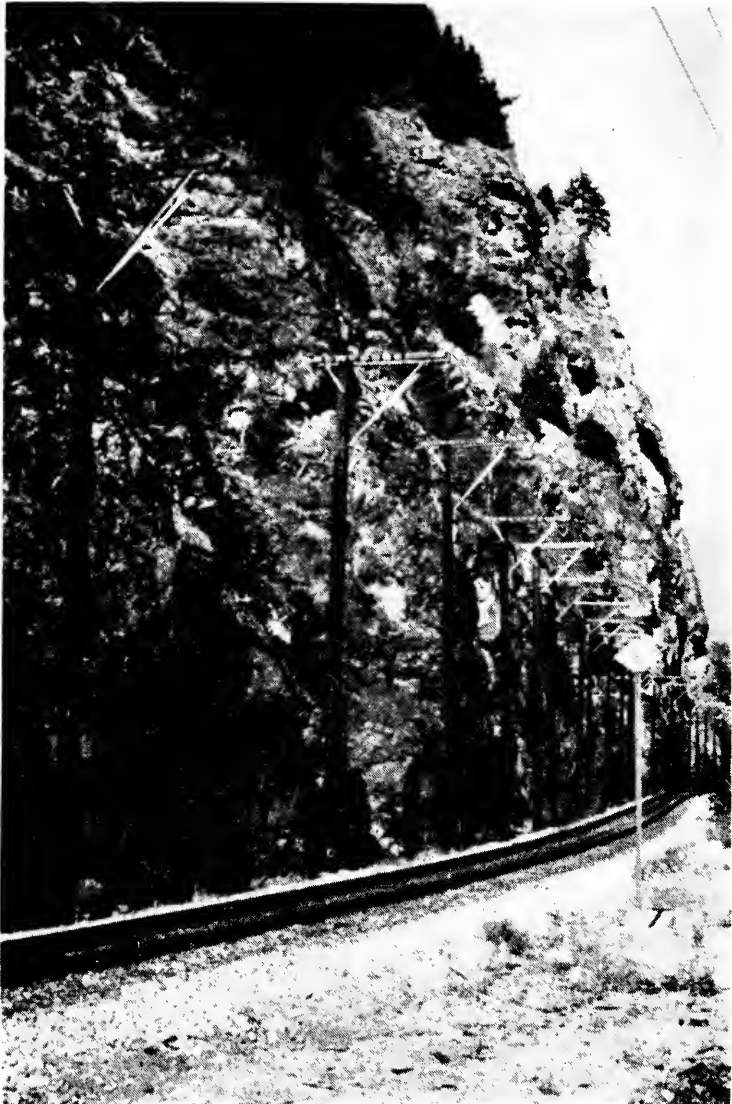
Figure 15—Electric warning fence below high, steep rock slope which is connected into track signal system.
