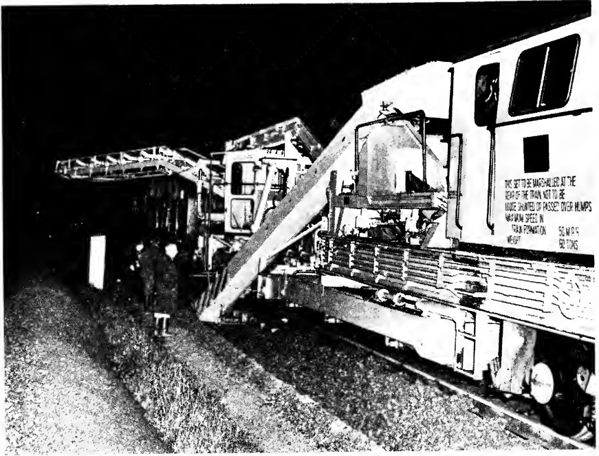
Photograph 6—Plasser ballast cleaner.
