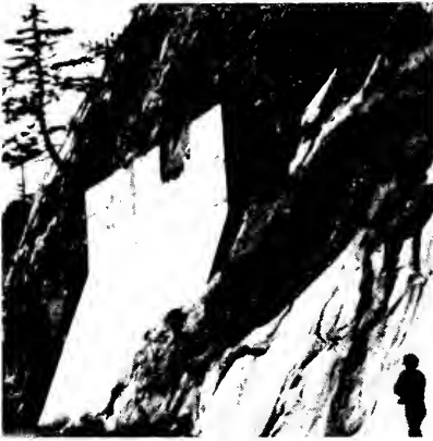
(a) Concrete buttress placed to support massive rock slab above the road bed.
