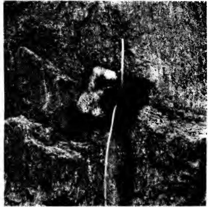
(d) Anchor bolt used to stabilize rock block. All bolts should be tensioned and grouted.
