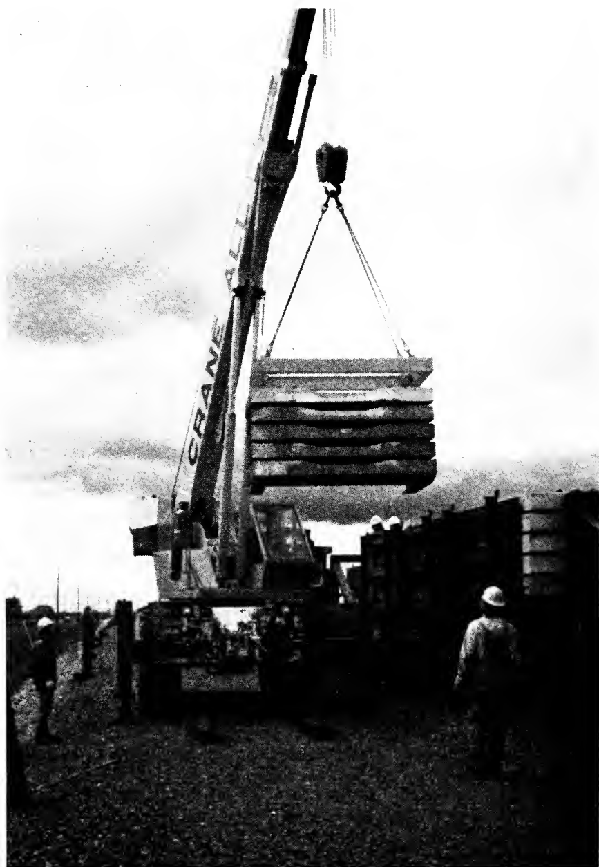
Fig. 6—Unloading concrete cross-ties onto the roadbed.
