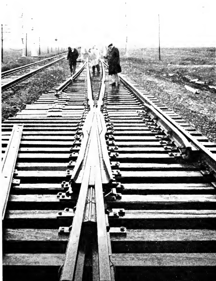
Fig. 5—No. 20 turnout under construction.
