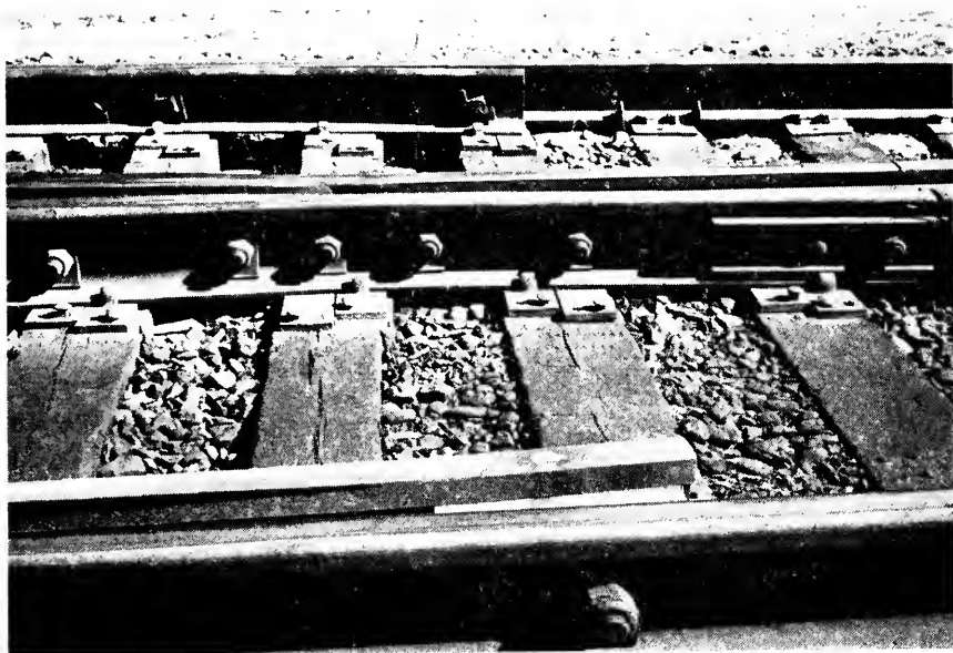
Fig. 10—Photo of toe end of guard rail.
