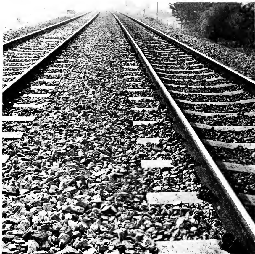
Photograph 3—Latest concrete sleepers, F27.
