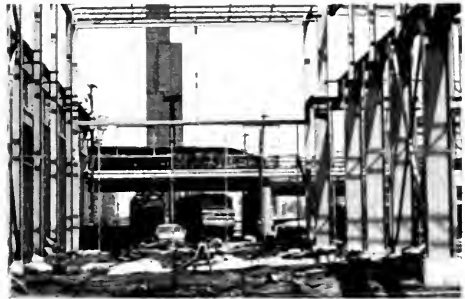
New Locomotive Service Shop Under Construction
