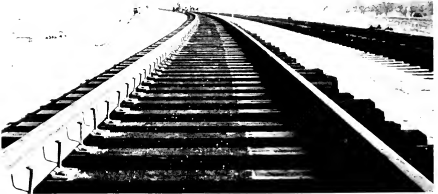
Figure 13.—Welded rail seated in the tie plates preparatory to being spiked when temperature reaches proper level.
