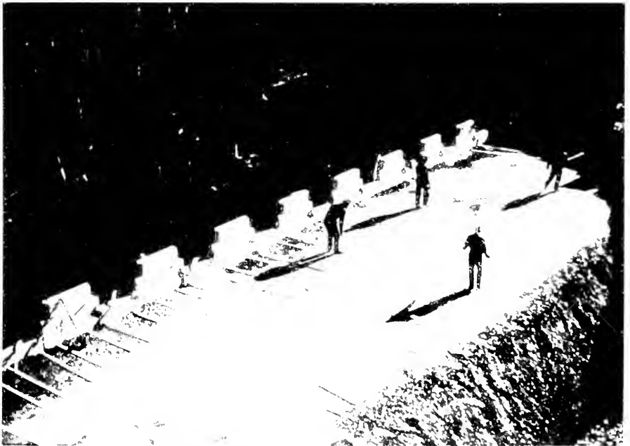
Figure 6. Placement of Reinforcing Strips
