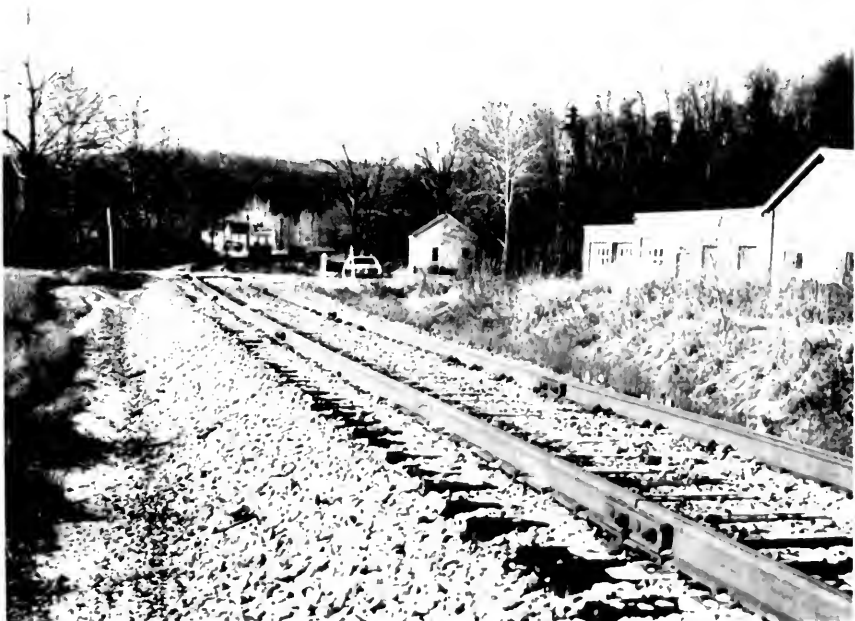
Figure 2—Route of Unit Train of 315,000 lb. cars using jointed relay 112 lb. rail over 30 years old (1980 photo).
