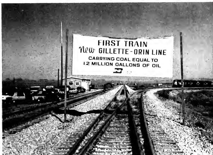
Figure 15.—First unit coal train moving on new line.
