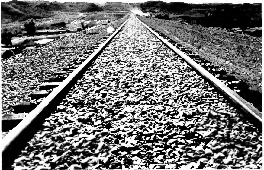
Figure 14.—Initial spread of ballast.
