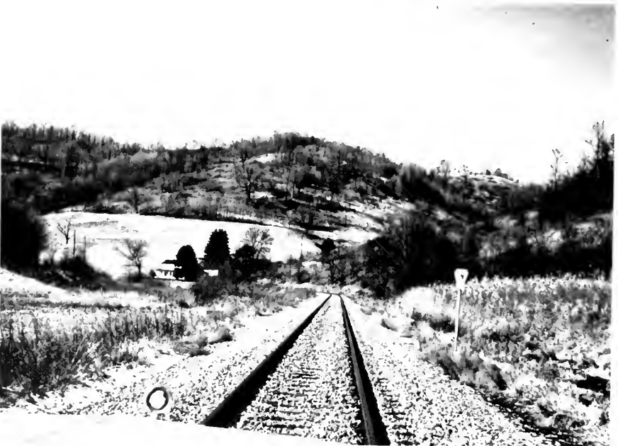
Figures 3 and 4—scenes on Route constructed south of Waynesburg, Pa. in 1968 for use of unit trains of 315,000 lb. cars (1980 photos).
