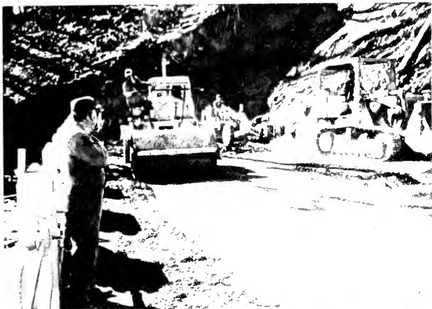
Figure 7. Compaction of Granular Backfill
