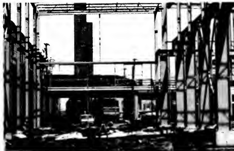
New Locomotive Service Shop Under Construction
