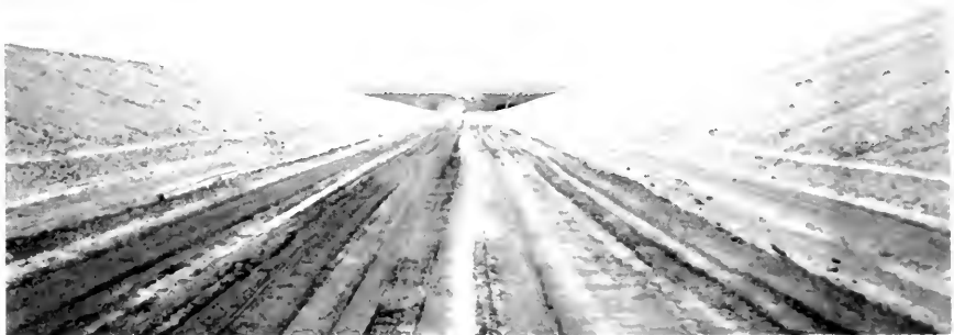
Figure 8.—Typical cut section with 3:1 slopes.
