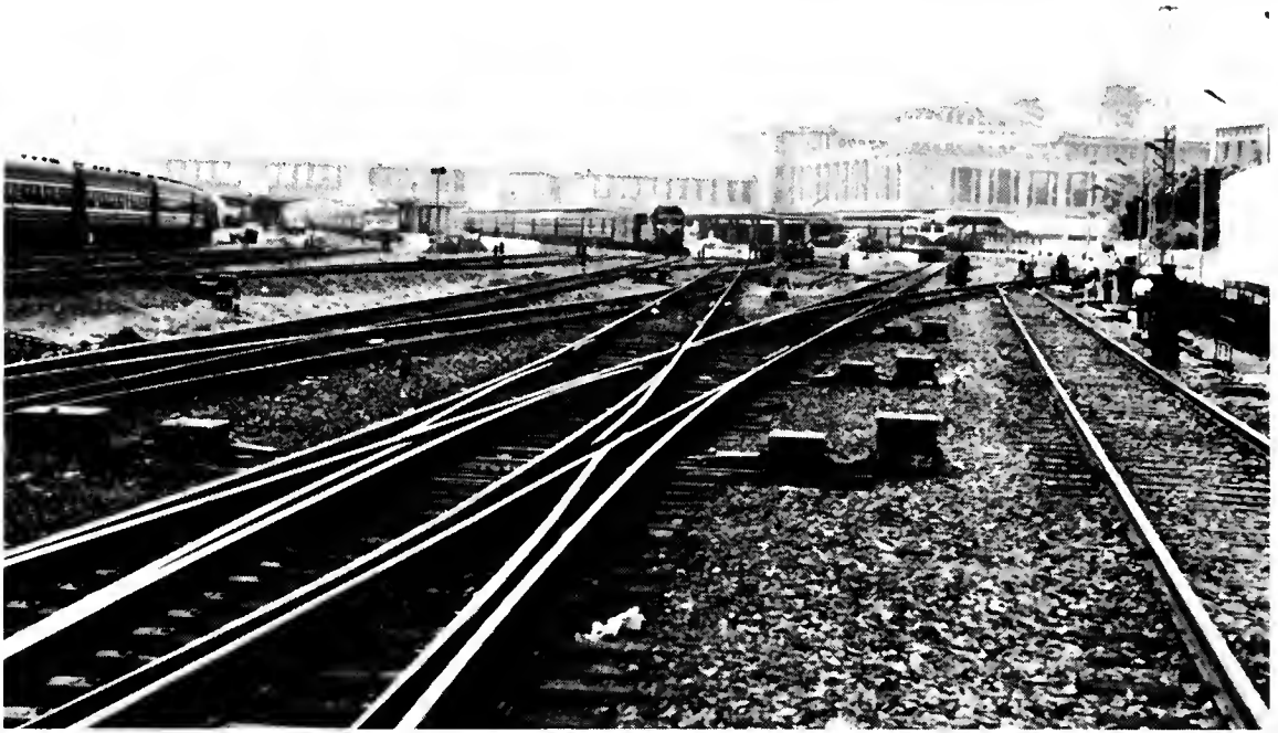
FIG. 3 Throat of main Beijing station which is stub-ended and completely dieselized.
