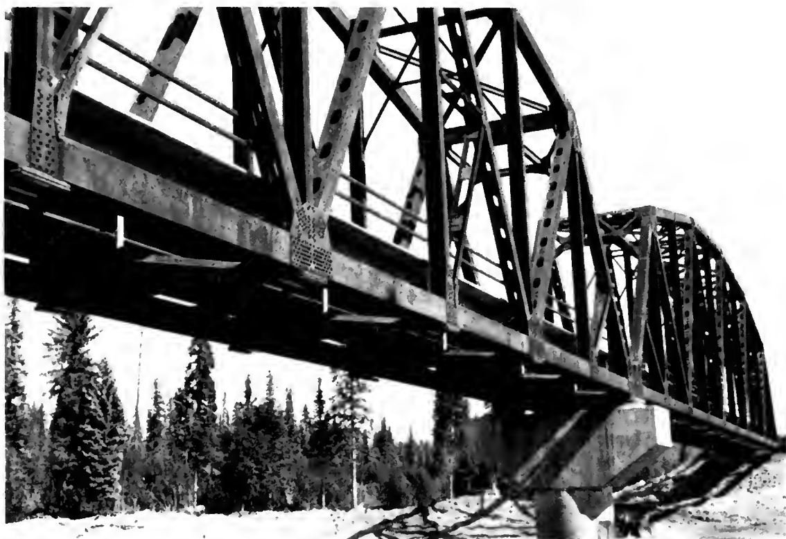
PLATE 1 -- Parsnip River Bridge
