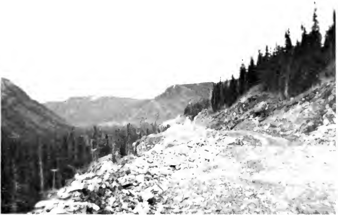
PHOTO. 3 View of grade under construction looking easterly towards the Table Tunnel.
