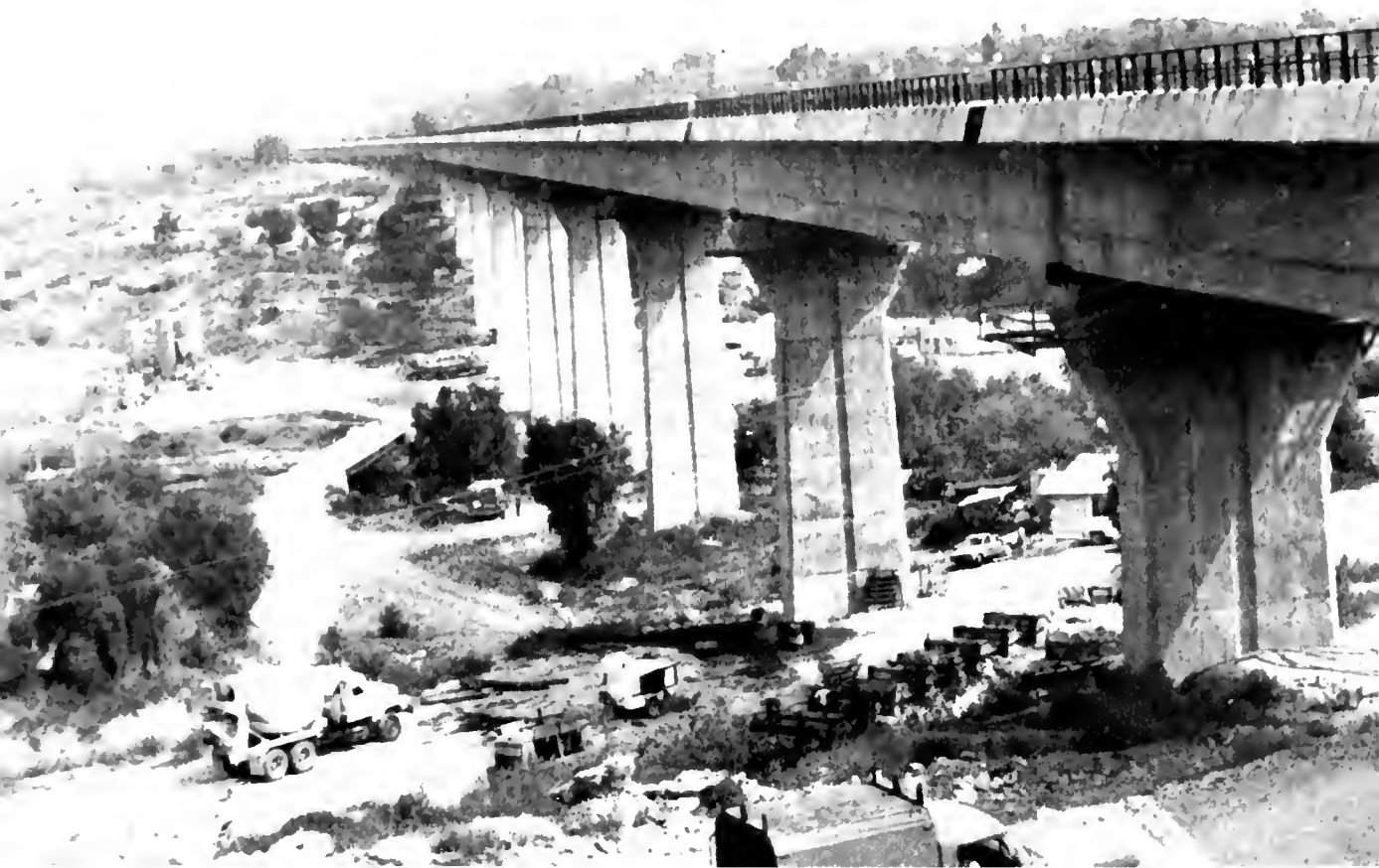
High bridge at Tula on high-speed Mexico City-Queretaro Line (note S - curve in background and archaeological ruins above and to right of second pillar).
