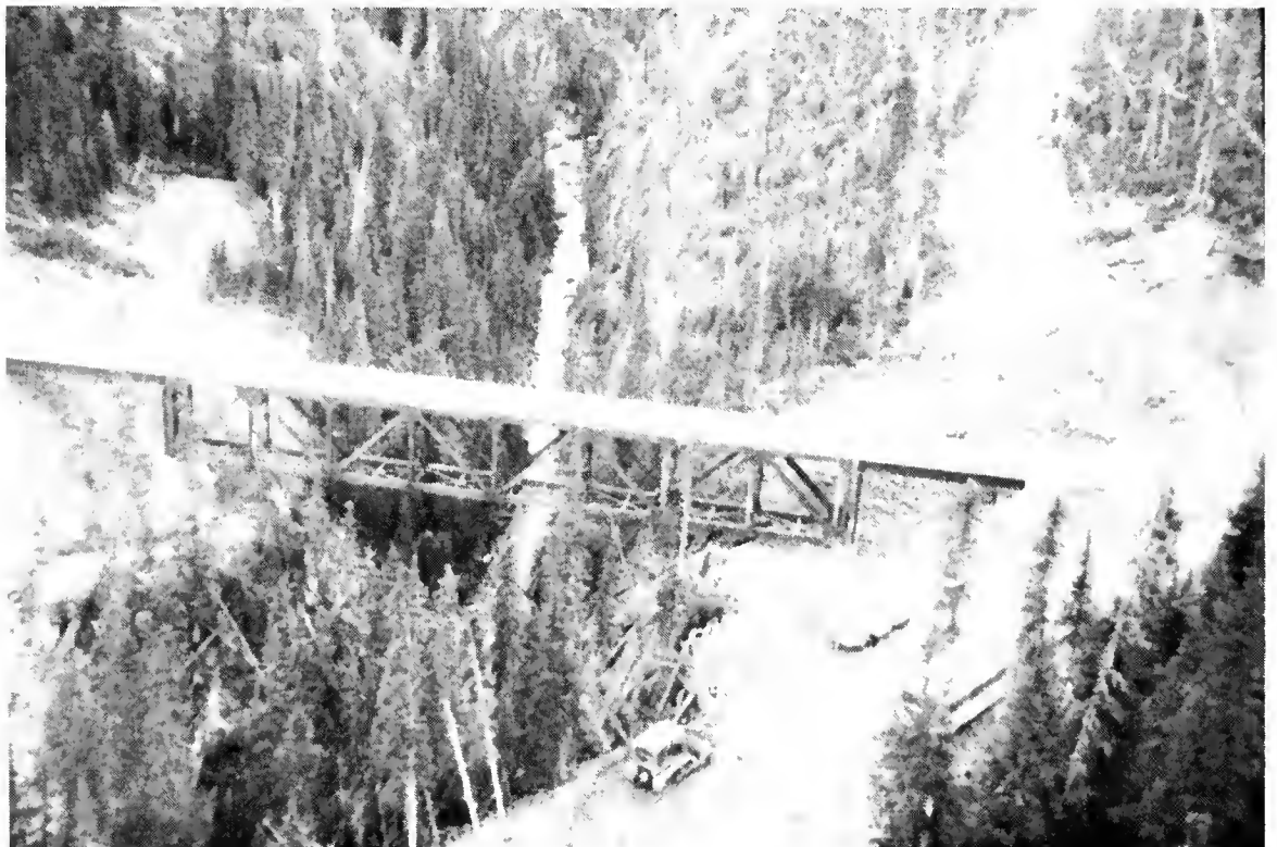
PHOTO. 10 Aerial view of completed Lost Creek Bridge at Km 80.
