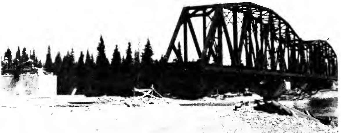
PHOTO. 9 The Parsnip River Bridge being launched (July, 1982).
