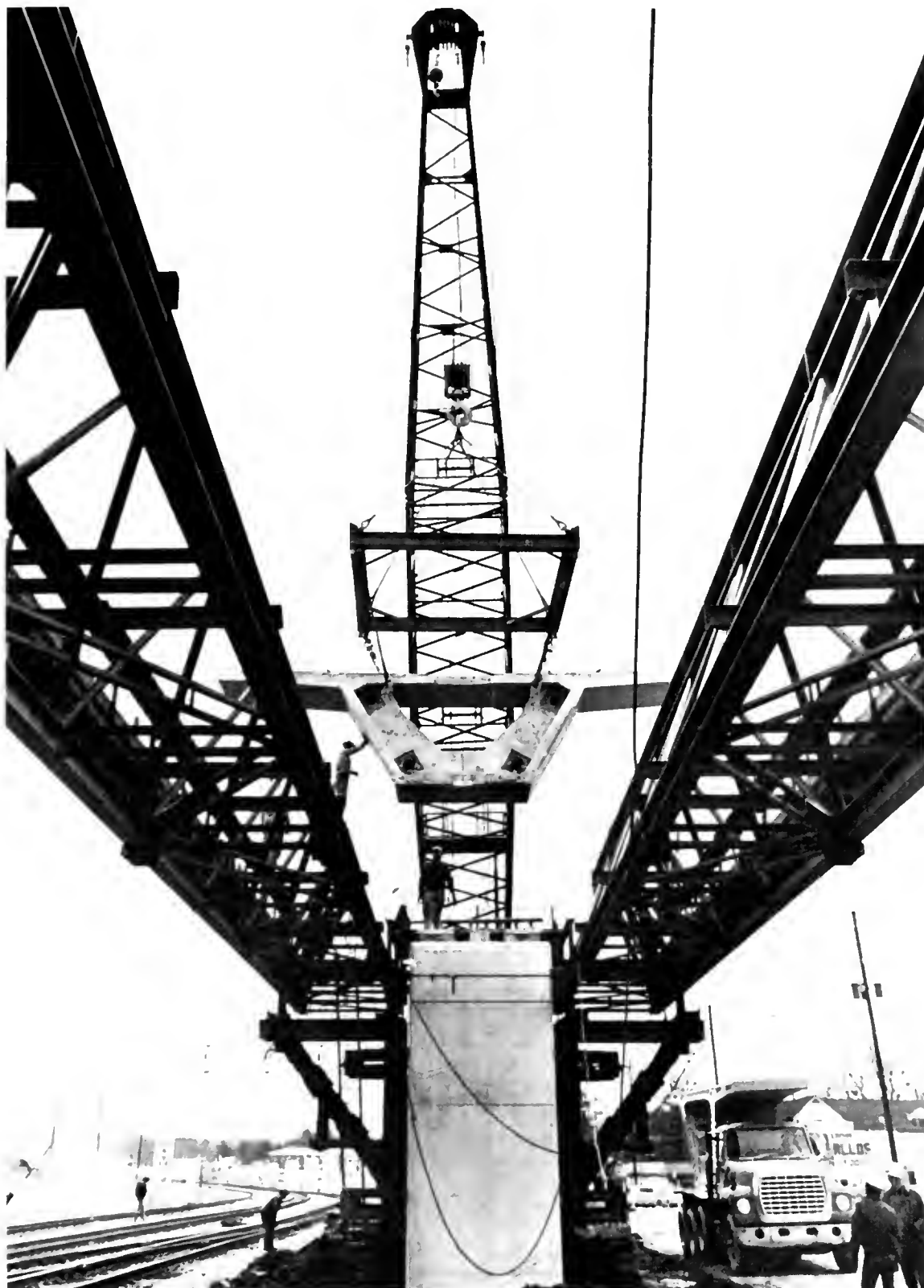
MARTA 360 RAPID TRANSIT PROJECT Atlanta, Georgia
