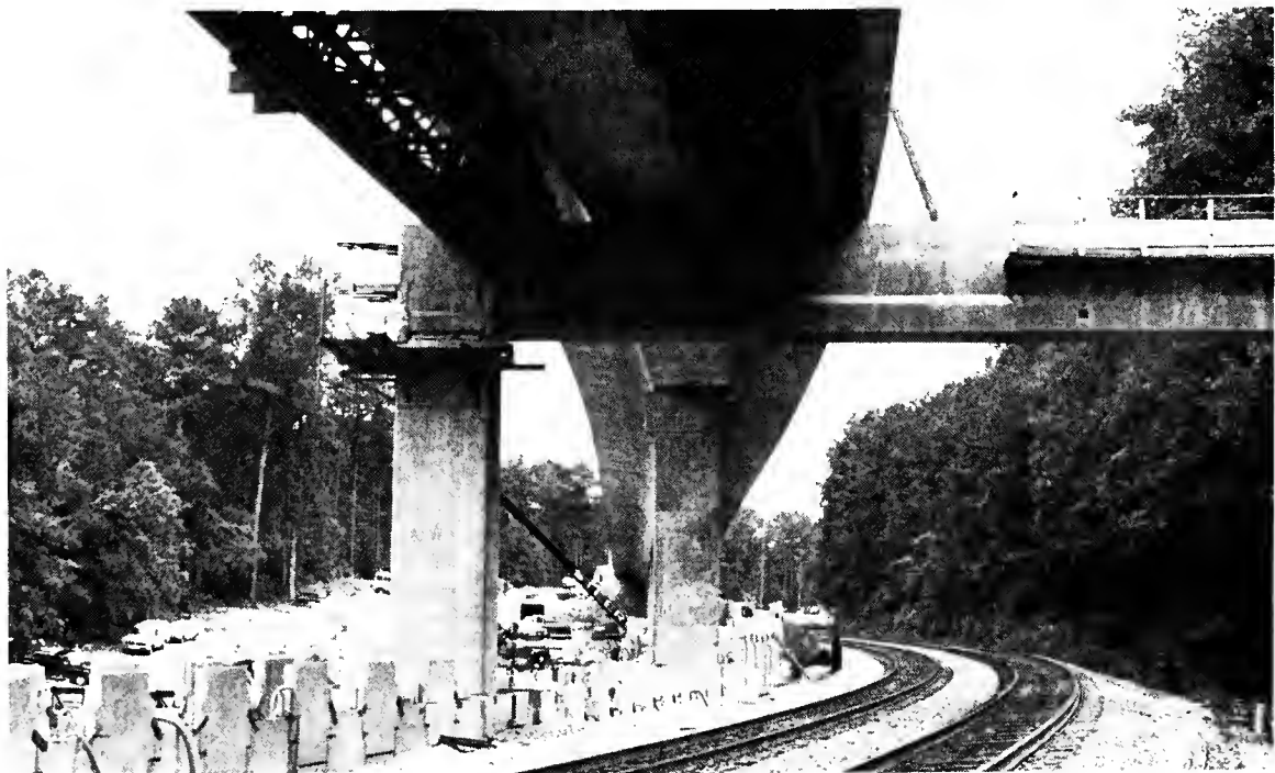
CN-480 MARTA RAPID TRANSIT PROJECT Atlanta, Georgia
