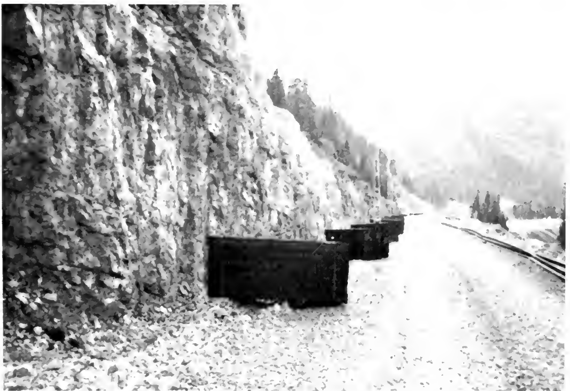
PHOTO. 4 View showing bundles of ties distributed along completed grade in the Table River Valley.
