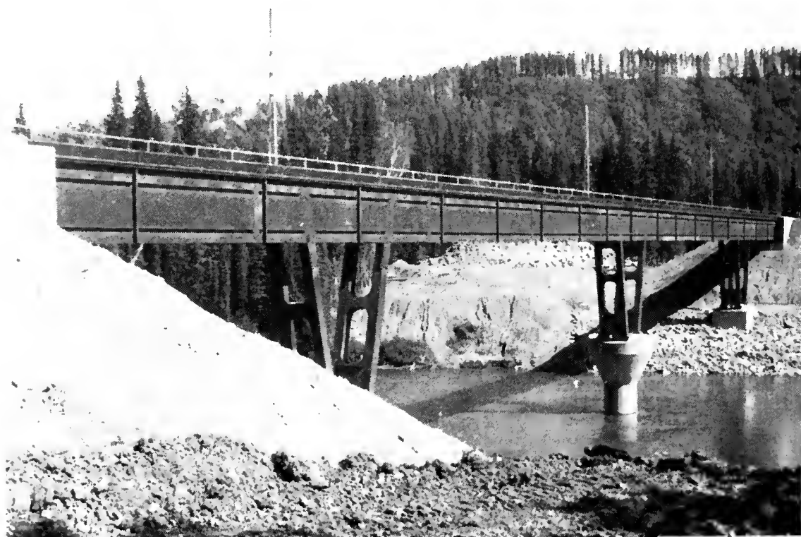
PLATE 2 — Murray River Bridge
