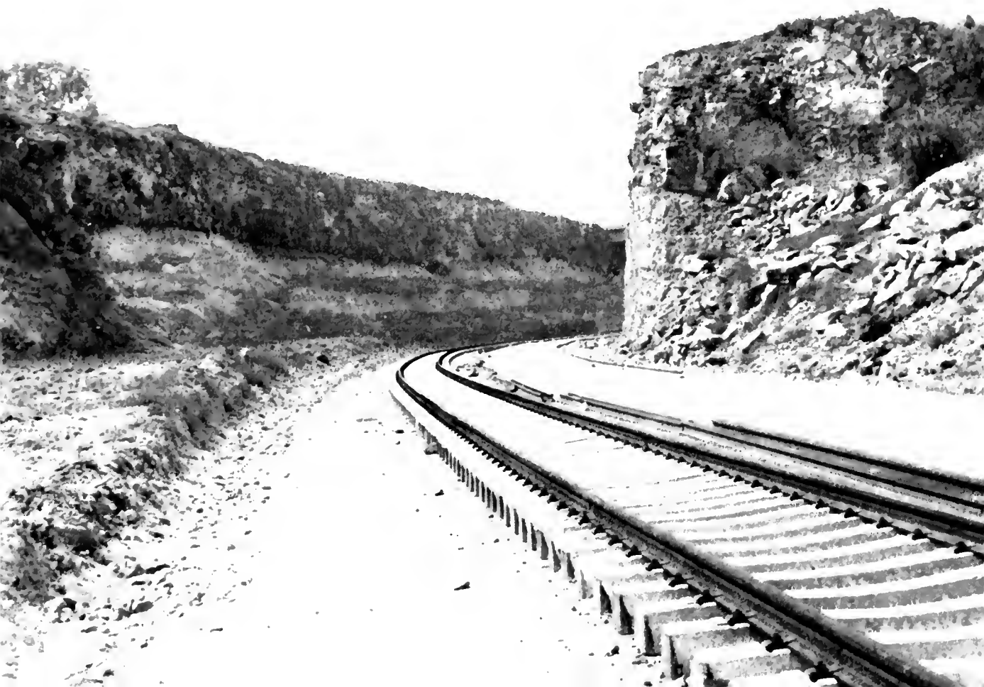
Cut just west of Tula high bridge with track under construction.
