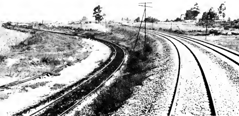
Old and new line as seen from rear of special train (two block ties, though no longer being purchased, were used in earlier construction on new line).
