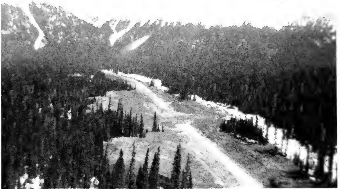
PHOTO. 5 Grade under construction in the Sukunka River Valley.
