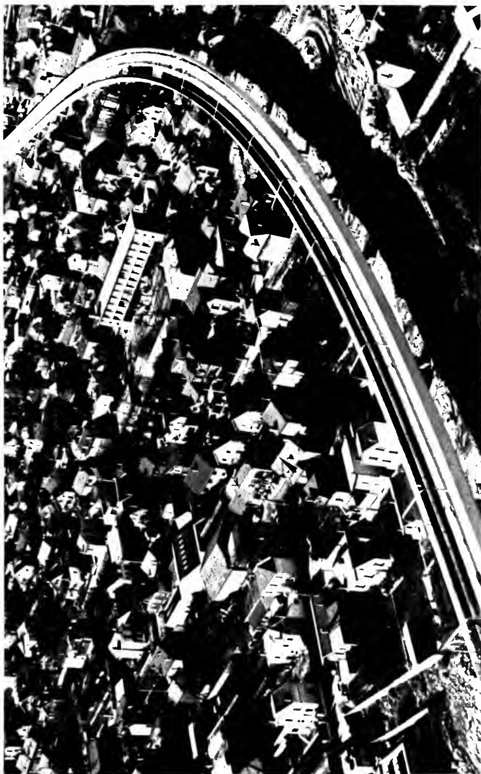
Marne la Vallée Viaduct, France
