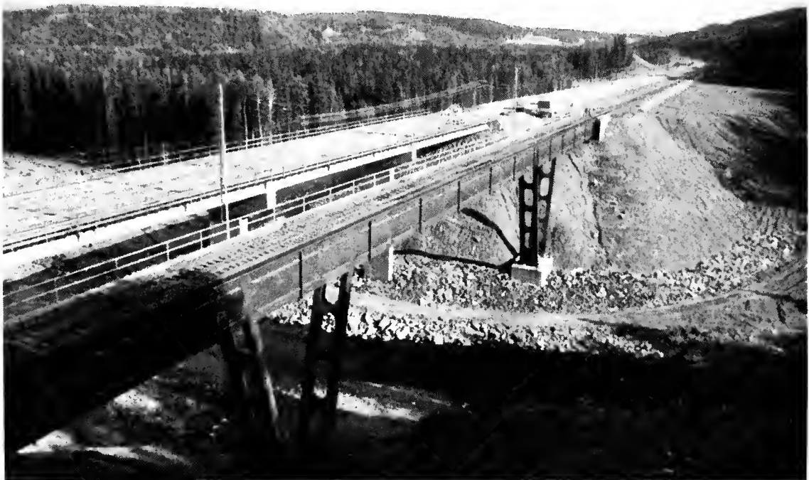
PLATE 3 — Wolverine River Bridge
