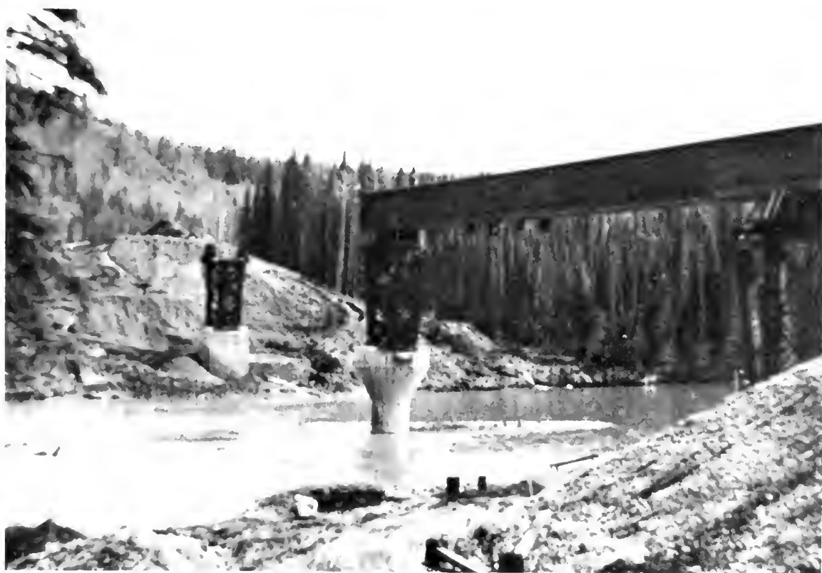
PHOTO. 12 View showing Murray River Bridge being launched into place.
