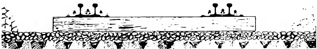
New panel in position—ready for ballast work.
