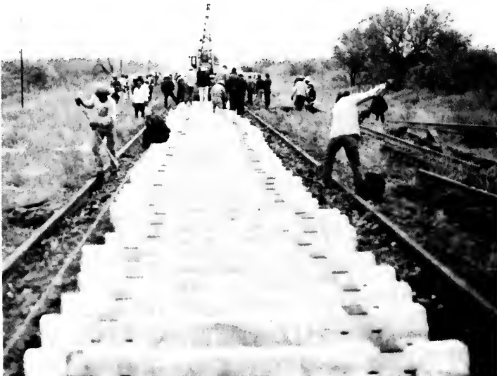
Installation of Concrete Ties
