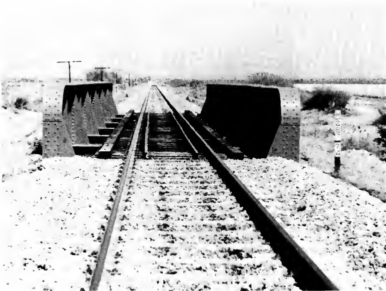
New bridge on N de M for 263,000 lb traffic
