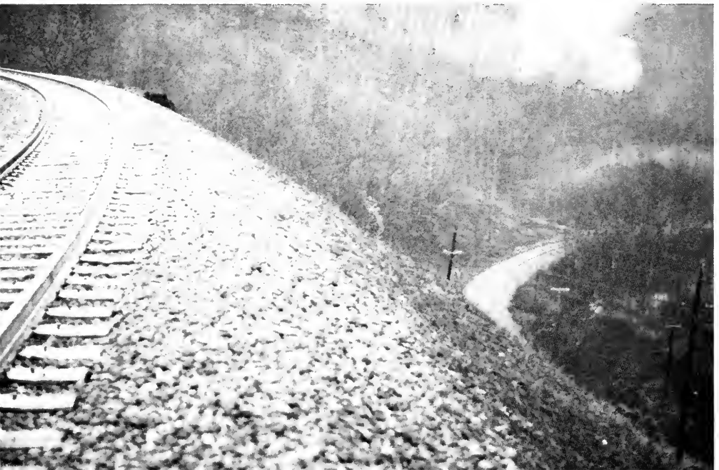
Figure 6 - Two levels and locations of track show in this photo. In the foreground is about milepost 116.8. Approximately 150 ft. below on the right is about milepost 115.5. The tracks get within about 200 ft. of each other measured horizontally near this point on the Salisbury-Asheville line.
