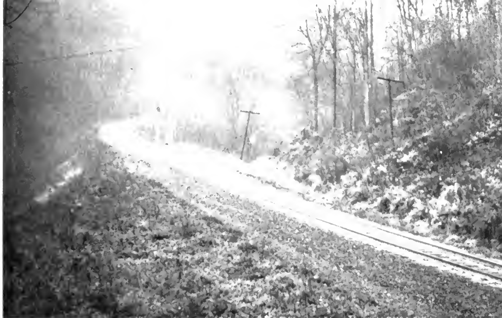
Figure 4 - 4.7% ! This photo looks upgrade at about the center of the 2.6 mile long 4.7% grade on the Asheville-Spartanburg line near Saluda, North Carolina.
