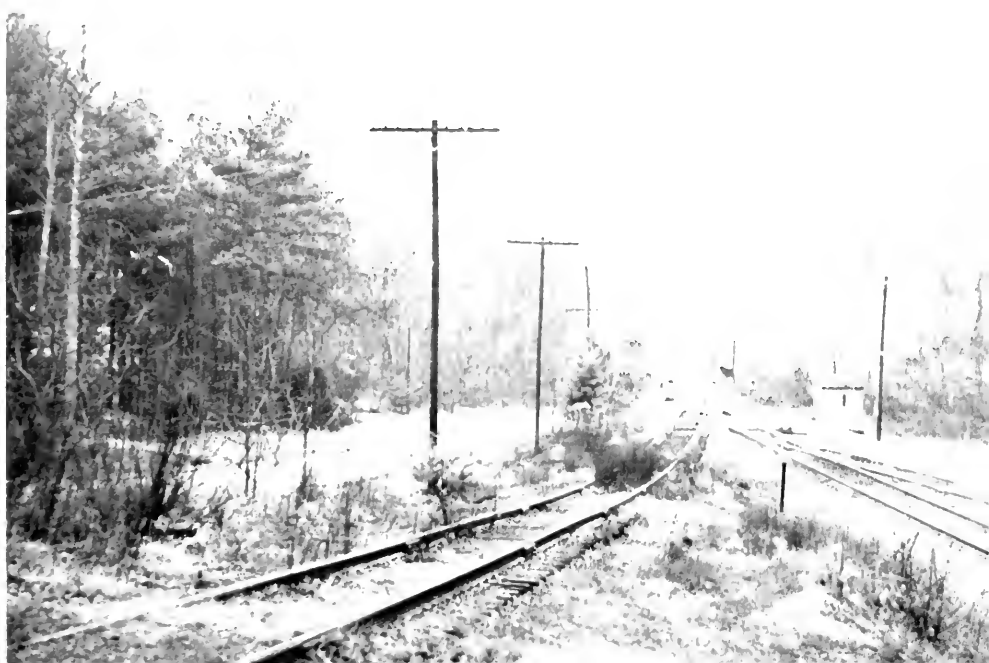
Figure 5 - Shown here is the obviously seldom used runaway track at the bottom of the 4.7% grade from Saluda.
