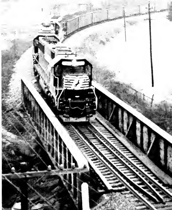
Figure 8 - Norfolk Southern Unit Coal Train at bottom of 2.2% grade on the Asheville-Salisbury line during rainstorm.
