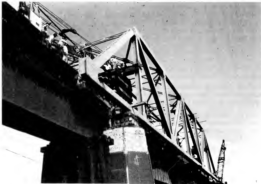
Replacement span installed
