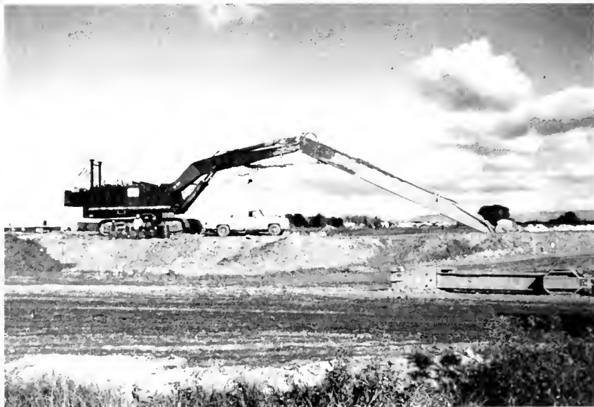
Backhoe with 70 ft. boom for cut-off wall excavation.
