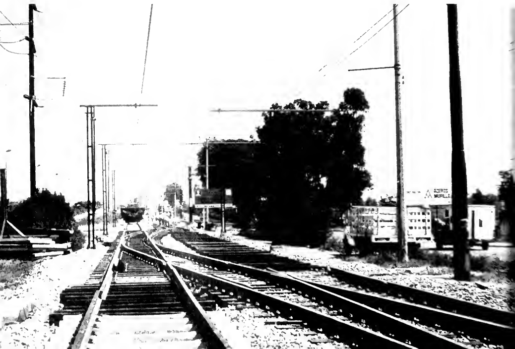
Photo below shows construction in progress near south end of new light rail line in Guadalajara—meeting attendees visited this location on Saturday.
