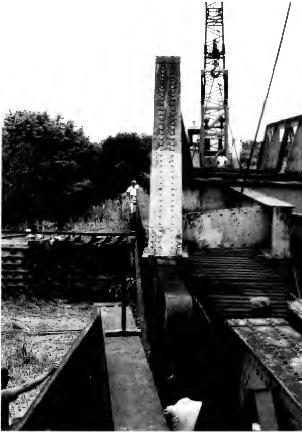
Thru girder span is jacked into position from false settings.
