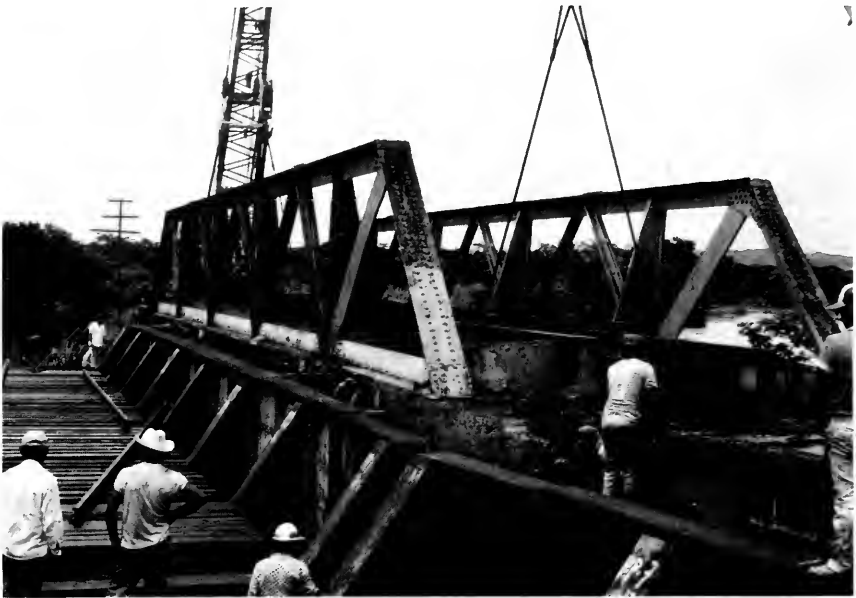
Old truss span is lifted for sliding of new thru girder span.
