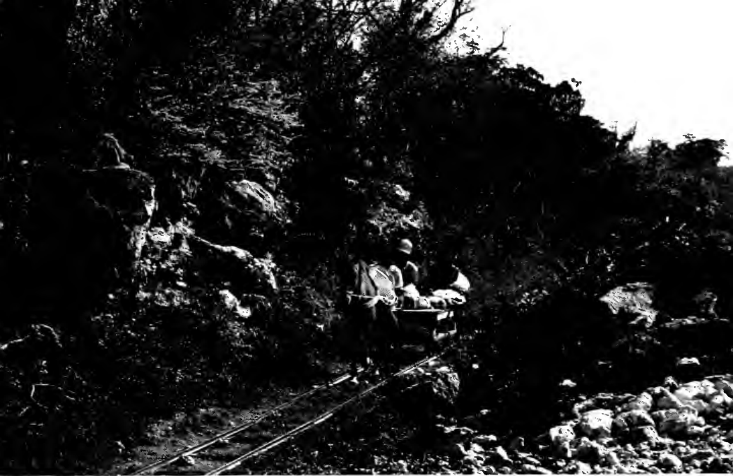
Photo 2—Family on horse car heads through rock cut between Homun and Cuzama, Yucatan—photo at right below shows fill between rock retaining walls at Tixkokob, Yucatan.
