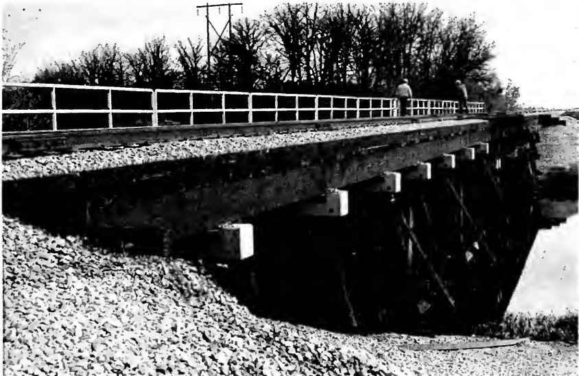
Photo 4. Installed longitudinal stress laminated railroad bridge.
