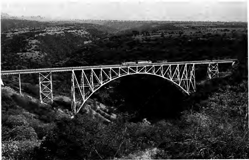
Rehabilitated and strengthened Marques bridge.
