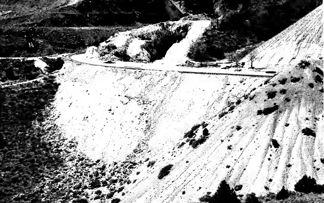
Photo 2: New 75-foot fill on tunnel by-pass.
