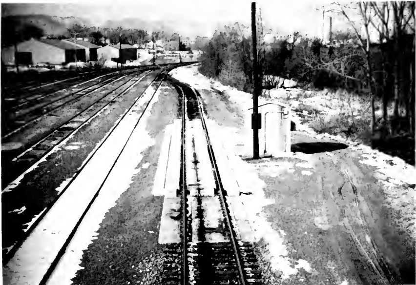
Figure 1. Uncoupled in-motion scale in Winona, Minnesota.
