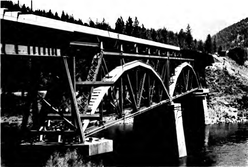
Figure 1. Completed arch system reinforcement in place on deck truss spans.
