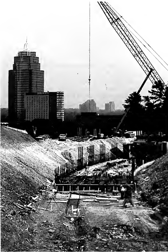
Construction in the Georgia 400 corridor.
