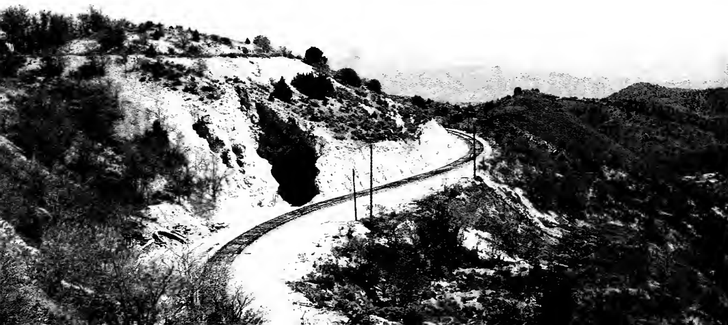
Photo 3: End of by-pass at Gold Hill end of tunnel.
