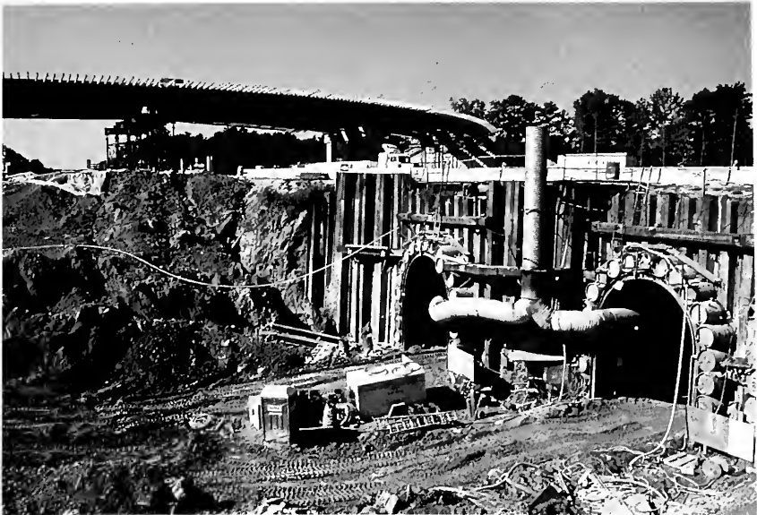
East end of tunnels under and car bridge over I-285.
