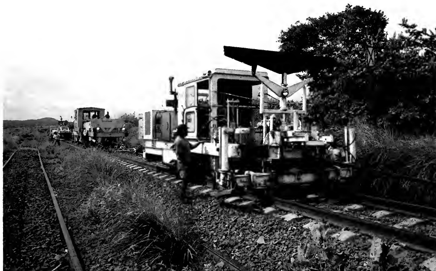
Surfacing work in progress on rehabilitated line.
