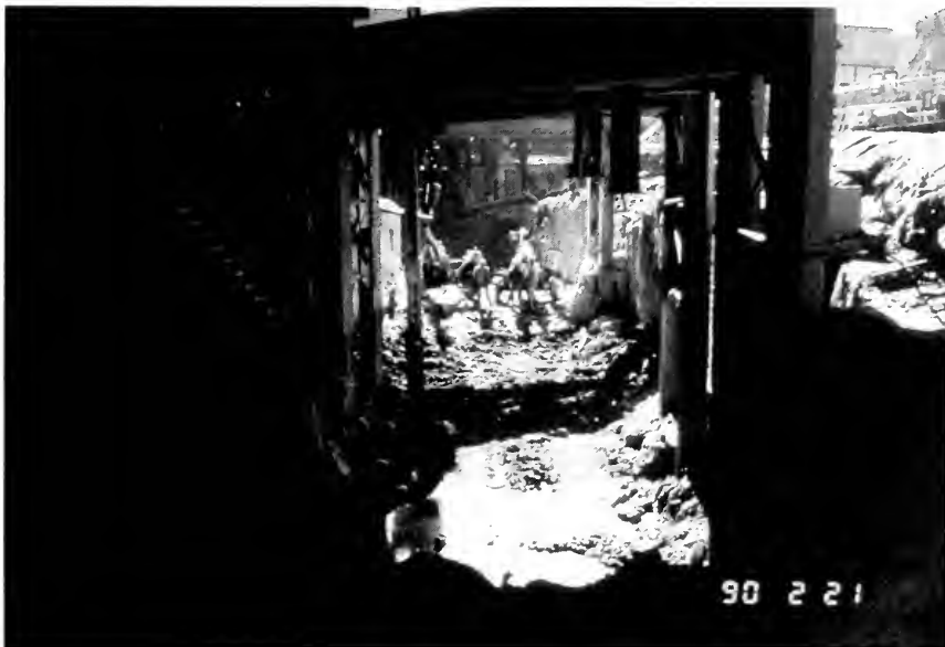
Photo 6. Inverted U-shapes near tunnel entrance for overhead structure support.
