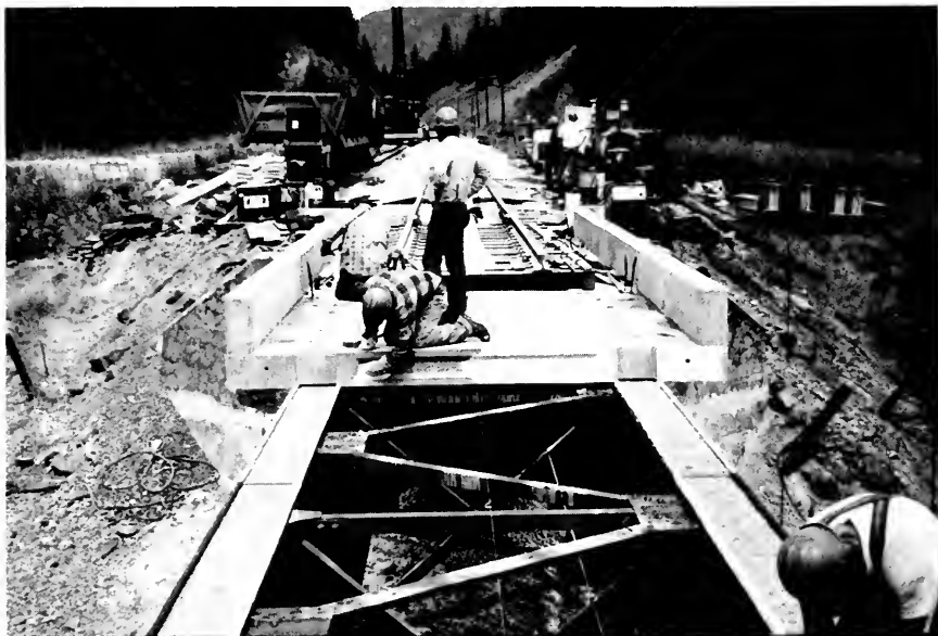
Figure 2. Precast ballast box installation on deck plate girder span.
