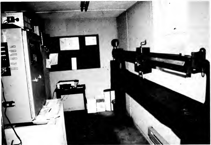
Figure 3. Remote weighing electronics in Roseport, Minnesota scale house.
