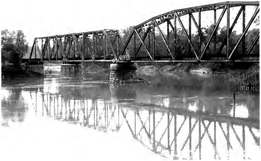
Figure No. 7 – Swing Span Prior to 1992 Flood
