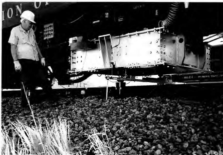
Exhibit 7. TLV Rail Uplift Ground Reference Frame and LVDTs.
