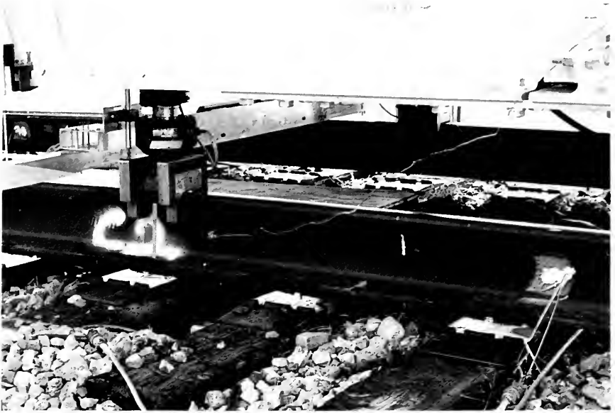
Exhibit 16. Rail Being Lifted.
