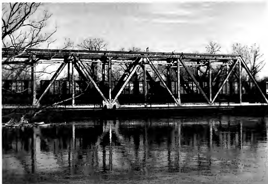
Figure No. 9 – Loaded Test Train for Checking Deflection of Strengthened Span
