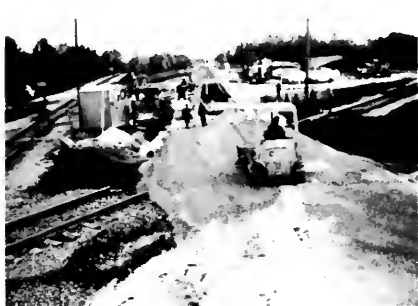
Figure 17. Cutover at Iles Junction.
