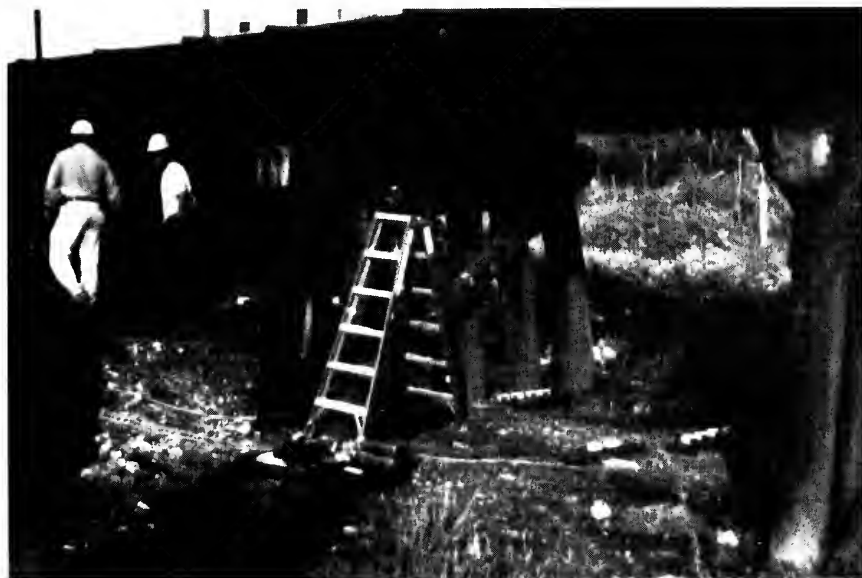
Figure 2. Instrumental SPRR Timber Bridge at Cline, Texas.
