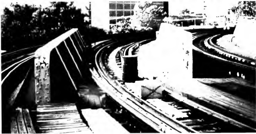
Reconstruction of the Green Line proceeds at various locations.
