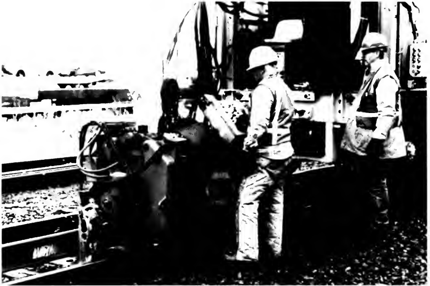
Figure 5. Mobile Holland welder in operation.
