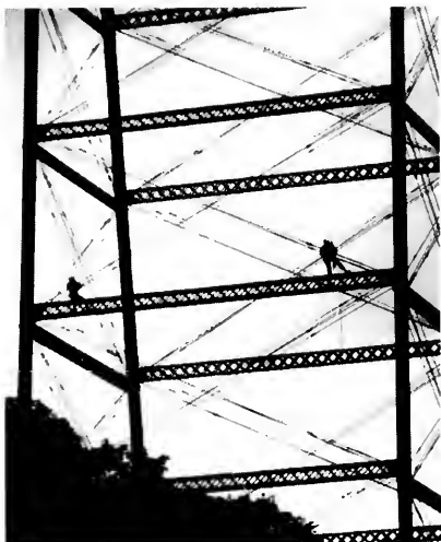
Figure 1. On high steel. Inspectors take on the role of a real life “Spider Man.”
