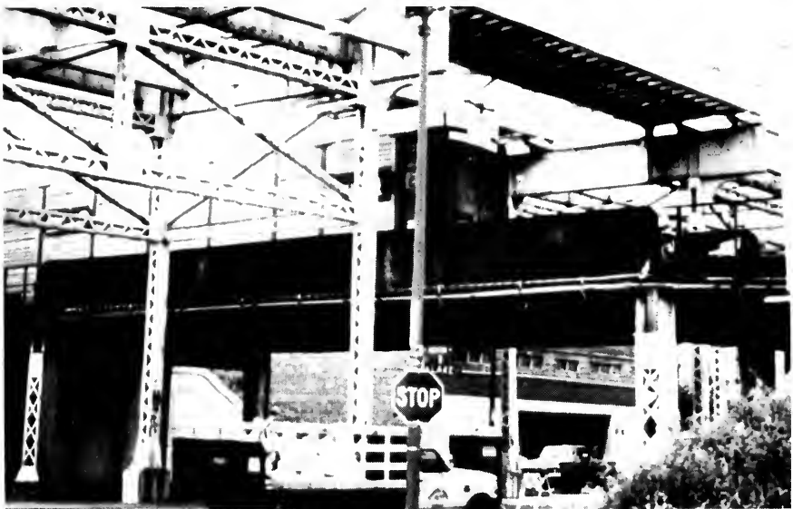
Reconstruction of the Green Line proceeds at various locations.
