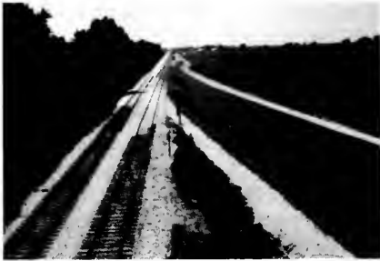
Figure 15. New Track Merges with Existing in Joint Use Corridor.
