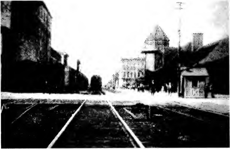
Figure 3. Railroad Service to Downtown Springfield.
