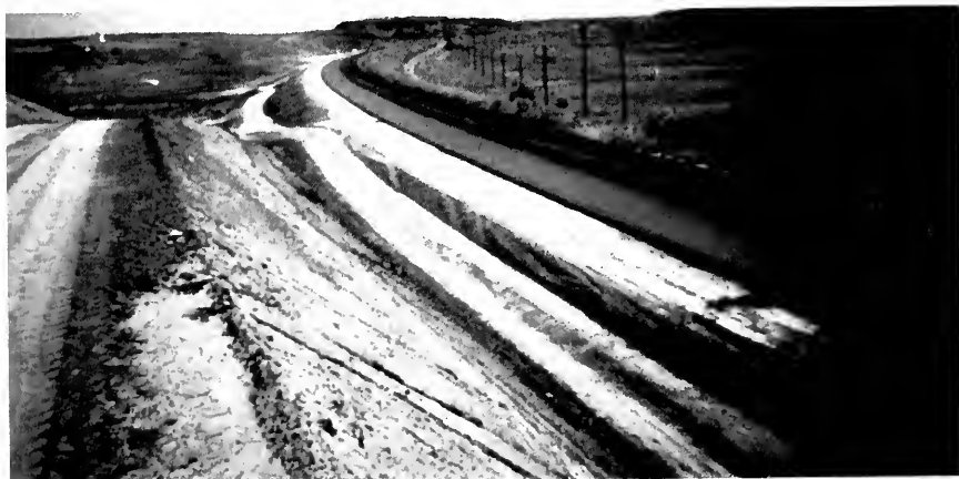
Figure 25. Long Asphalt Road
