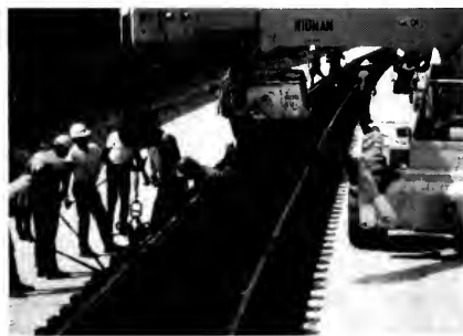
Figure 13. Skeleton Track Construction.
