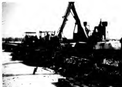
Figure 14. Southern Pacific Tie & Rail Replacement.
