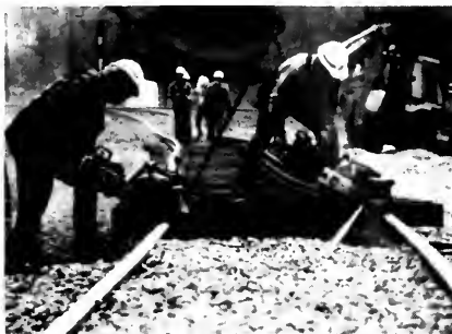
Figure 18. Placing Track Panels at Iles Junction.
