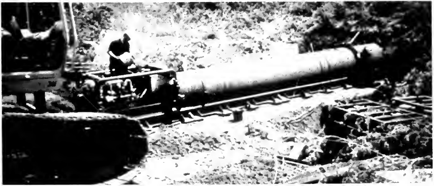
Figure 22. Pipe Bore
