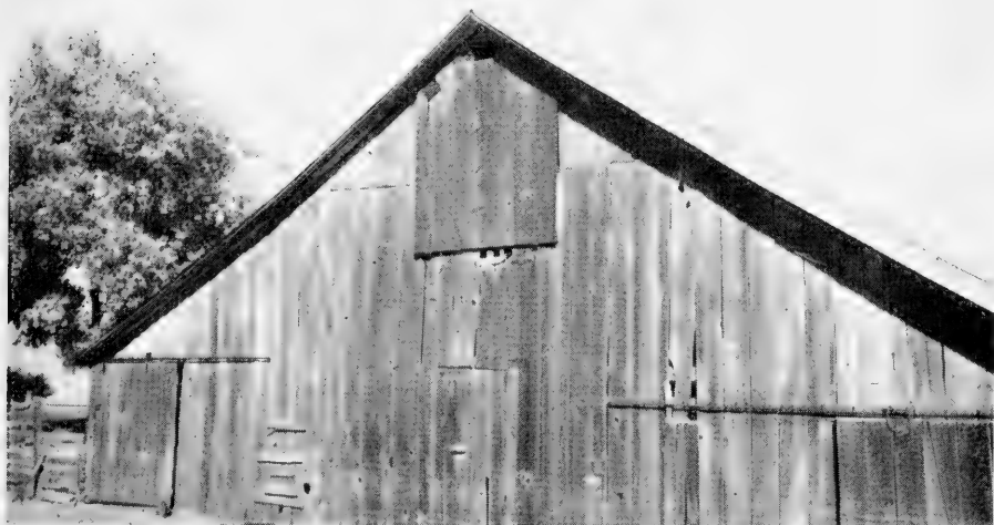
Figure 7. Pallid bats inhabiting this barn, 4\frac{1}{2} miles northeast of Shandon, San Luis Obispo County, California, were observed entering and leaving through the opening seen immediately below the peak of the roof. Photographed October 22, 1949.
