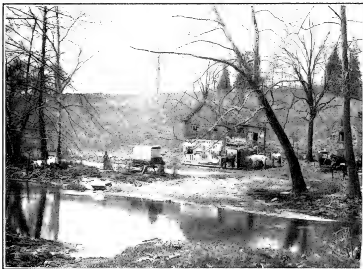
View across Creek below Bridge (from Northeast)
