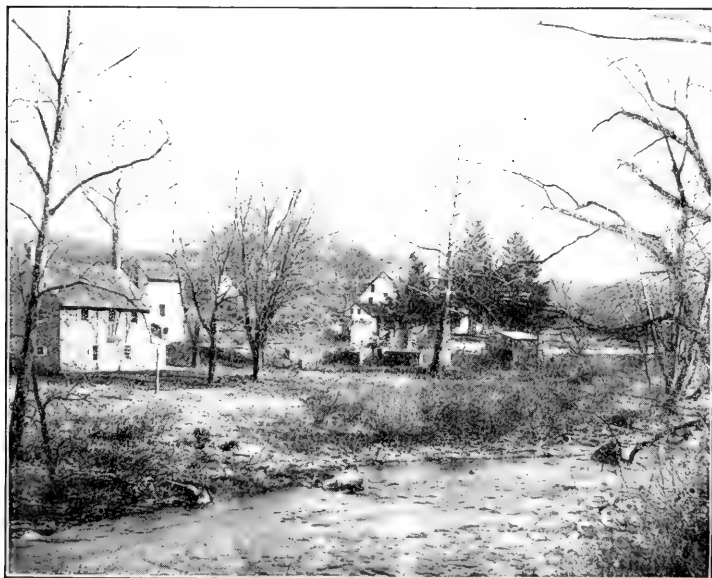
Former Blacksmith and Wheelwright Shop, Library, Ruins and Farm House (from West)
