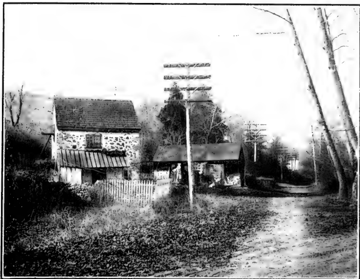
View on Southwest side of Creek near Bridge (from Southeast)
