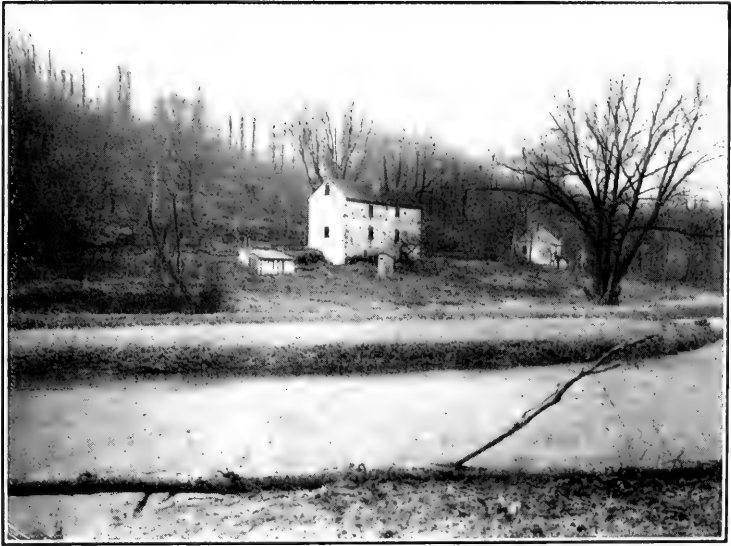
View across Dam (from Northeast)
