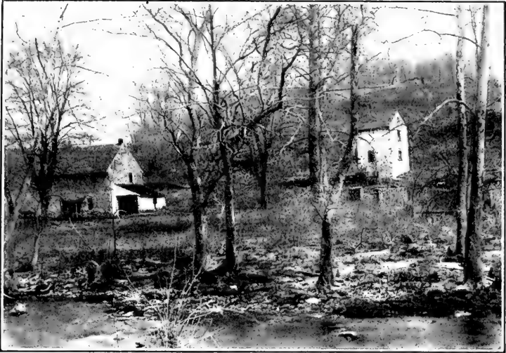
Former Blacksmith Shop and Library (from South)
