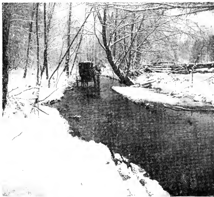
Many gravelly and rock bottom streams are used as public roads. This view in southern Martin County.
