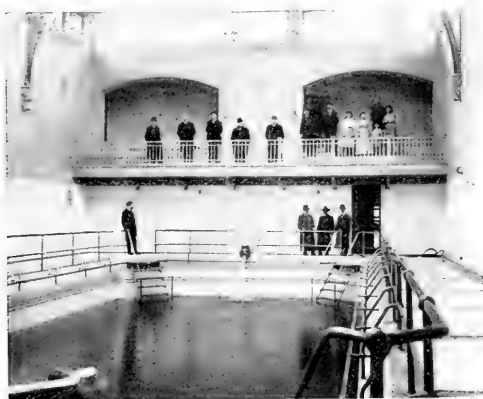
Fig. 5. Plunge, East 23d St. Public Bath, New York City. (A fairly well lighted indoor pool.) By courtesy of "Modern Sanitation."
