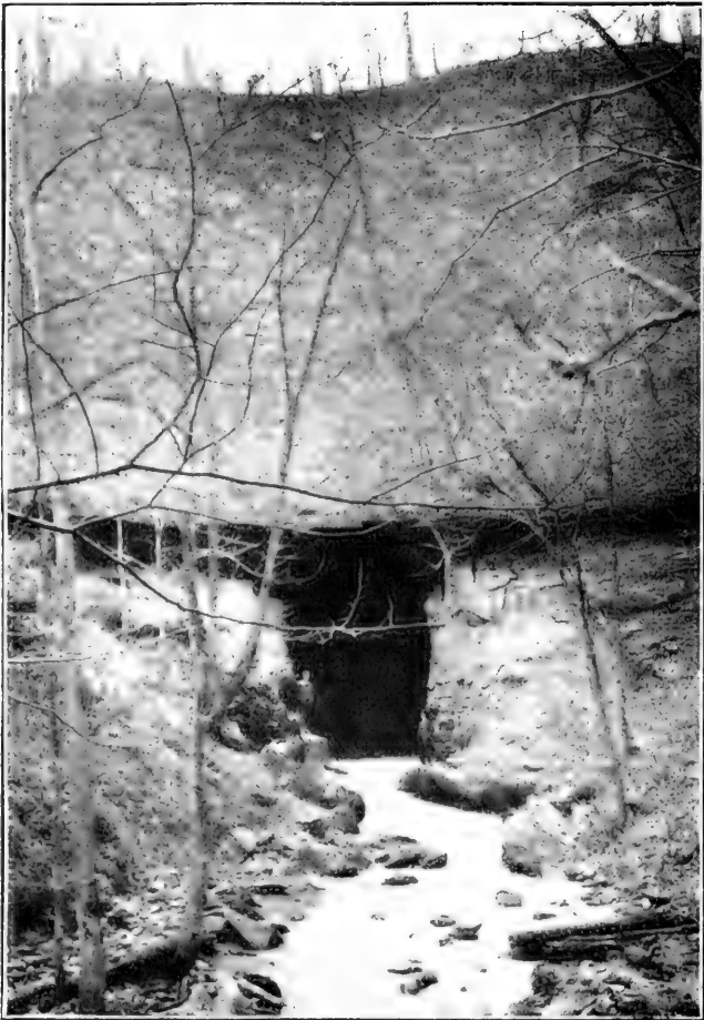
Fig. 11. Emergence of cave stream, mouth of Shawnee cave east of Mitchell, Indiana. The roof of the cave at its mouth is well supported. Just back of this there are two large rooms connecting with the main cave, leaving a large area of roof unsupported. It has faulted down about six inches. The completion of this collapse might, in time, leave a natural bridge at the present mouth of the cave. The valley is a typical collapse valley.
