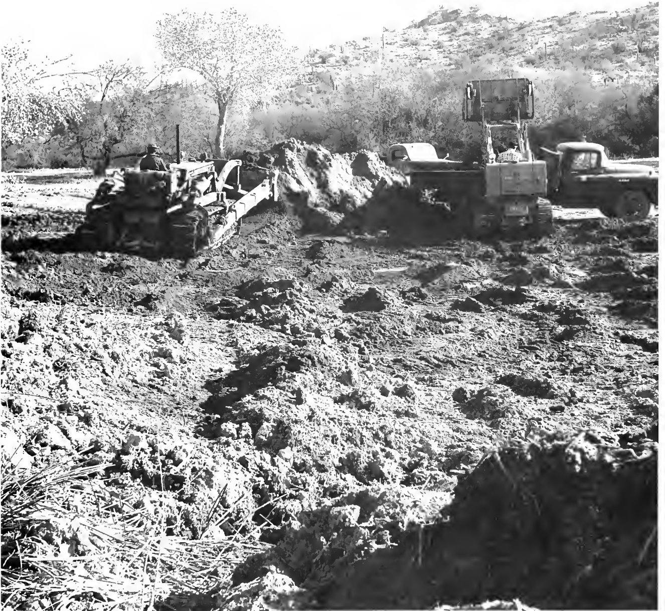
Figure 9 Quitobaquito, looking northeast, while the pond was being deepened. Photo by Warren F. Steenbergh, January 1962, courtesy Organ Pipe Cactus National Monument (photo file W-34C)
