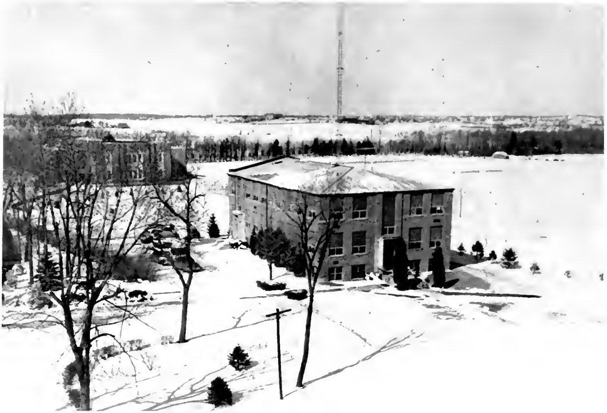
VIEW OF THE NORTHWEST — SCIENCE BUILDING AND GYMNASIUM
