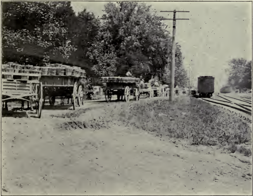
THE OTHER END OF THE LINE—WHERE CARS ARE LOADED FOR SHIPPING
